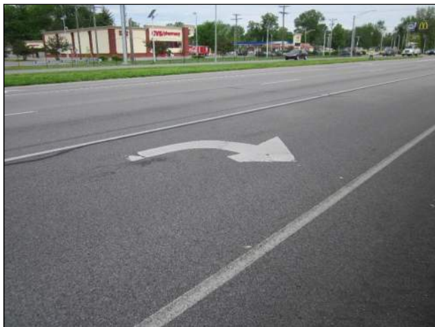
Pavement Markings in Northbound Right-Turn Lane
