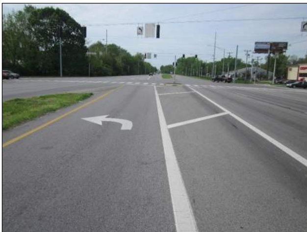
Pavement Markings in Southbound Left-Turn Lane
