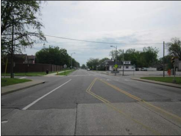
Washington Ave Looking East, East of US 41
