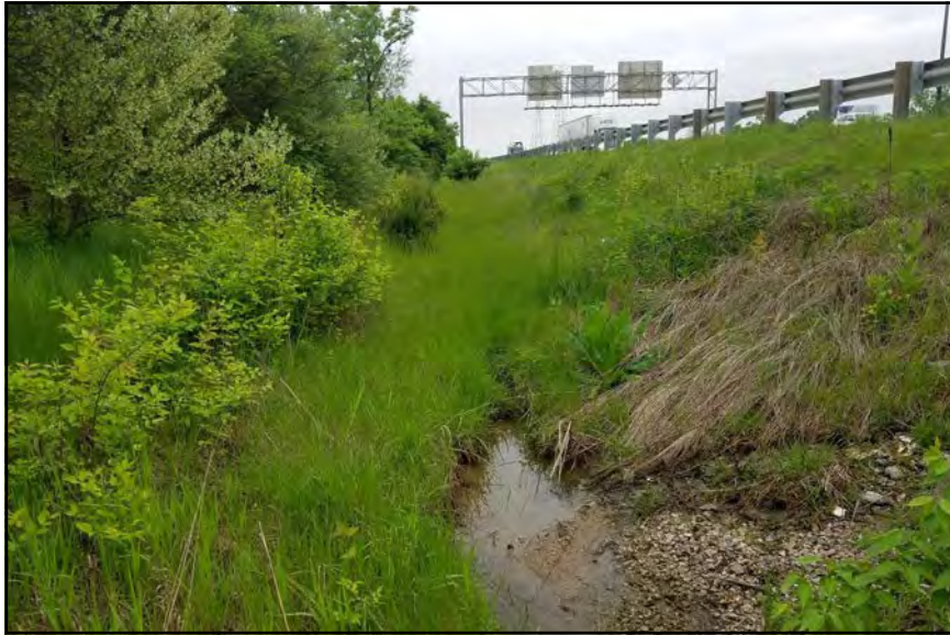
Photo 25, I-465 On Ramp, Facing Northwest, Located at the end of Ditch 1.
