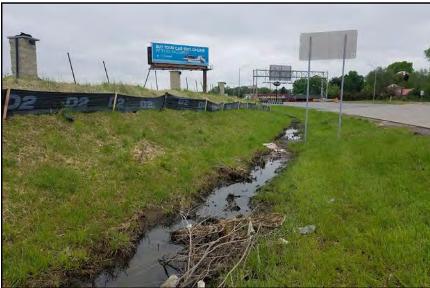
Photo 31, Ditch 2, Roadside, Facing Southwest.
