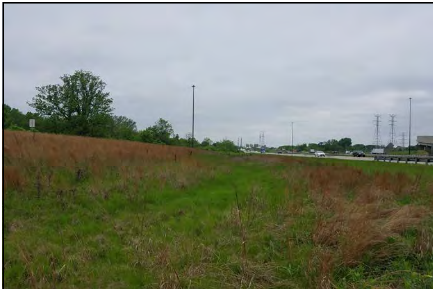
Photo 27, I-465, Facing Southwest.
