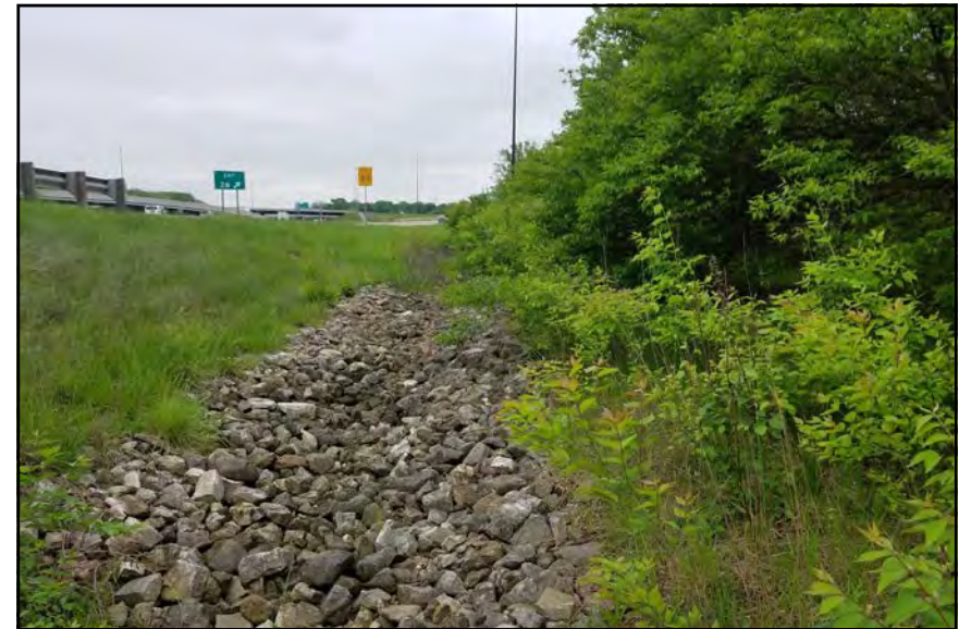
Photo 24, I-465 On Ramp, Facing Southeast.
