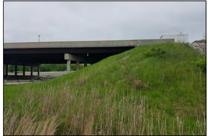
Photo 26, I-465, Facing Northeast.
