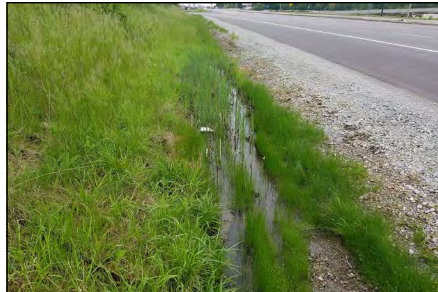
Photo 2, Data Point 01, Toe of Steep Slope, Facing North (Wetland 01).
