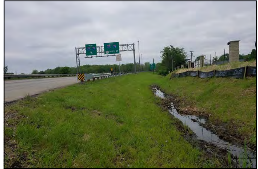
Photo 30, Ditch 2, Roadside, Facing Northeast.
