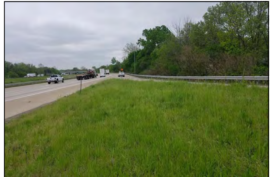
Photo 28, I-465 On Ramp and I-465 Facing East.
