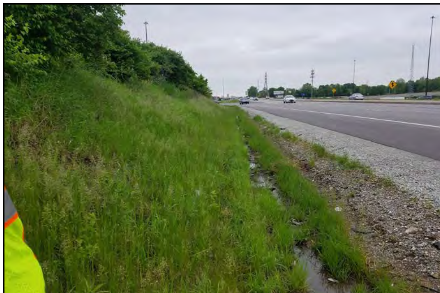
Photo 5, Upland Data Point 02, Steep Slope Above Wetland 01, Facing North.
