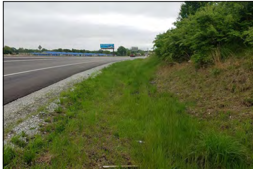
Photo 19, Ditch 1, Roadside, Facing Upstream.
