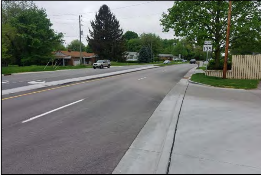
Photo 21, SR135, Facing West.
