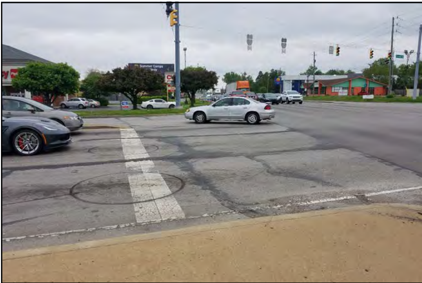
Photo 23, US31, Facing South.
