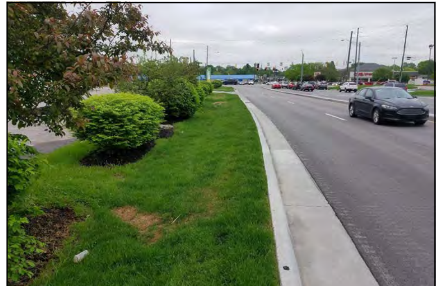
Photo 20, Project Limits on East Thompson Road, Facing Northeast.
