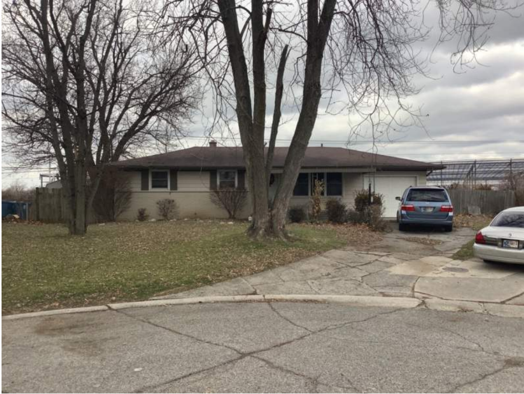
B-11. House at 2017 Tweedwood Drive, view to the northwest.
