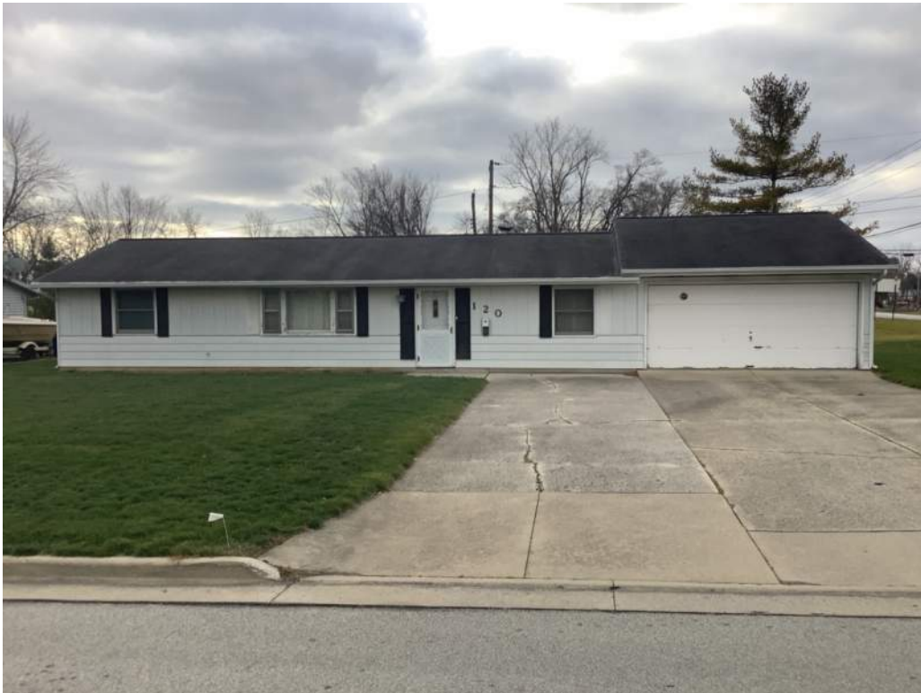
B-8. House at 120 Tanglewood Drive, view to the west.
