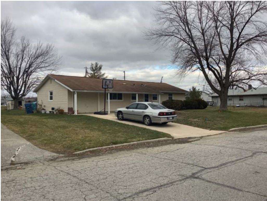
B-6. House at 1919 Tyland Boulevard, view to the north.
