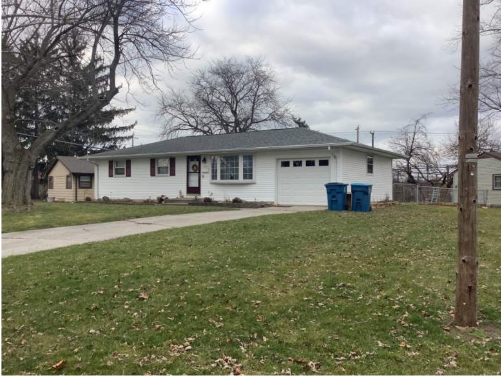
B-9. House at 2003 Tweedwood Drive, view to the northwest.
