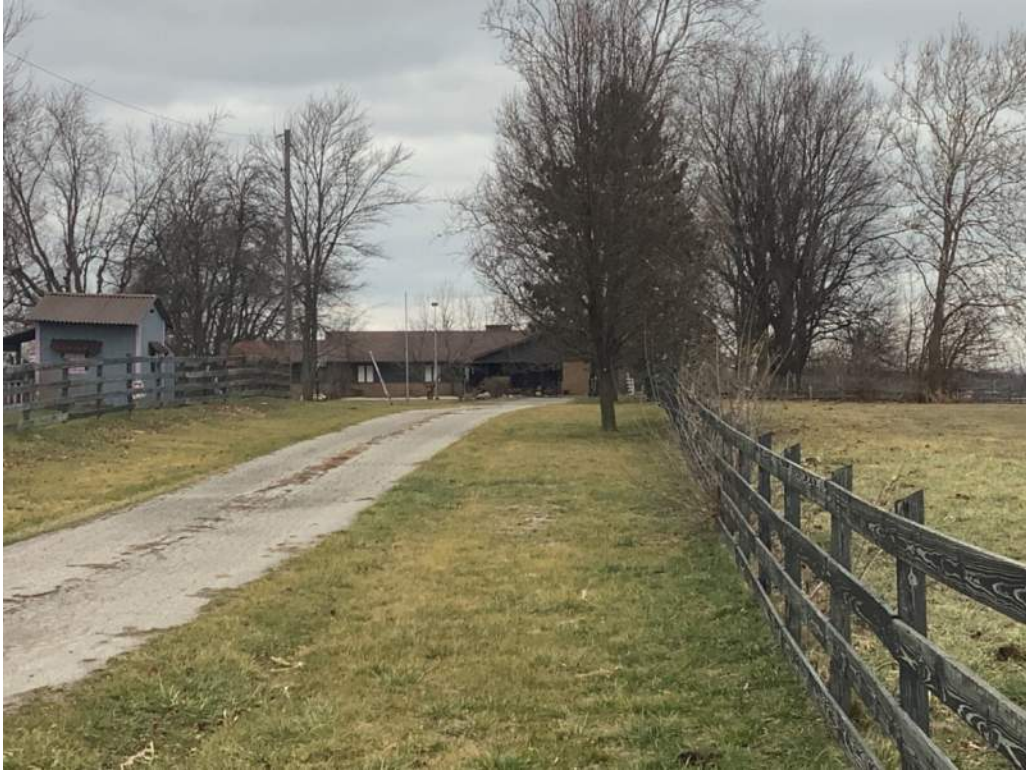
B-17. House at 11701 Edgerton Road, view to the north.
