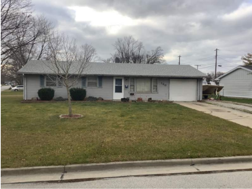
B-7. House at 130 Tanglewood Drive, view to the west.
