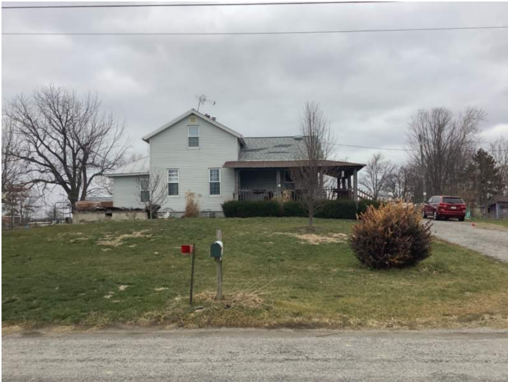
B-16. House at 11613 Edgerton Road, view to the north.
