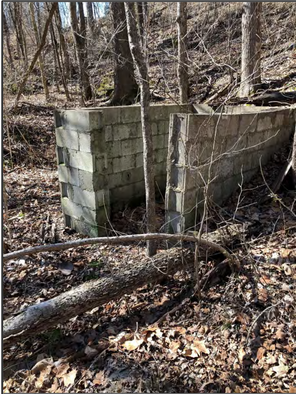
Figure 8. Modern concrete-block structure associated with a monitoring well situated within the survey area, facing west.
