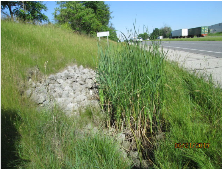
Photo 14: Southwest Quadrant Looking northwest from south side of US 30 at riprap with cattails in RSD-2.
