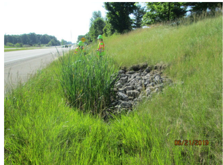
Photo 16: Southwest Quadrant Looking southeast along US 30 at riprap with cattails in RSD-2.
