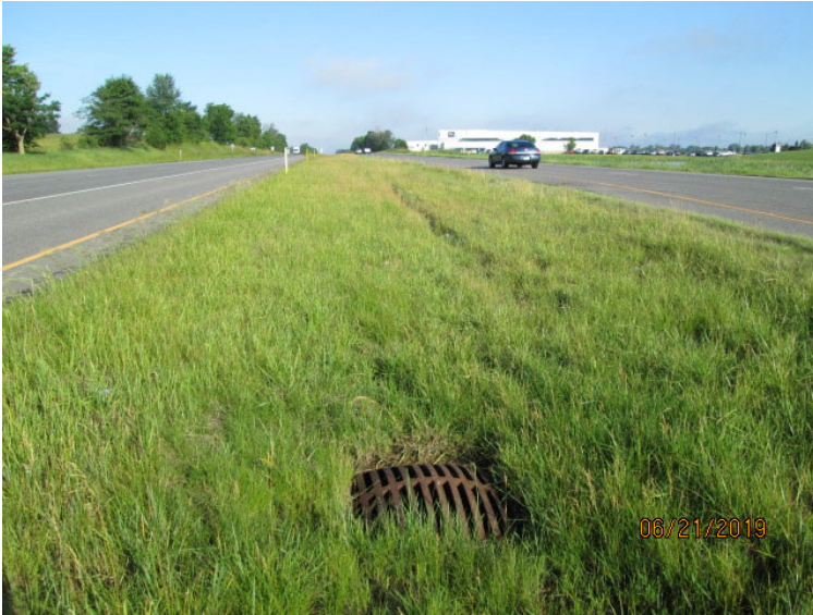
Photo 9: Western Median Looking northwest in the median on the west side of the intersection of US 30/CR 500 E. Shown inlet is Structure No. 102 on plans.
