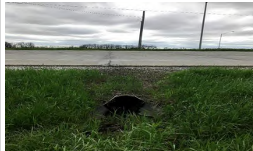
Photo 3. Looking east toward a drainage pipe that runs underneath US 421, approximately 0.02 mile north of the US 6 and US 421 intersection.
