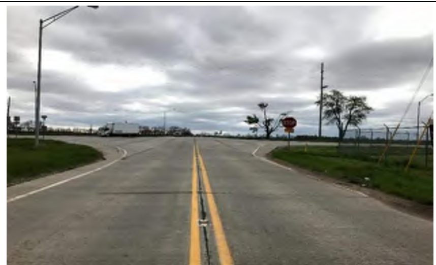
Photo 12. Looking west from the center of CR W. 600 S., approximately 0.03 mile west of the US 6 and US 421 intersection.
