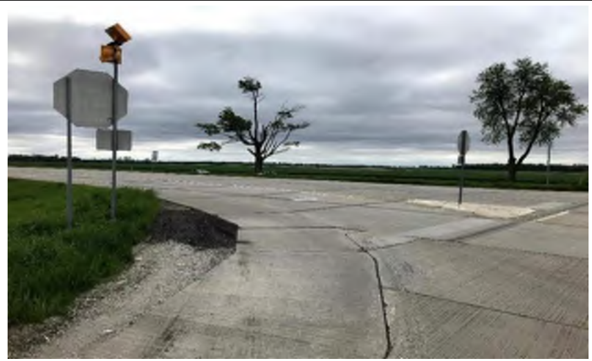
Photo 26. Looking southeast toward US 6, from the northeast corner of the US 6 and US 421 intersection.
