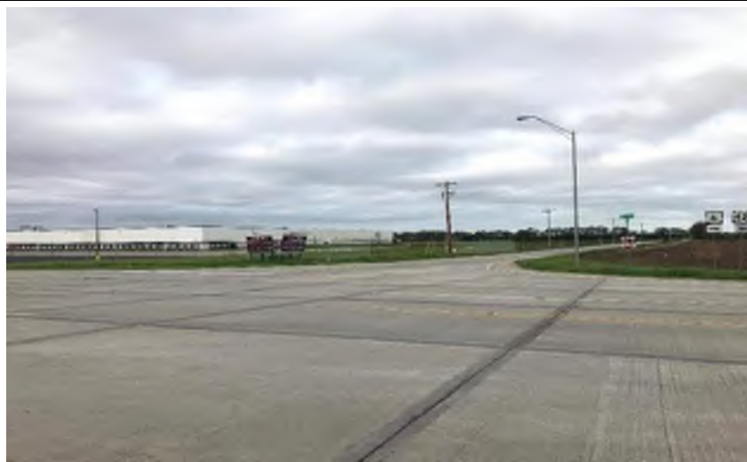
Photo 27. Looking southwest toward the US 6 and US 421 intersection.
