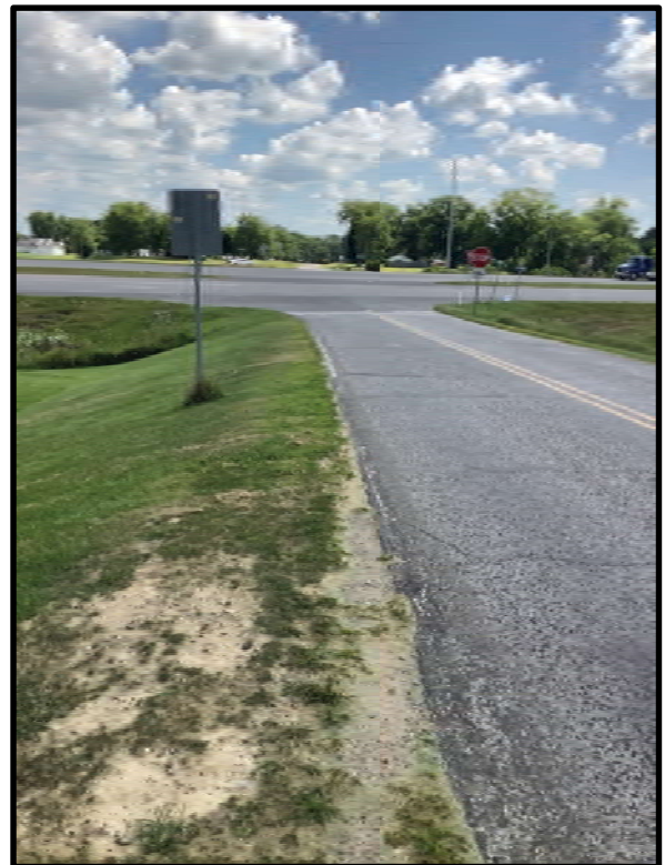
4. View east of mowed ROW along northside of western leg of Waits Rd towards SR 3 intersection. 8/4/2021
