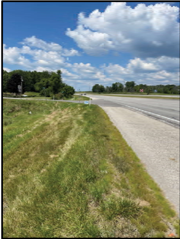
1. View north of mowed right-of-way (ROW) along westside of the south leg of SR 3, towards Waits Rd. 8/4/2021
