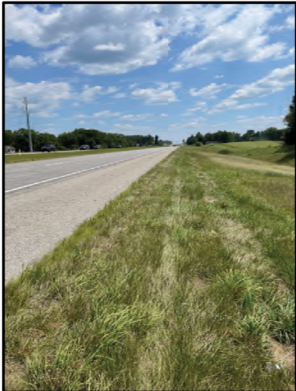
14. View south of mowed ROW along westside of the south leg of SR 3. 8/4/2021.
