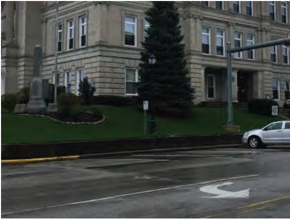
Figure 15: Looking northeast at the wide curb surrounding the Putnam County Courthouse. The curb and wall are anticipated to be maintained.
