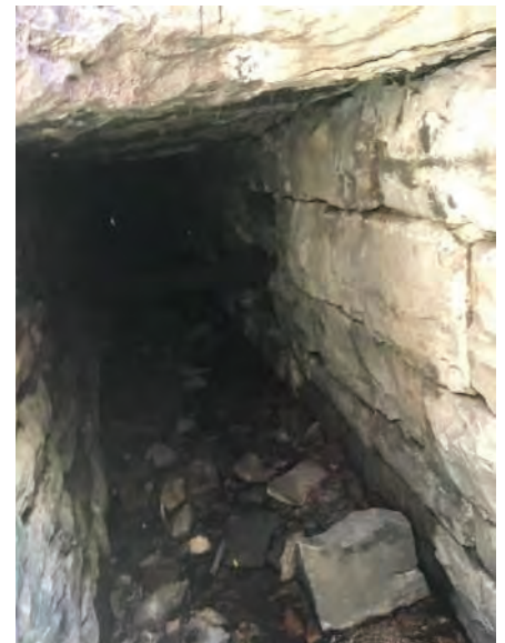
Figure 16: View inside stone drainage structure.
