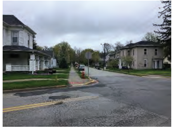
Figure 1: Looking east at the typical pavement condition and existing curb ramps along Bloomington Street and within the Eastern Enlargement Historic District.
