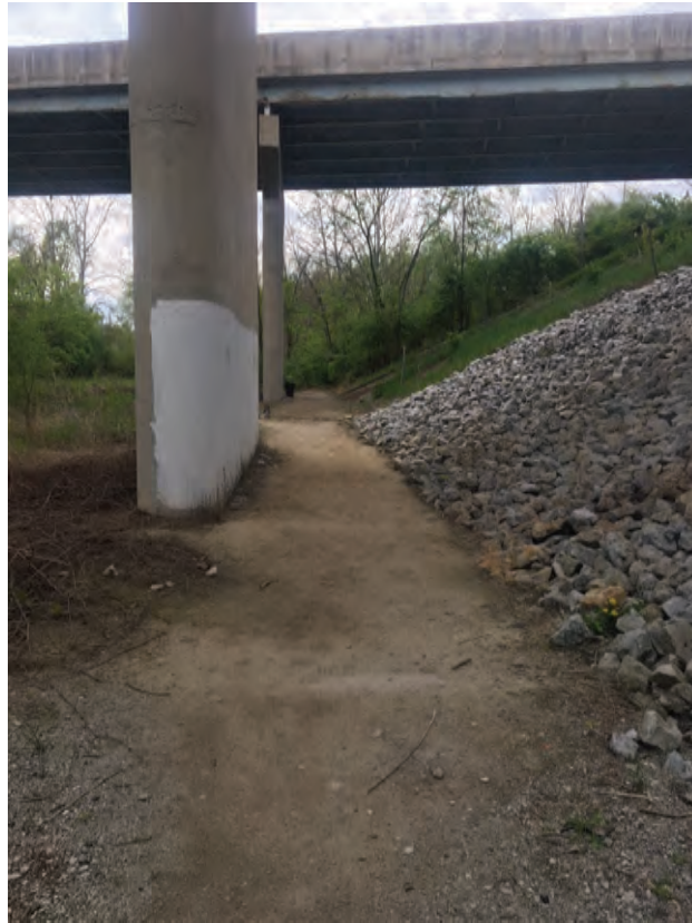
13. Facing Wabash Heritage Trail under 9th Street bridge, looking southwest
