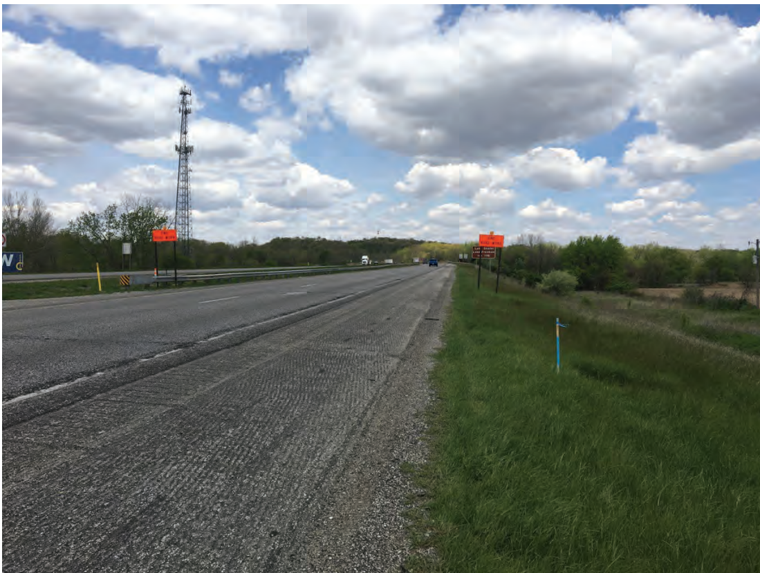
8. Facing I-65 northbound, looking north
