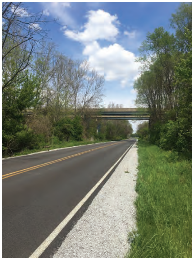
10. Facing I-65 over 9th Street bridge, looking northeast
