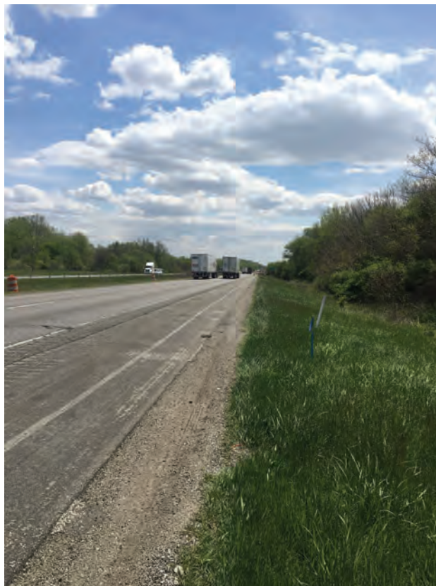
2. Facing I-65 southbound, looking south
