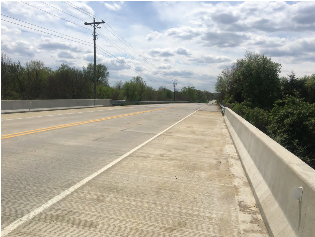
7. Facing Swisher Road at bridge over I-65, looking southwest
