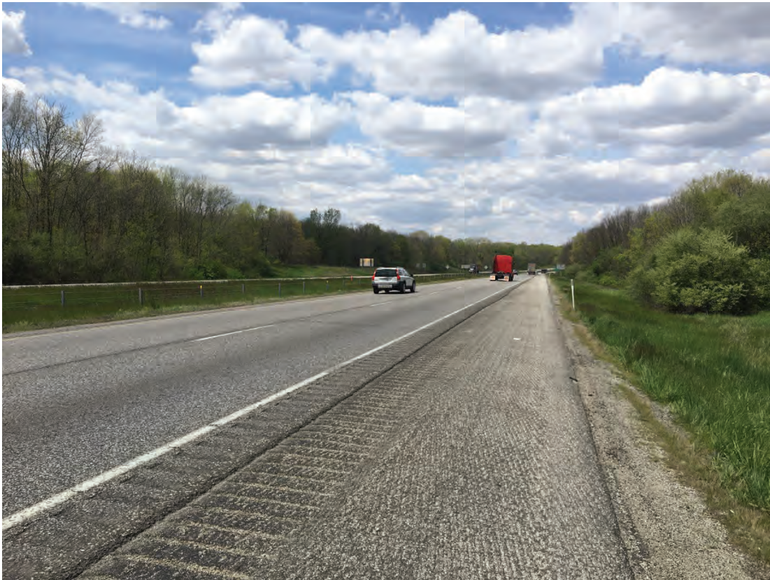
21. Facing I-65 northbound, looking northwest
