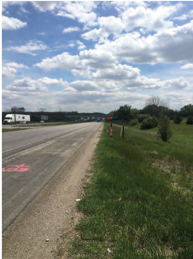
9. Facing I-65 southbound, looking south
