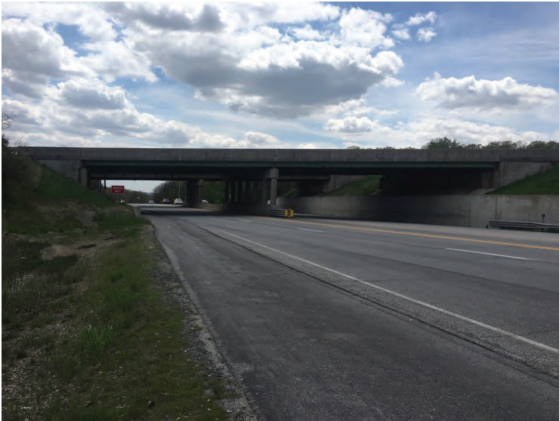
19. Facing I-65 bridges over SR 43, looking south
