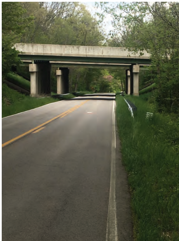
16. Facing I-65 bridge over Prophets Rock Road, looking northeast
