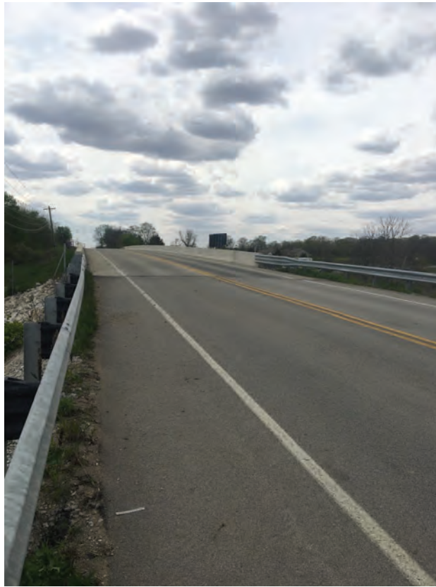
23. Facing CR 600 bridge over I-65, looking west
