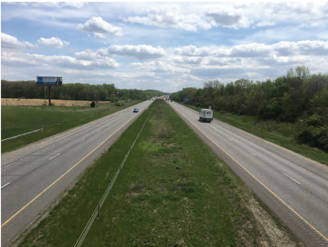
4. Facing I-65 at Swisher Road bridge, looking south
