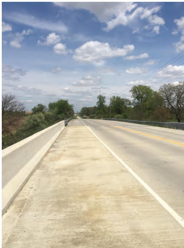
6. Facing Swisher Road at bridge over I-65, looking northeast
