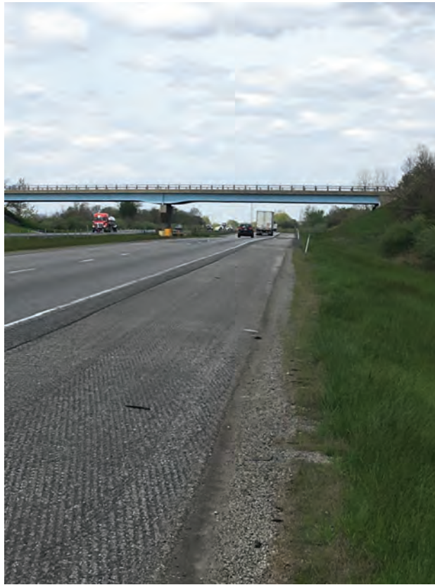
27. Facing CR 725 bridge over I-65, looking northwest
