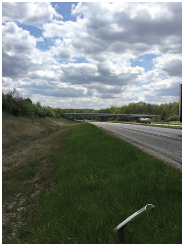
24. Facing CR 600 bridge over I-65, looking southeast
