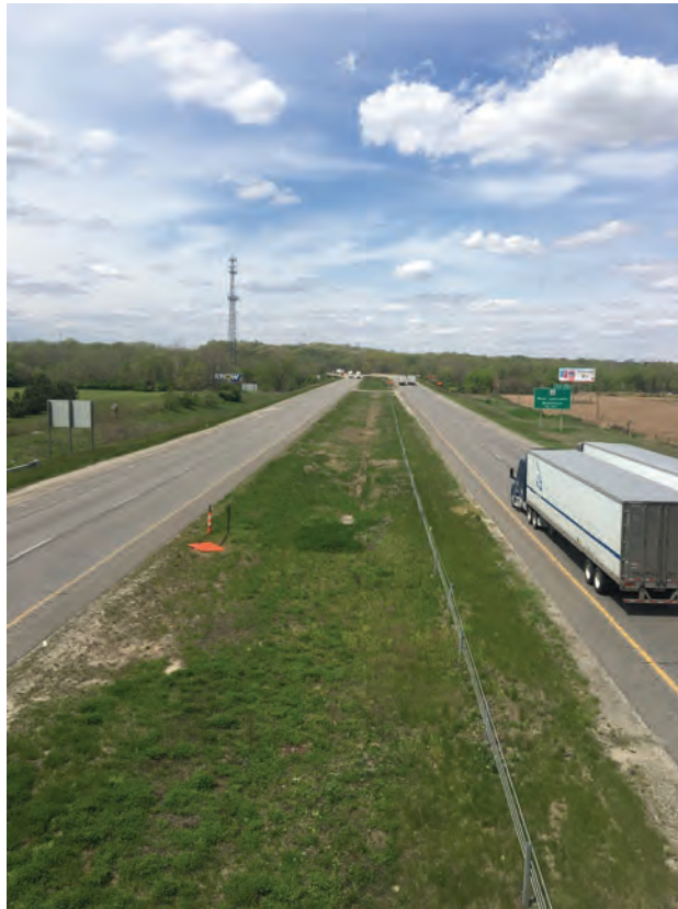
5. Facing I-65 at Swisher Road bridge, looking north
