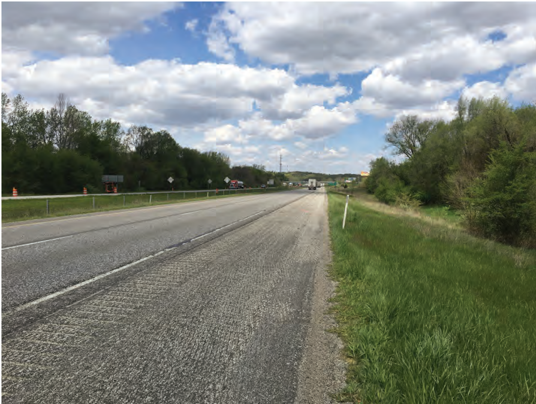
1. Facing I-65 northbound, looking north
