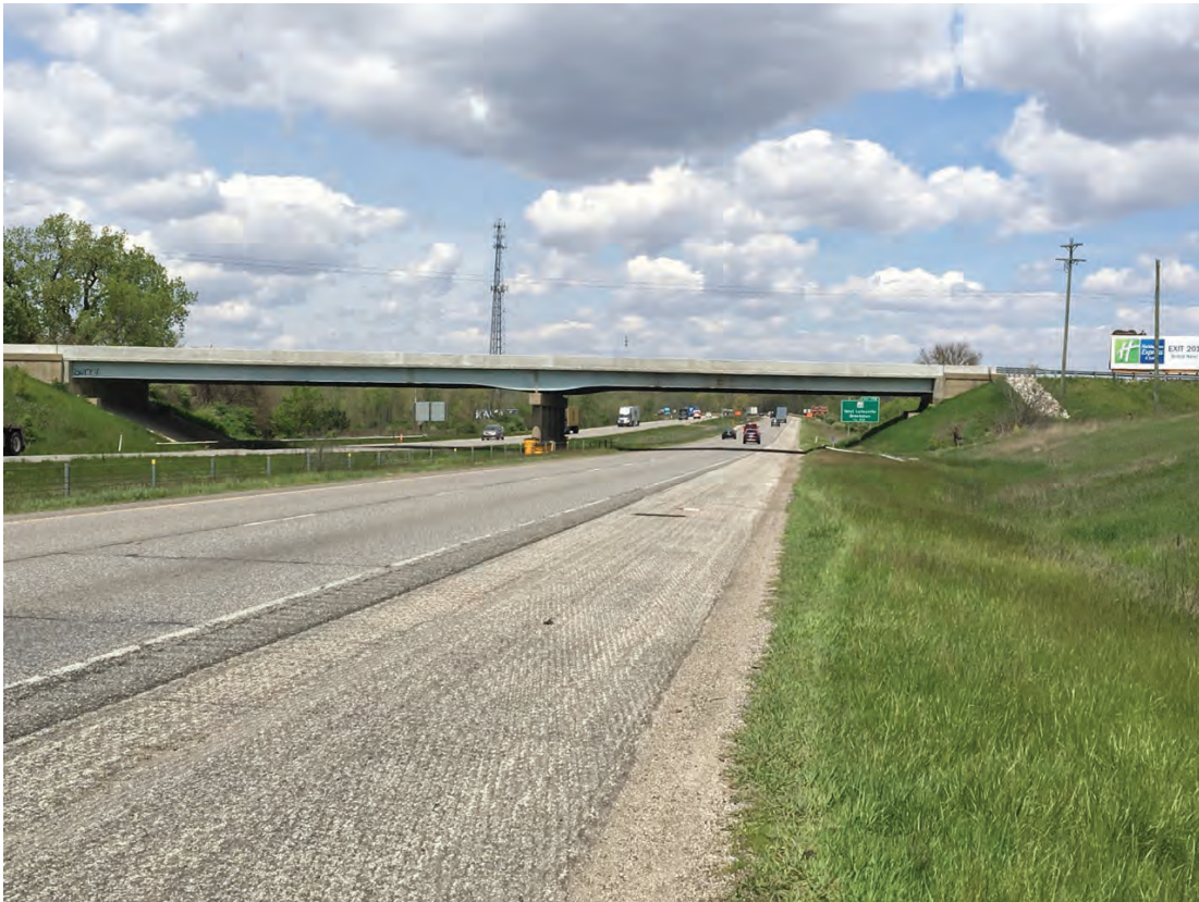
3. Facing I-65 northbound, looking north at Swisher Road bridge
