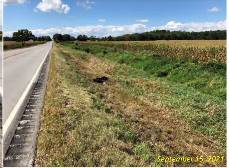
Photo 26: View west along the north side of SR 8 from west of the small structure.
