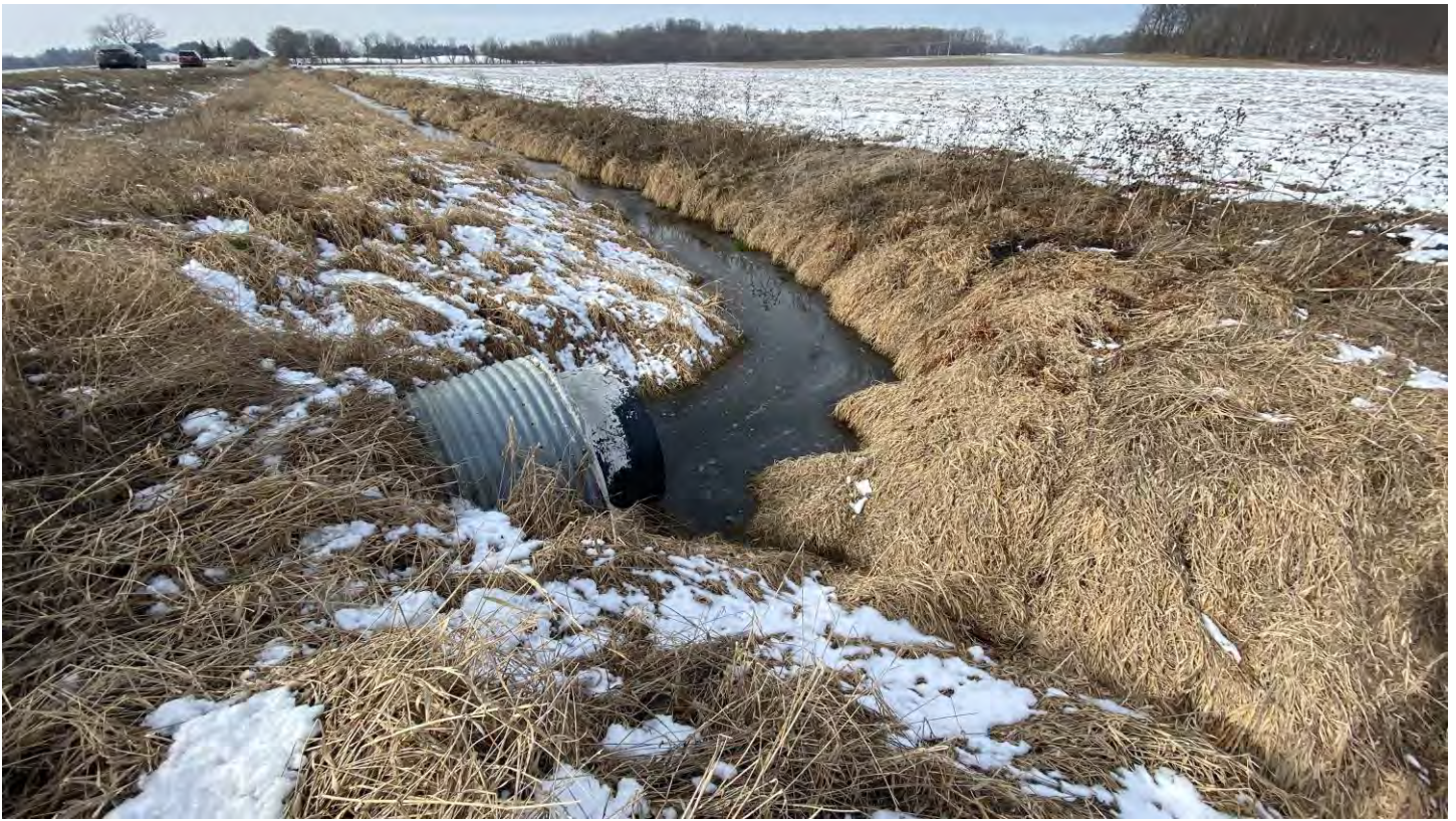
Photo 3 – View westerly, north end of small structure CV 008-057-47.08
