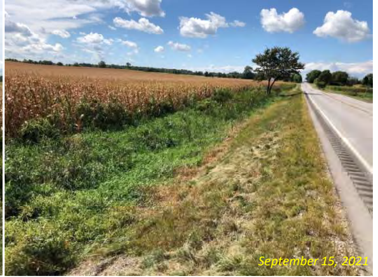
Photo 22: View west along the south side of SR 8 from near the west study limit. Wetland A is also shown.
