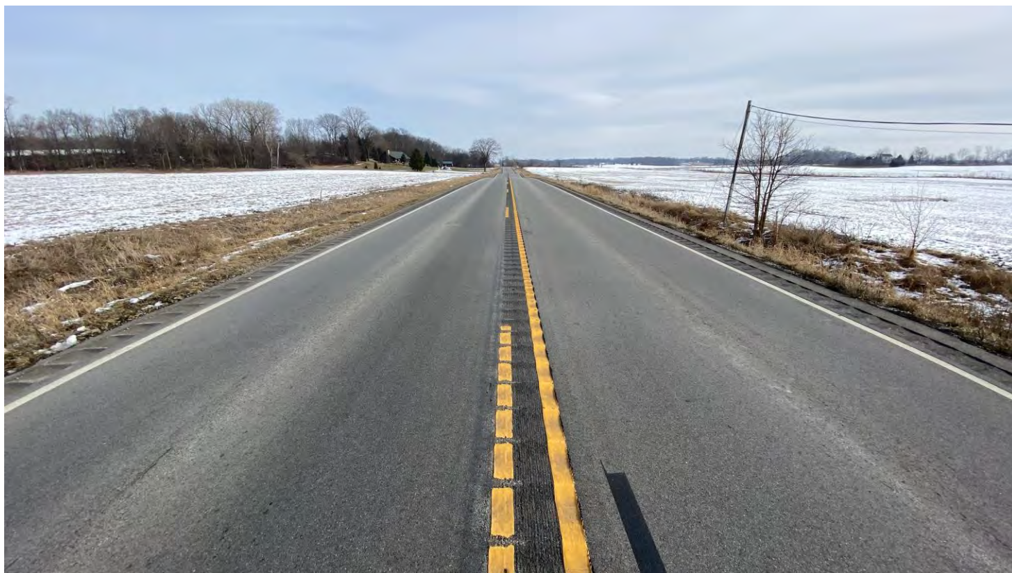
Photo 2 – View easterly along SR 8 from small structure CV 008-057-47.08
