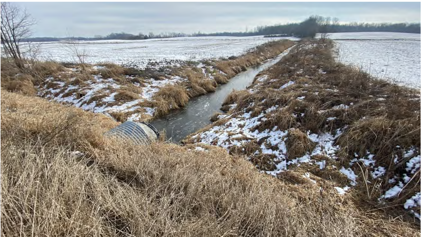
Photo 4 – View southeasterly, south end of small structure CV 008-057-47.08
