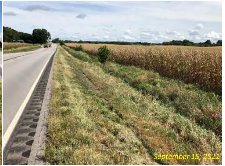
Photo 30: View east along the south side of SR 8 from east of the small structure. Wetland B is also shown.
