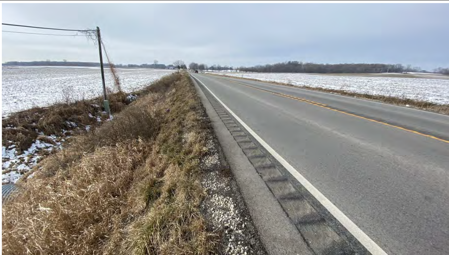
Photo 1 – View westerly along SR 8 from small structure CV 008-057-47.08
