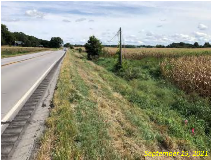
Photo 23: View east along the south side of SR 8 from west of the small structure. Wetland A is also shown.
