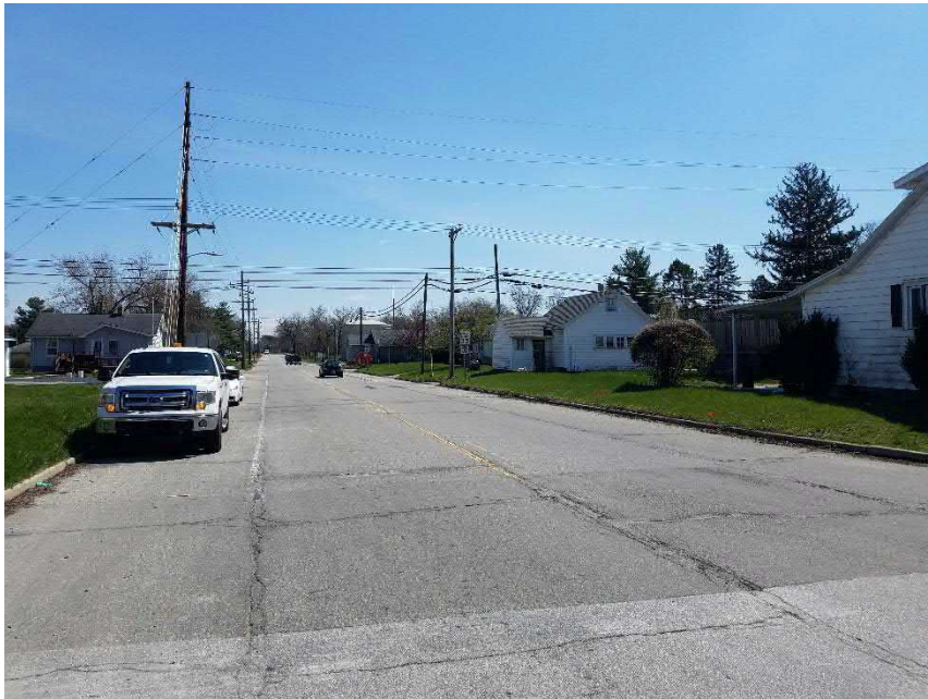
Photo 2. SR 14 and SR 35 Intersection Facing East
