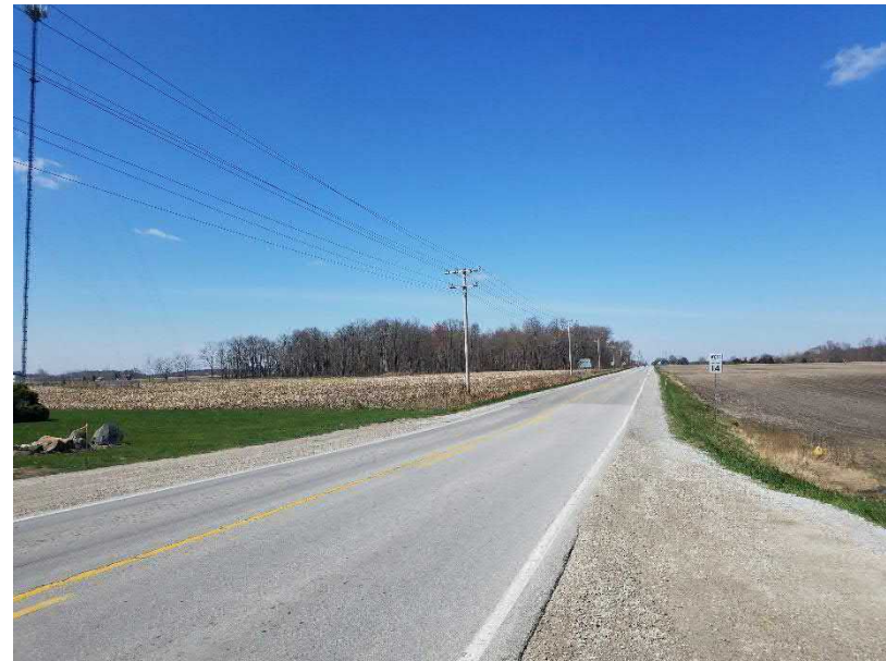
Photo 27. SR 14 and SR 17 Intersection Facing West
