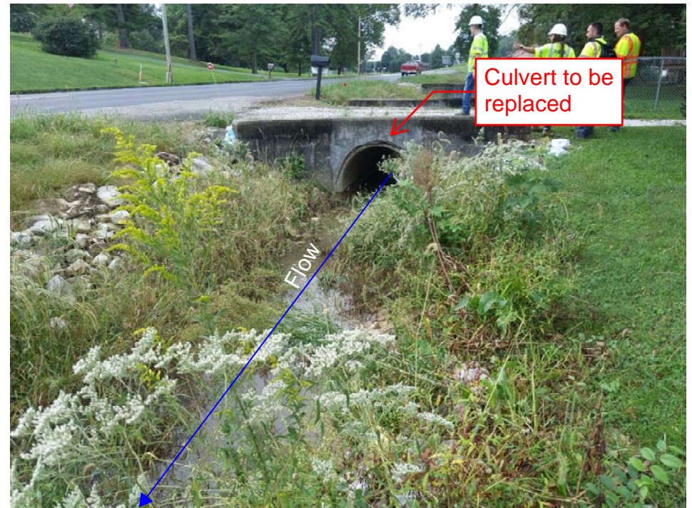
8. View of investigated area and UNT to Bruner Creek looking southwest.
