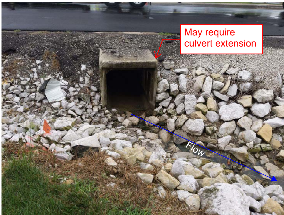
17. View of UNT 3 and culvert that carries stream beneath US 231
