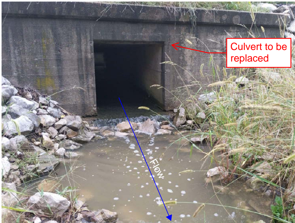
11. Looking southwest to UNT to Bruner Creek and driveway culvert
