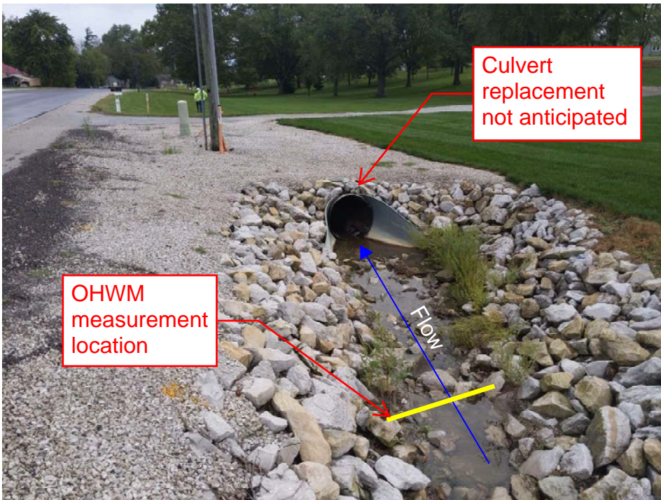
23. Looking northeast to investigated, UNT 2, and inlet to enclosed drainage system
