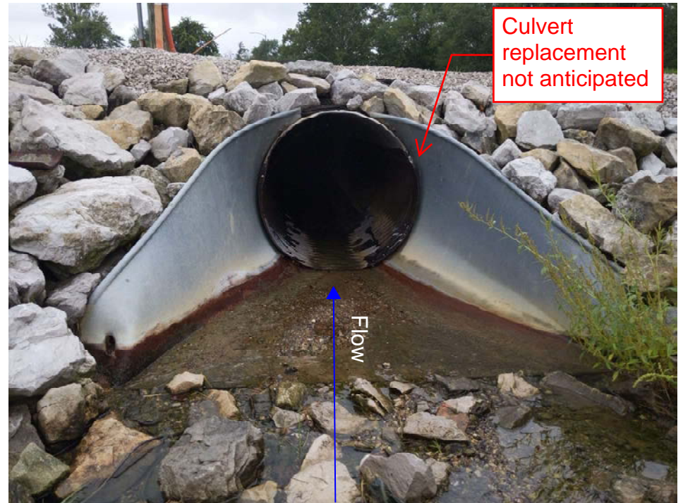
16. Looking north to UNT 2 and inlet to enclosed drainage system
