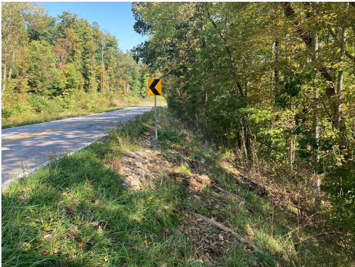
9 – View of SR 237 road embankment facing north
