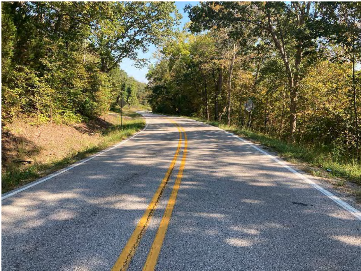
14 – View of survey area facing northeast
