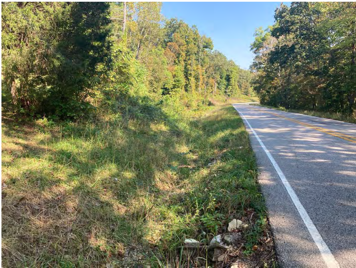
7 – View of RSD1 facing north
