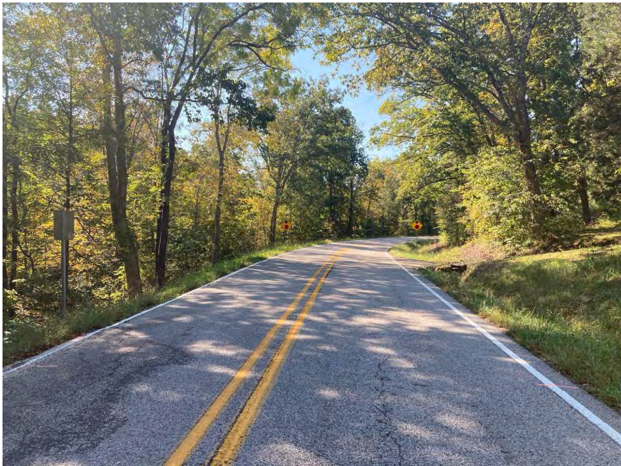
6 – View of survey area facing southwest; RSD1 is on the west
