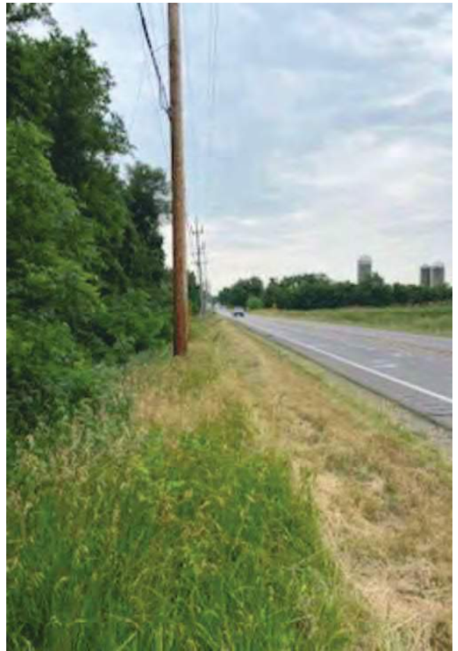
14-Facing South from East Side of SR15 From North Terminus
