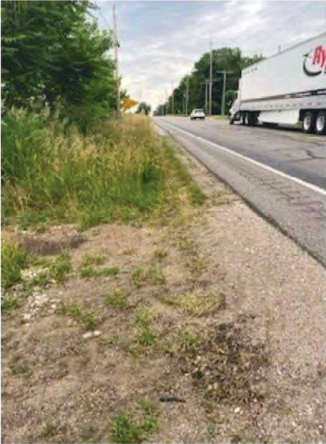
17- Facing North from West Side of SR 15
