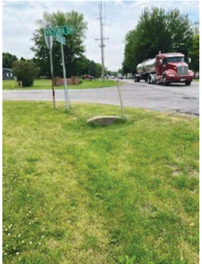
4- Facing South at Victoria Drive, failed pipe Appendix B - 5
