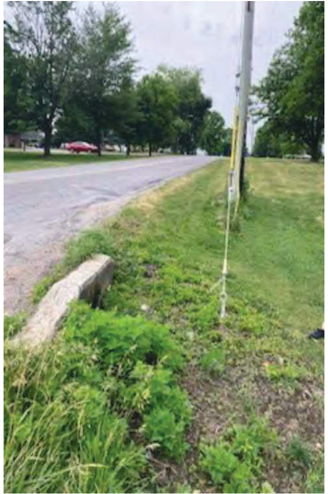
6- Facing West from Pipe under CR 18, Northwest Quadrant
