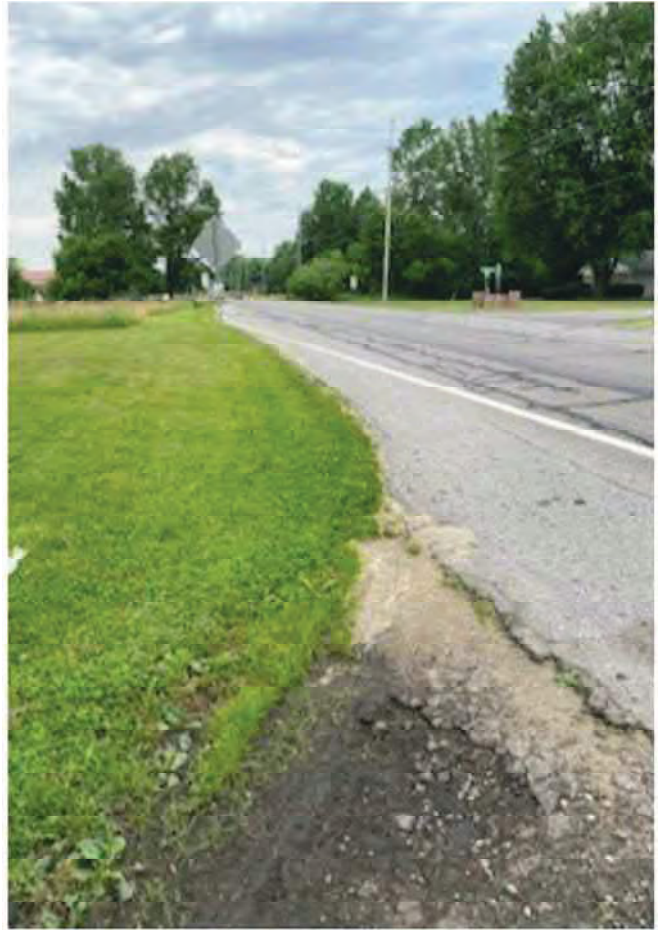
18-North Facing to Intersection from South Terminus
