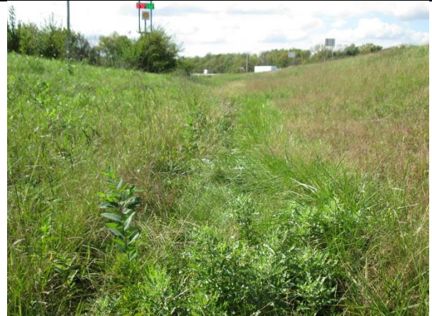
4. Looking west at roadside ditch along I-70 east bound exit ramp.
