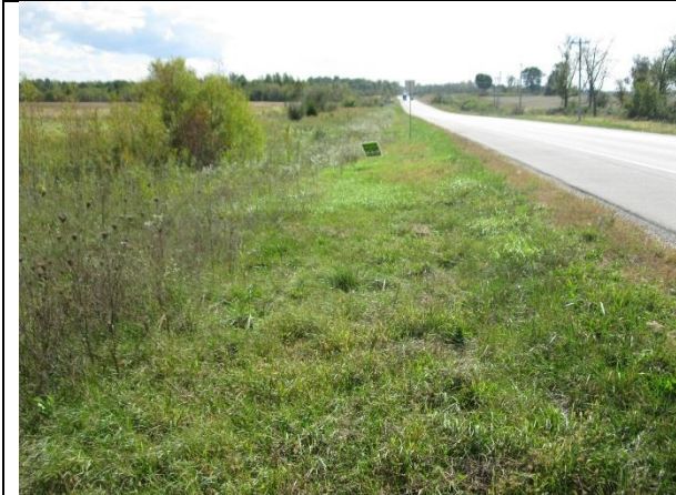
3. Looking south at east road side along SR 39.
