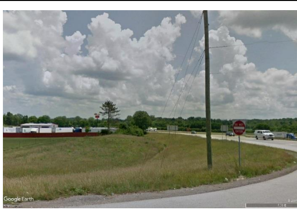
12. Looking east at roadside ditch lined with concrete. From north side of SR 39/I-70 Interchange.
