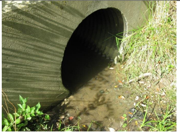
8. Looking at culvert outlet draining from wetland 8 within southeast interchange area.
