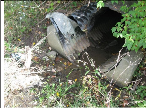
7. Looking at culvert inlet draining under frontage road south of I-70.
