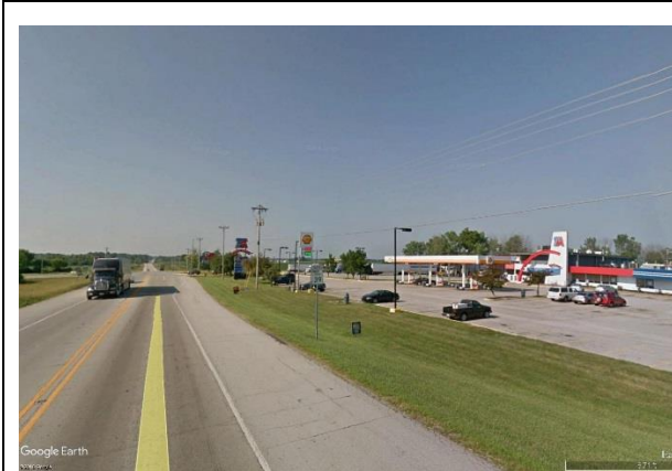
5. Looking southwest at roadside swale from SR 39 on south side of SR 39/I-70 interchange.
