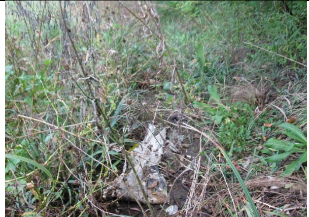
6. Looking northeast at roadside ditch south of east bound entrance ramp from SR 39 to I-70.
