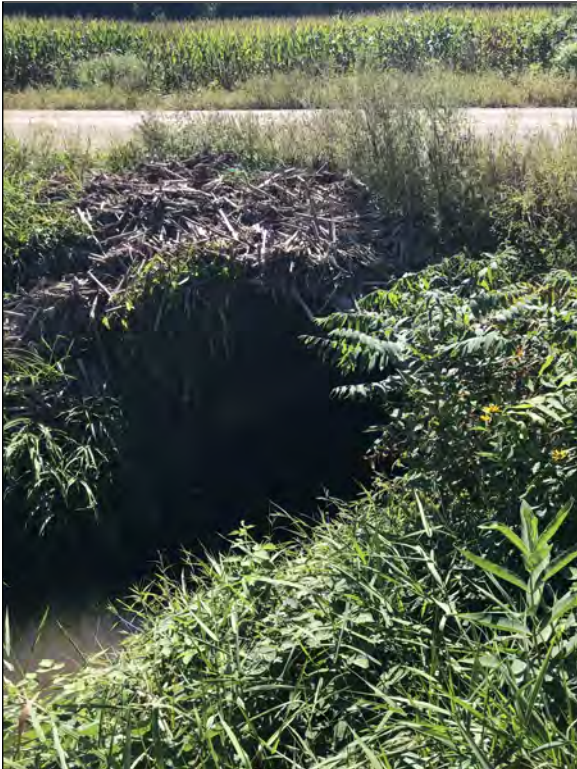
Picture 13—UNT to Lick Creek and project structure; southeast view; 9 SEP 2021.
