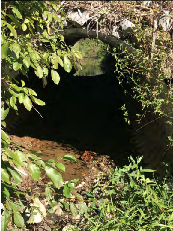
Picture 5—UNT to Lick Creek east project structure; northwest view; 9 SEP 2021.
