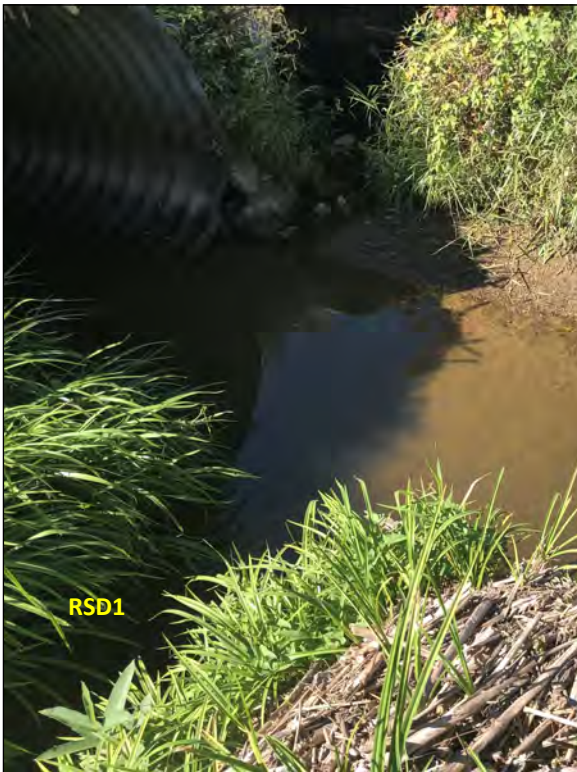
Picture 11—UNT to Lick Creek at RSD1; southwest view; 9 SEP 2021.
