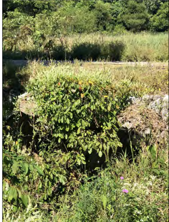
Picture 42—Southeast quadrant and project structures; northwest view; 9 SEP 2021.
