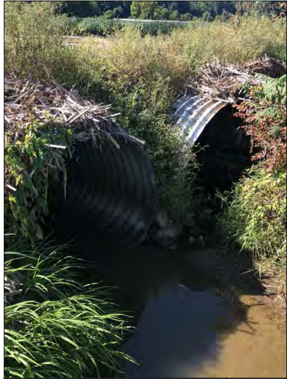
Picture 10—UNT to Lick Creek project structure; southwest view; 9 SEP 2021.
