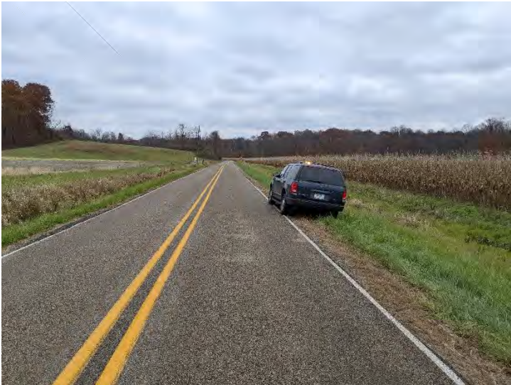
Photo 5: View of the roadway looking westbound
