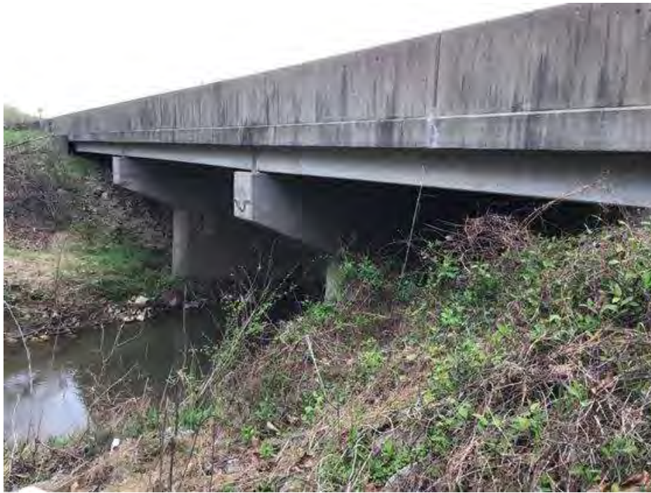
PHOTO 1 Elevation, Condition Description West side.
