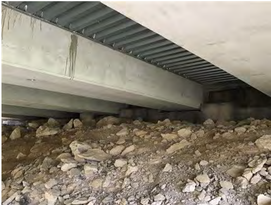
PHOTO 18 Condition Description North abutment.
