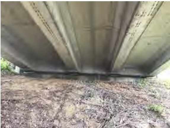
File Description Abutment #1 facing West
