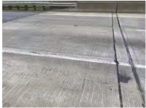
File Description North joint and approach slab.
