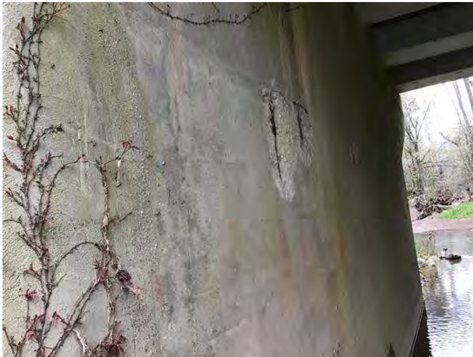
PHOTO 14 Condition Description Pier 2 north side.
