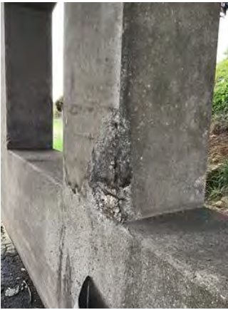
File Description Pier 4 column 2. File Type Category Condition, Other
