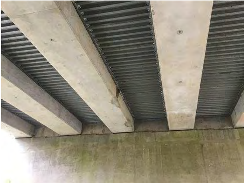
PHOTO 9 Condition Description Span B facing north.
