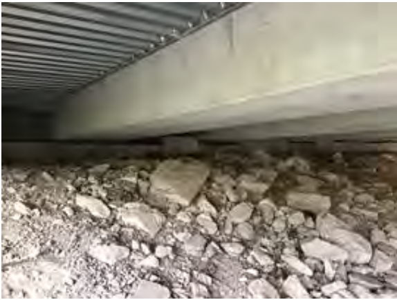
File Description South abutment. File Type Category Condition
