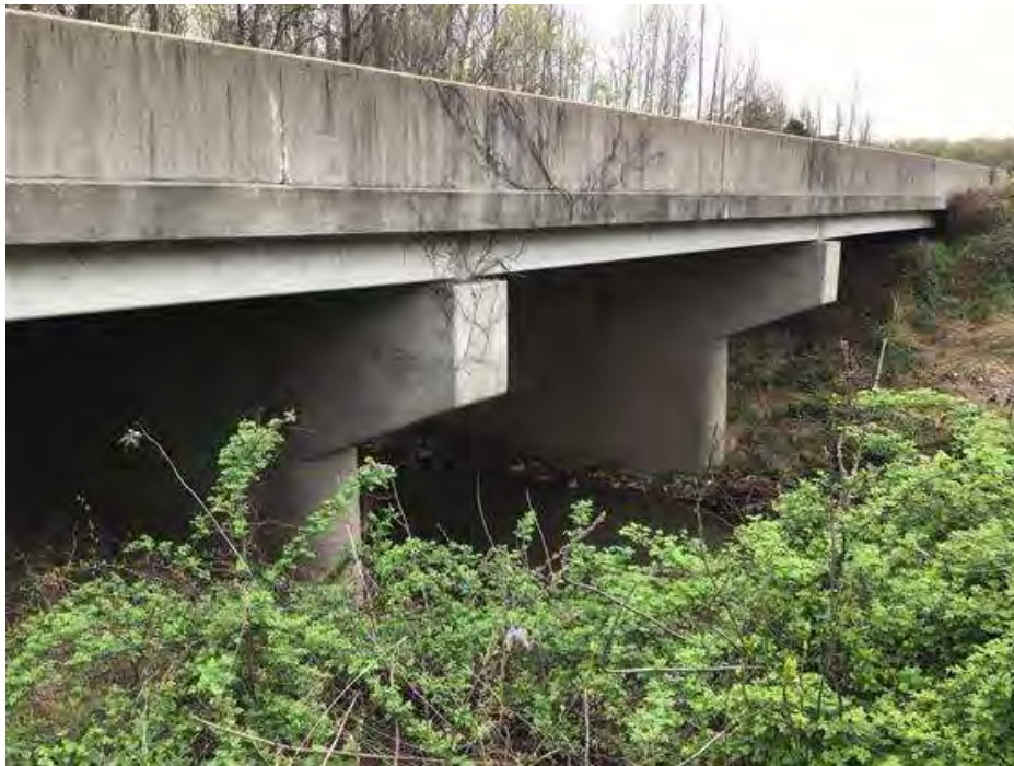
PHOTO 2 Elevation, Condition Description East side.
