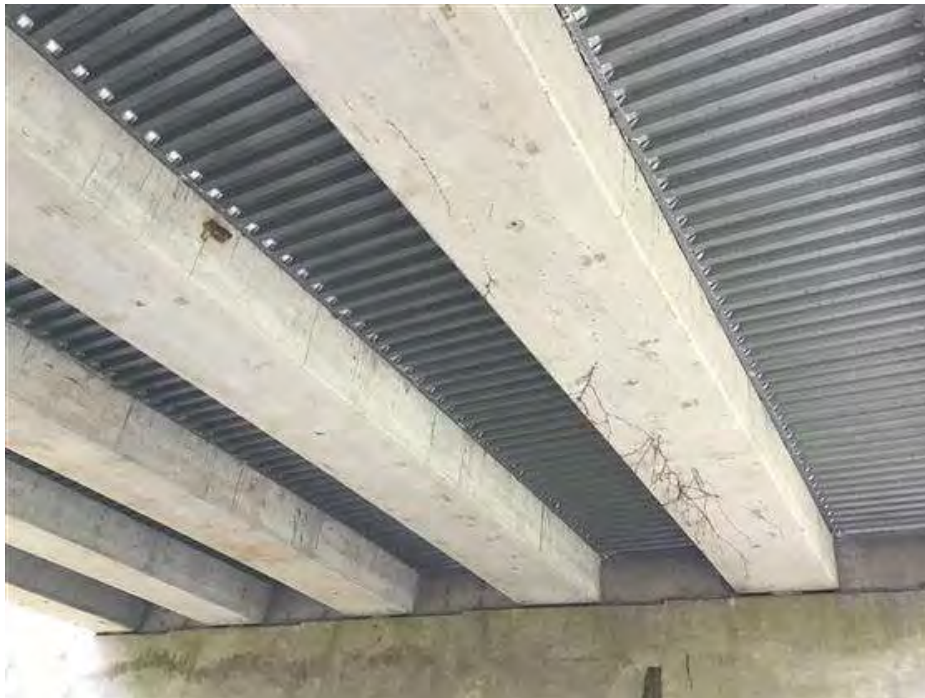
PHOTO 10 Condition Description Span B facing north.
