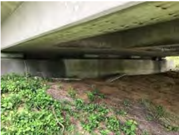
File Description West abutment.
