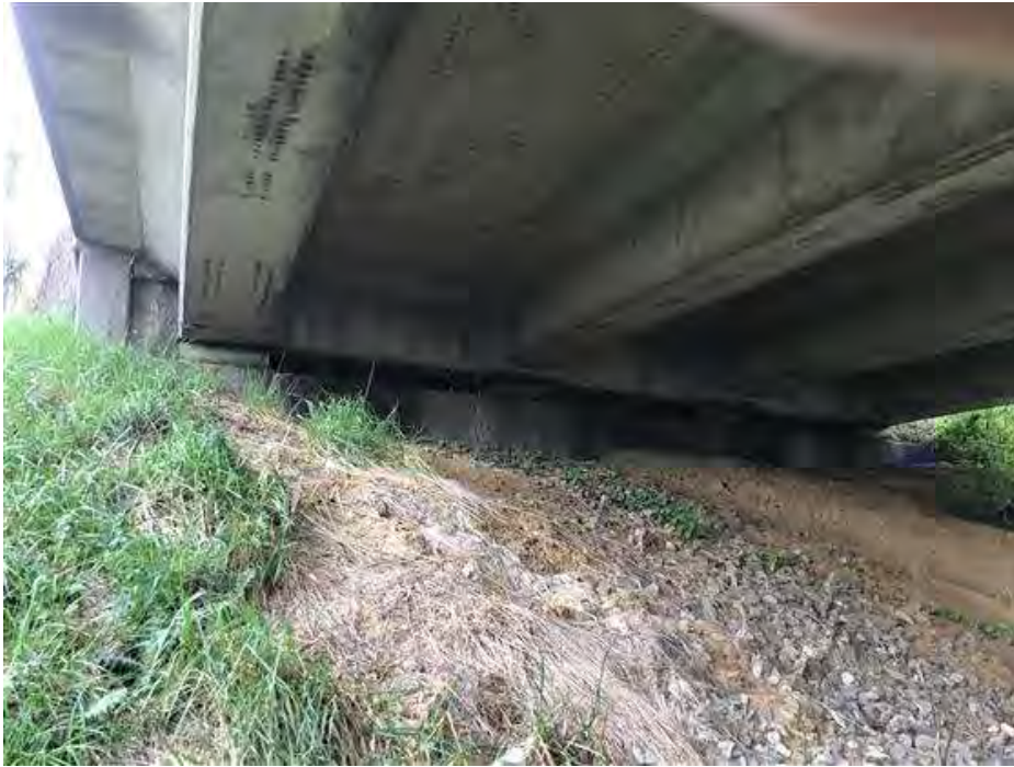
PHOTO 21 Condition Description Abutment #5 facing East
