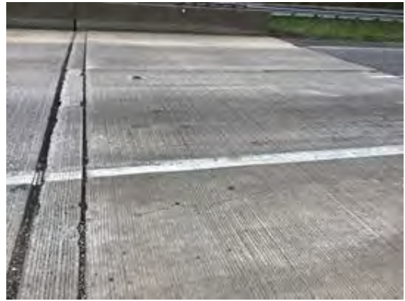
File Description North joint and approach slab.
