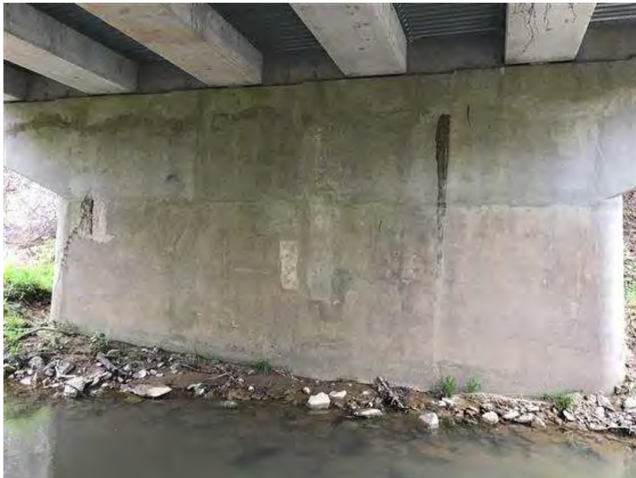
PHOTO 16 Condition Description Pier 3 south side.
