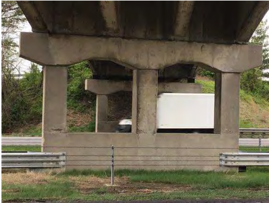
PHOTO 15 Condition Description Bent #3 facing West
