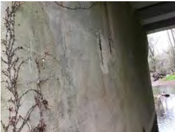
File Description Pier 2 north side.
