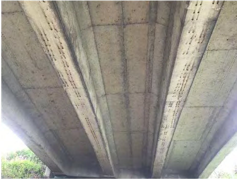
PHOTO 9 Condition Description Underside Span A facing West
