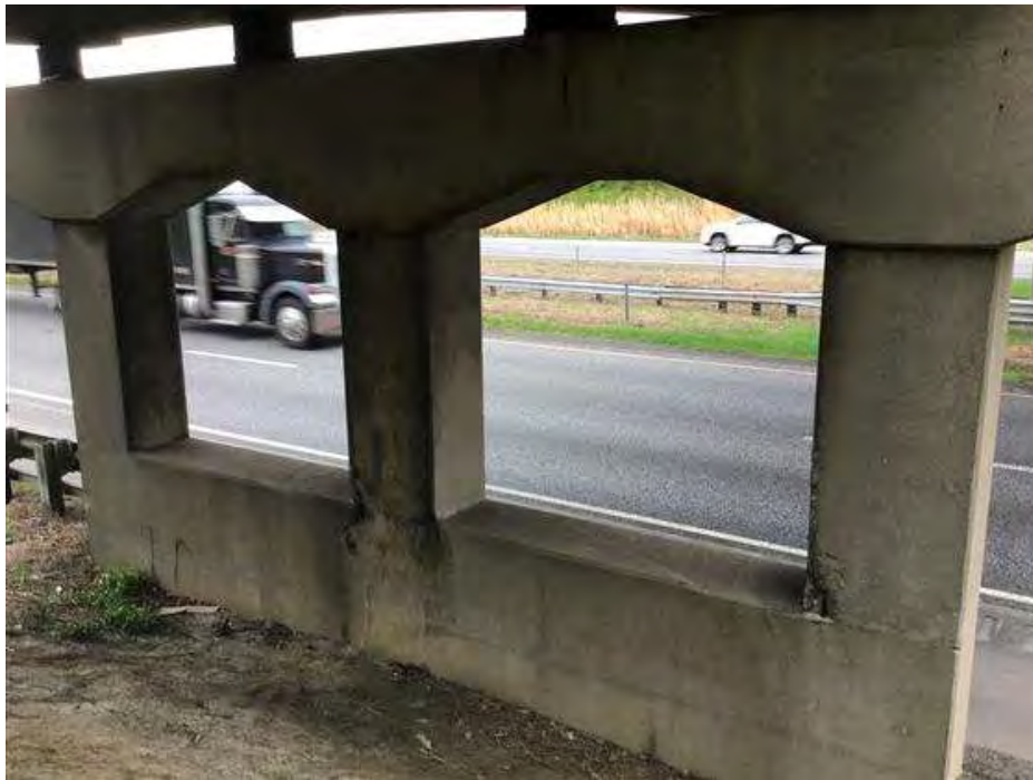
PHOTO 10 Condition Description Bent #2 facing East
