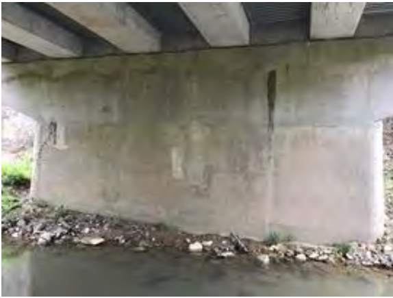
File Description Pier 3 south side.
