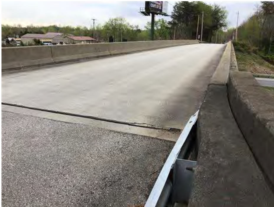
PHOTO 4 Condition Description Roadway east.
