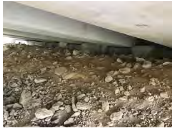
File Description South abutment.
