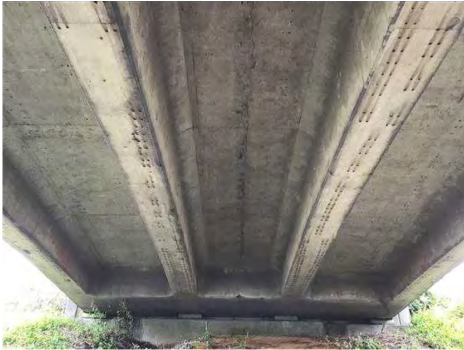
PHOTO 11 Condition Description Span D facing east.
