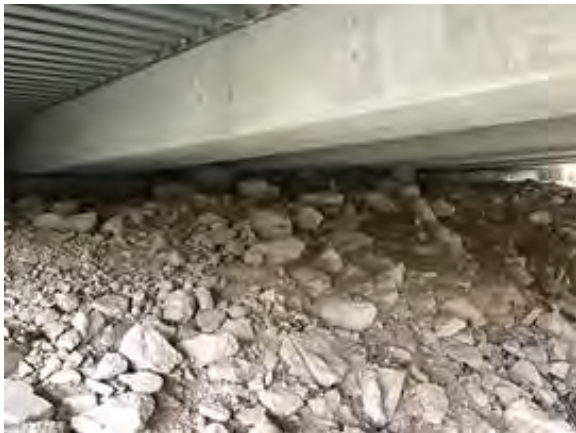
File Description North abutment.
