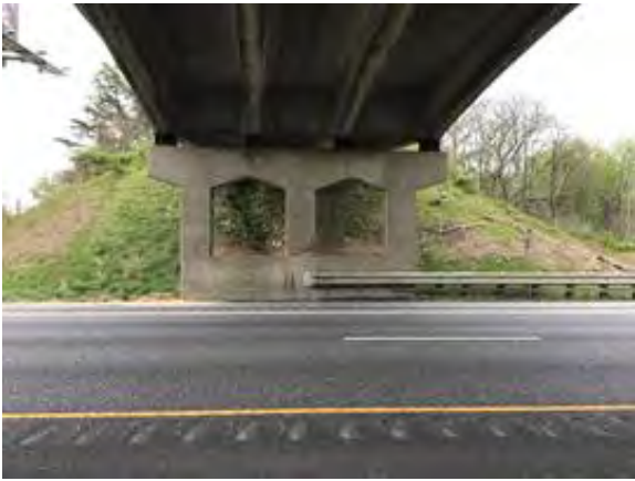
File Description Pier 4 facing east.
