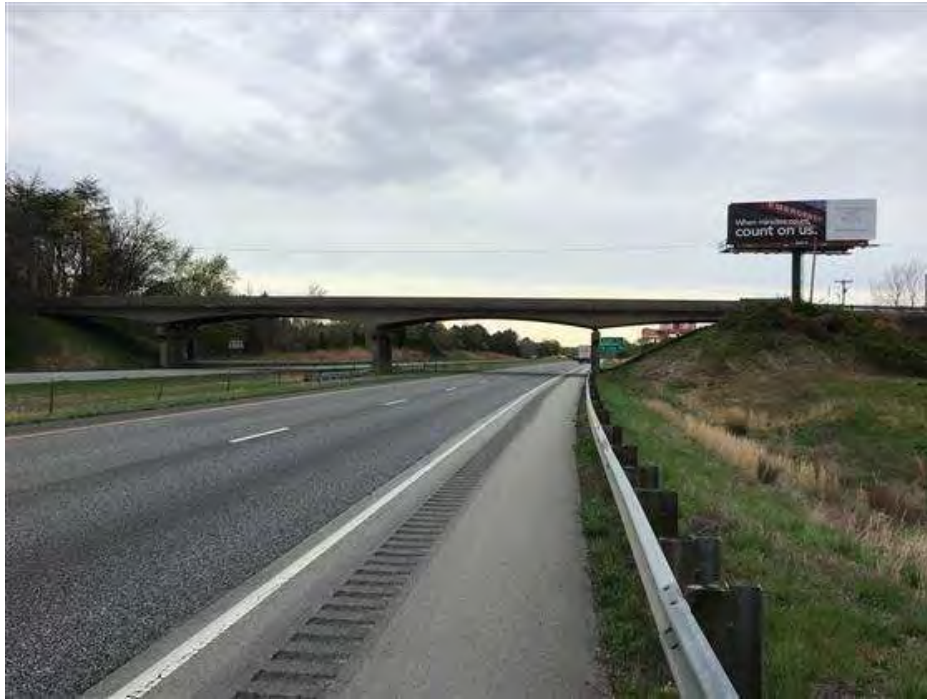
PHOTO 1 Elevation, Condition Description South side.
