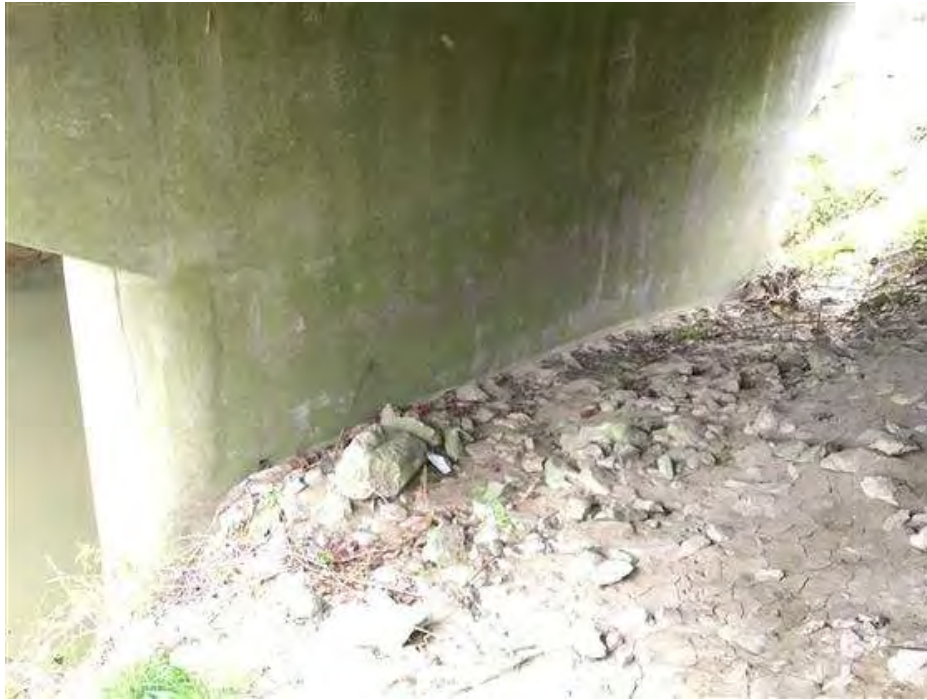
PHOTO 15 Condition Description Pier 3 north side.
