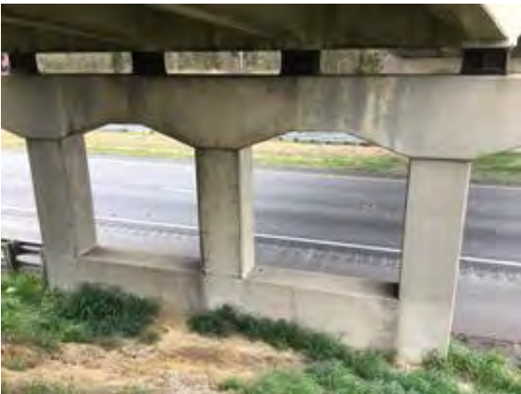
File Description Bent #4 facing West File Type Category Condition
