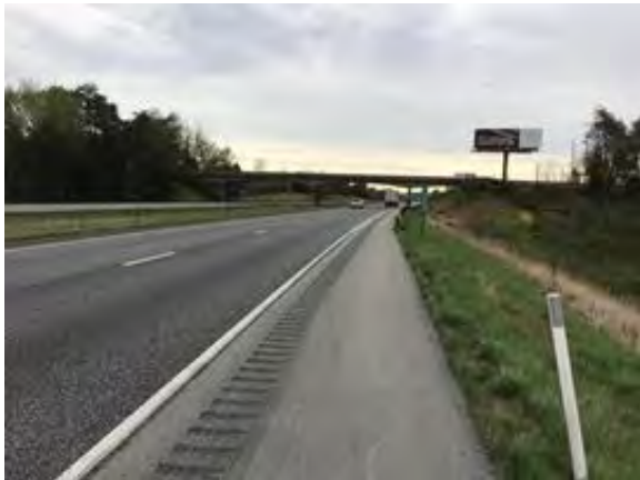
File Description South side. File Type Category Condition, Elevation
