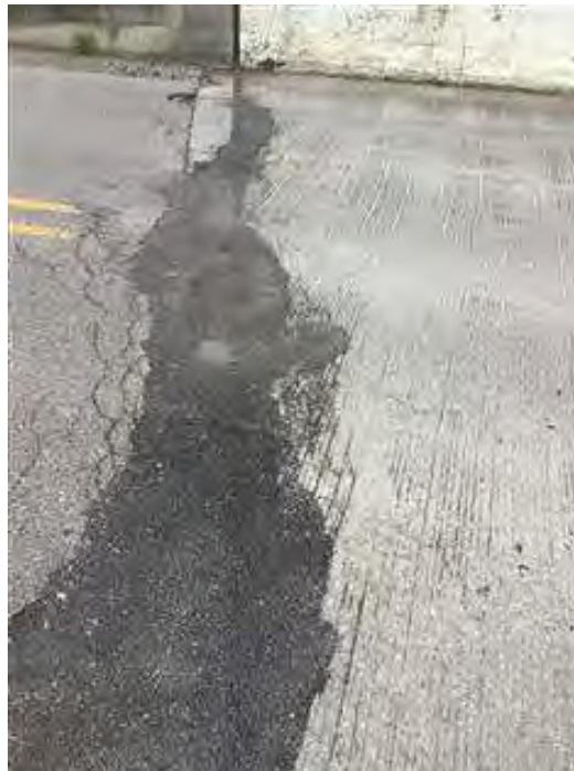
PHOTO 6 Condition, Maintenance - Bridge Description East Joint facing South
