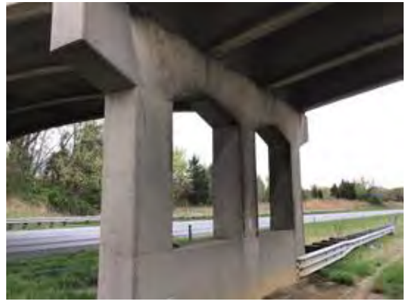
File Description Pier 3 east side.
