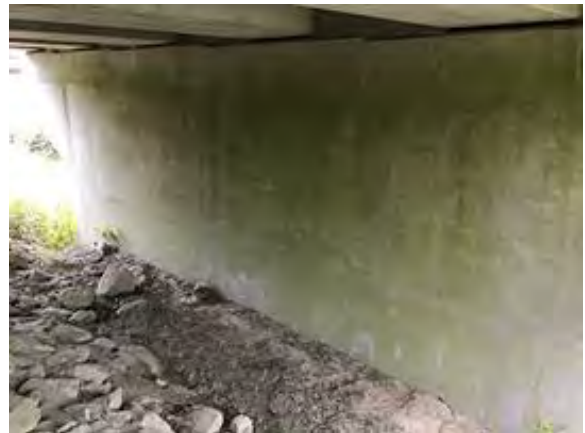
File Description Pier 2 south side.
