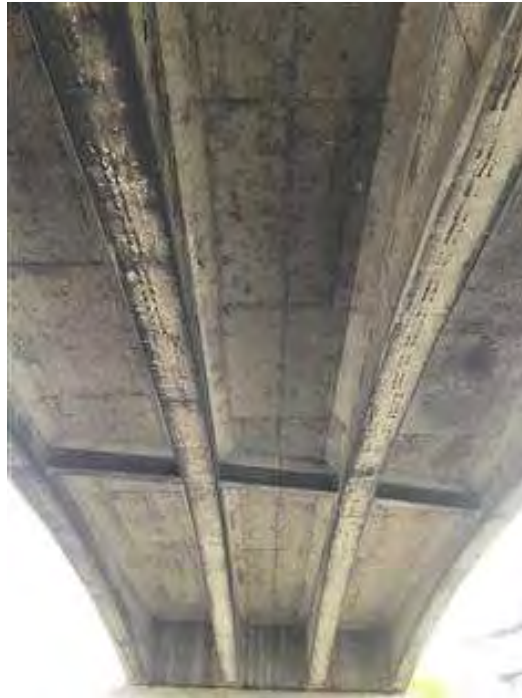
PHOTO 13 Condition Description Underside Span B facing East
