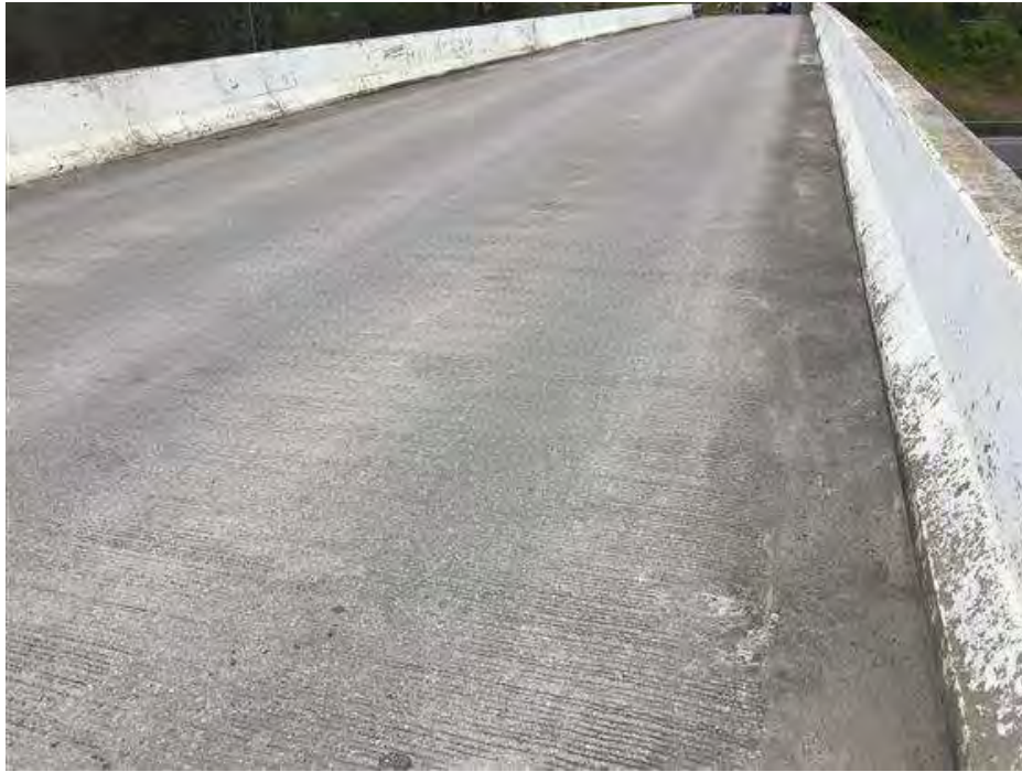
PHOTO 5 Condition Description Deck facing West
