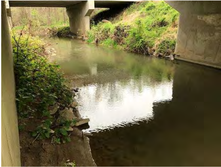
PHOTO 17 Condition Description US channel facing west through Span B.
