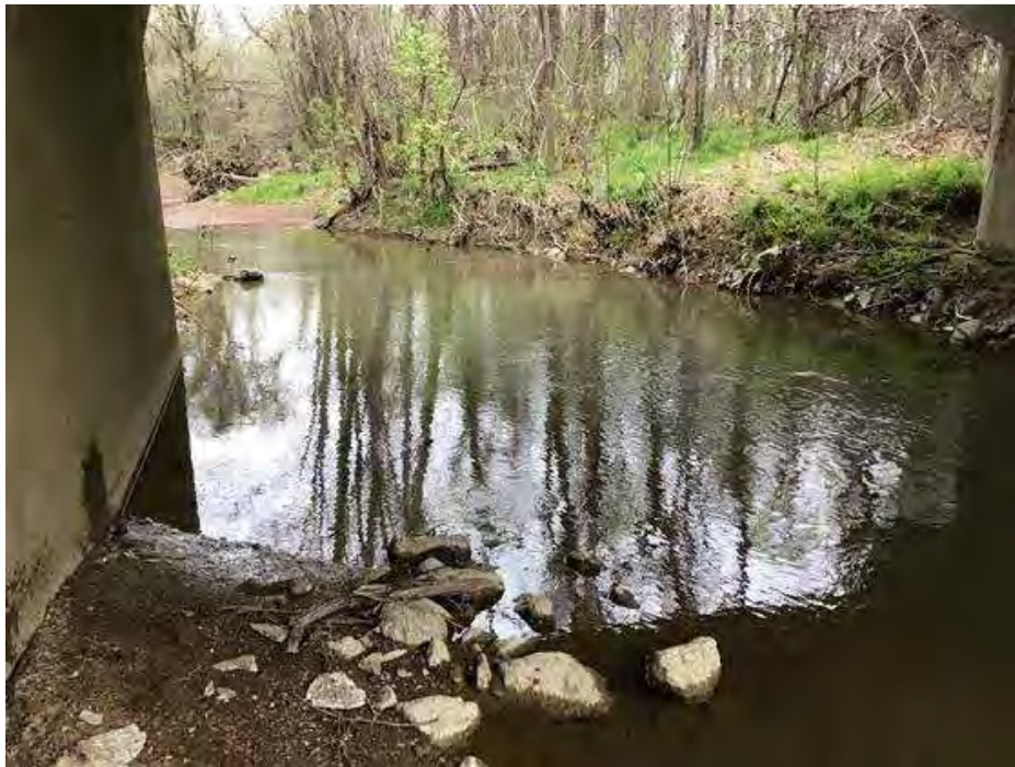
PHOTO 20 Condition Description US channel facing west through Span B.
