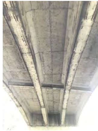
File Description Underside Span C facing West
