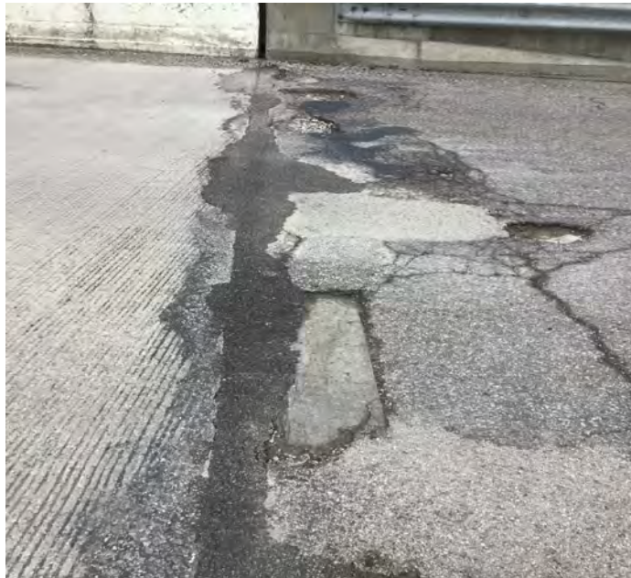
PHOTO 1 Description West Joint facing South
