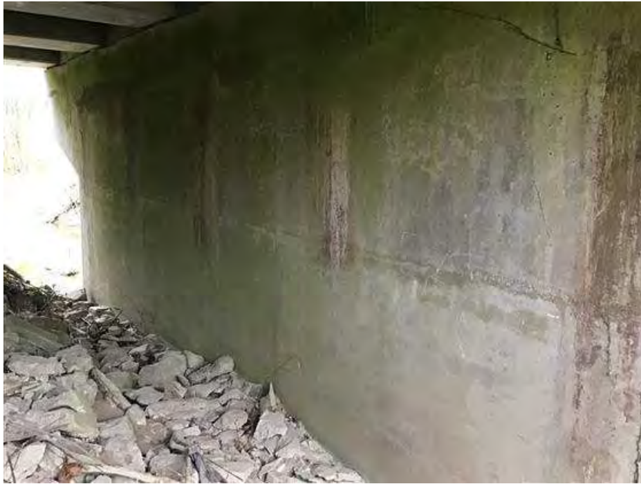
PHOTO 15 Condition Description Pier 2 south side.
