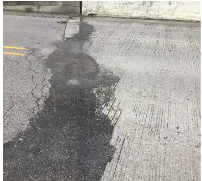
PHOTO 2 Description East Joint facing South
