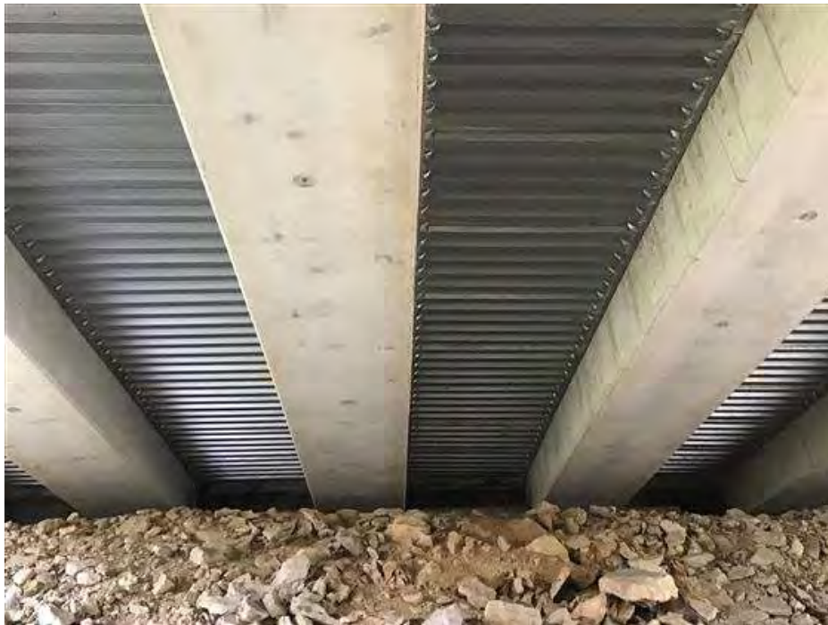
PHOTO 10 Condition Description Span C facing north.
