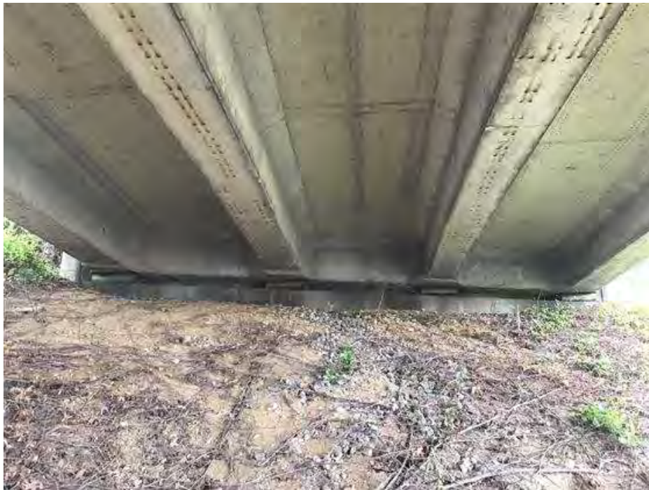
PHOTO 8 Condition Description Abutment #1 facing West
