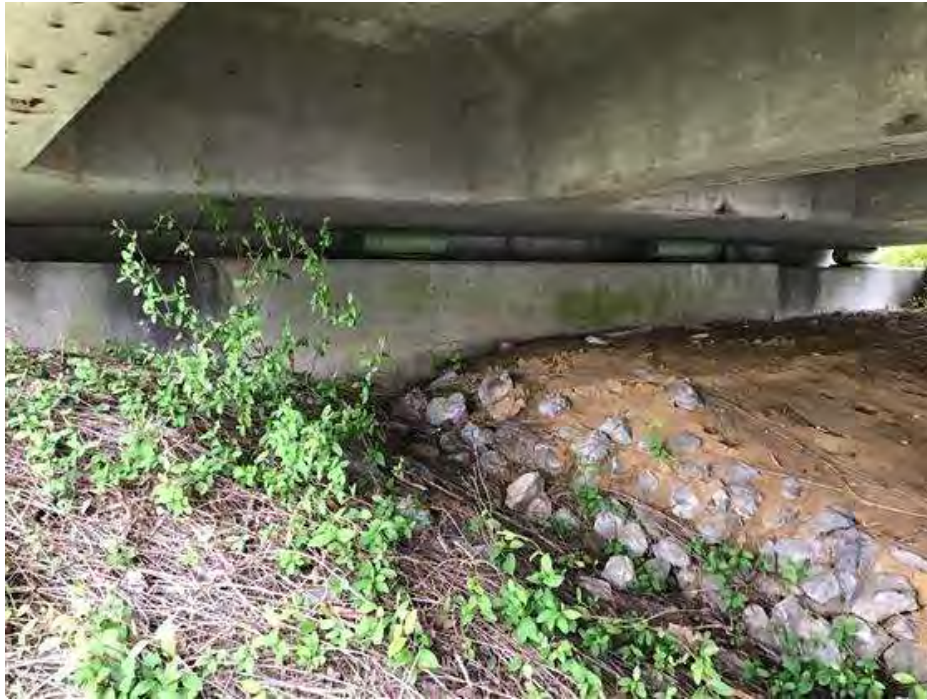
PHOTO 17 Condition Description East abutment.
