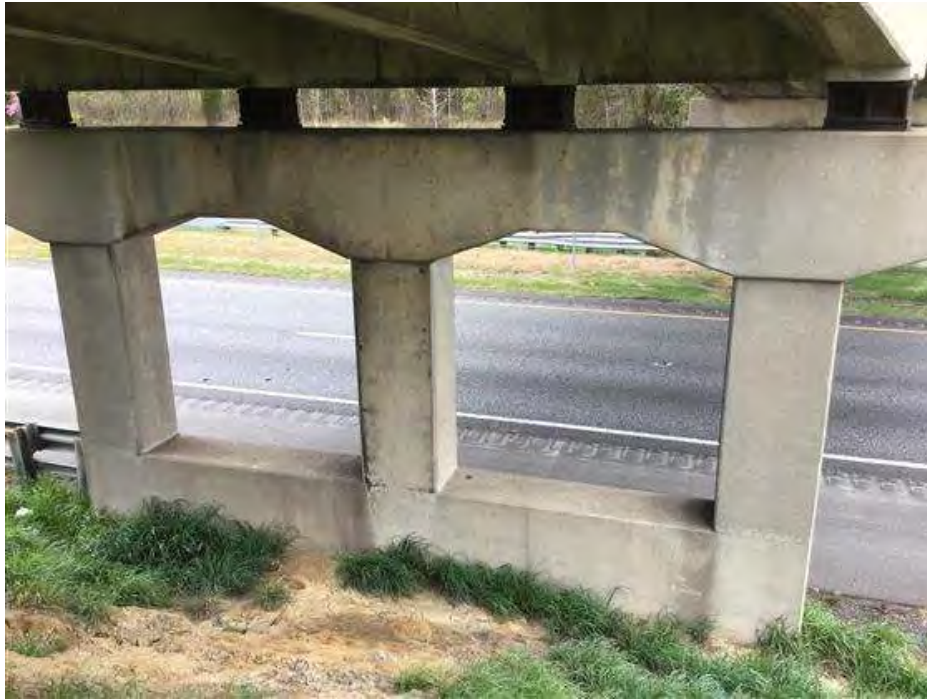
PHOTO 19 Condition Description Bent #4 facing West
