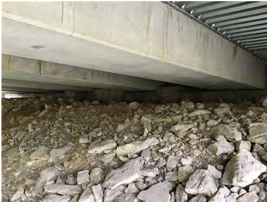
PHOTO 16 Condition Description North abutment.
