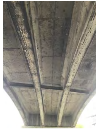
File Description Underside Span B facing East
