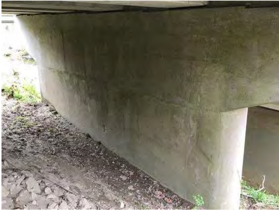
PHOTO 17 Condition Description Pier 3 north side.
