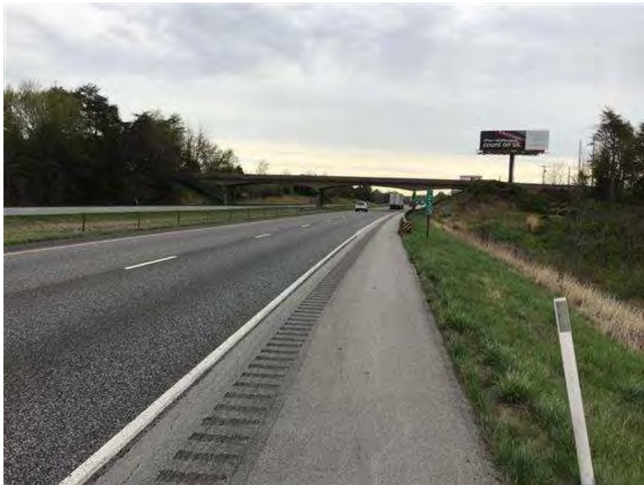
PHOTO 2 Elevation, Condition Description South side.
