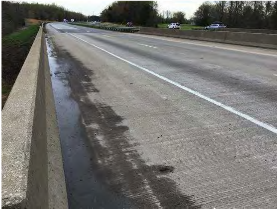
PHOTO 3 Condition Description Roadway north.
