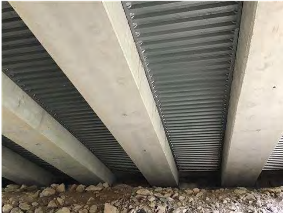
PHOTO 11 Condition Description Span C facing north.
