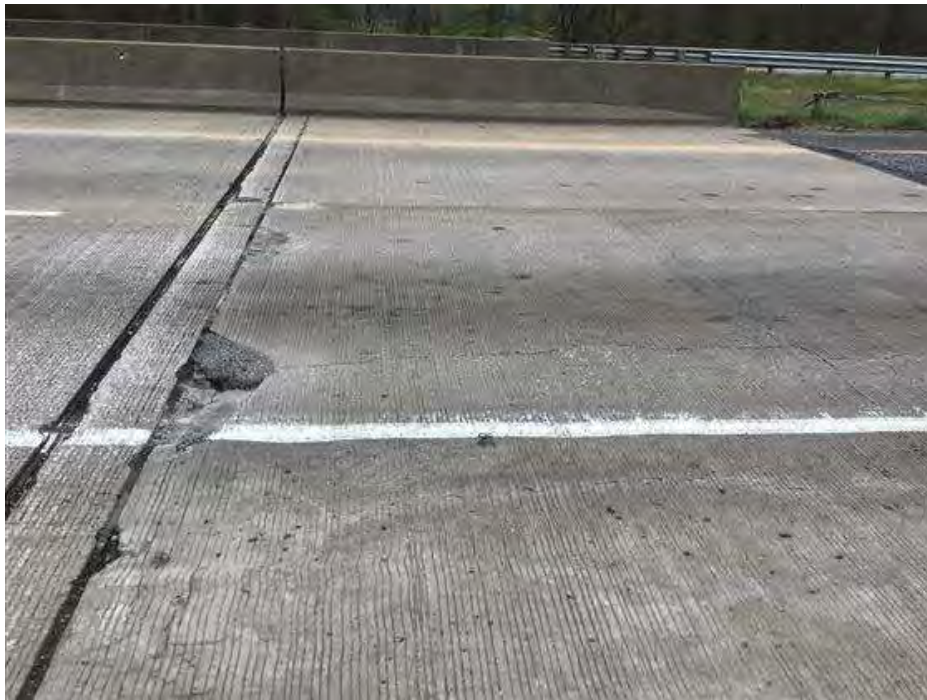
PHOTO 6 Condition Description South joint and approach slab.
