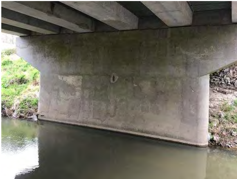
PHOTO 14 Condition Description Pier 3 south side.
