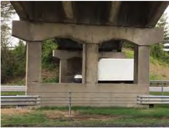
File Description Bent #3 facing West
