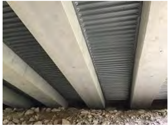
File Description Span C facing north.
