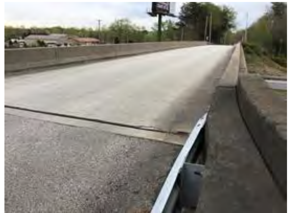
File Description Roadway east.
