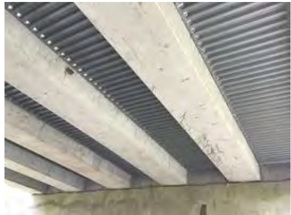
File Description Span B facing north.
