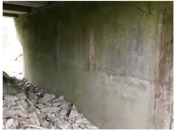
File Description Pier 2 south side.
