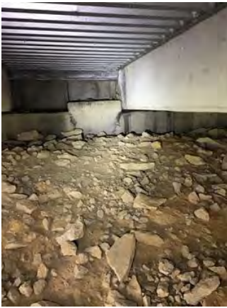
File Description Span A Beam 4.
