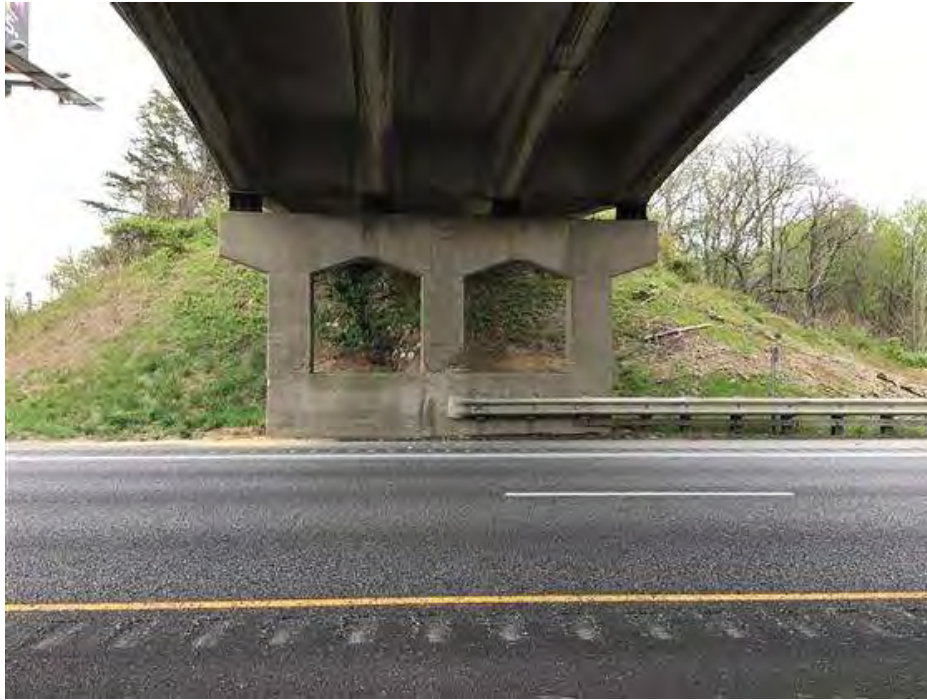
PHOTO 15 Condition Description Pier 4 facing east.
