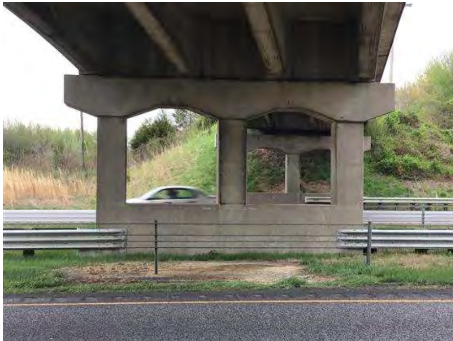
PHOTO 14 Condition Description Bent #3 facing East
