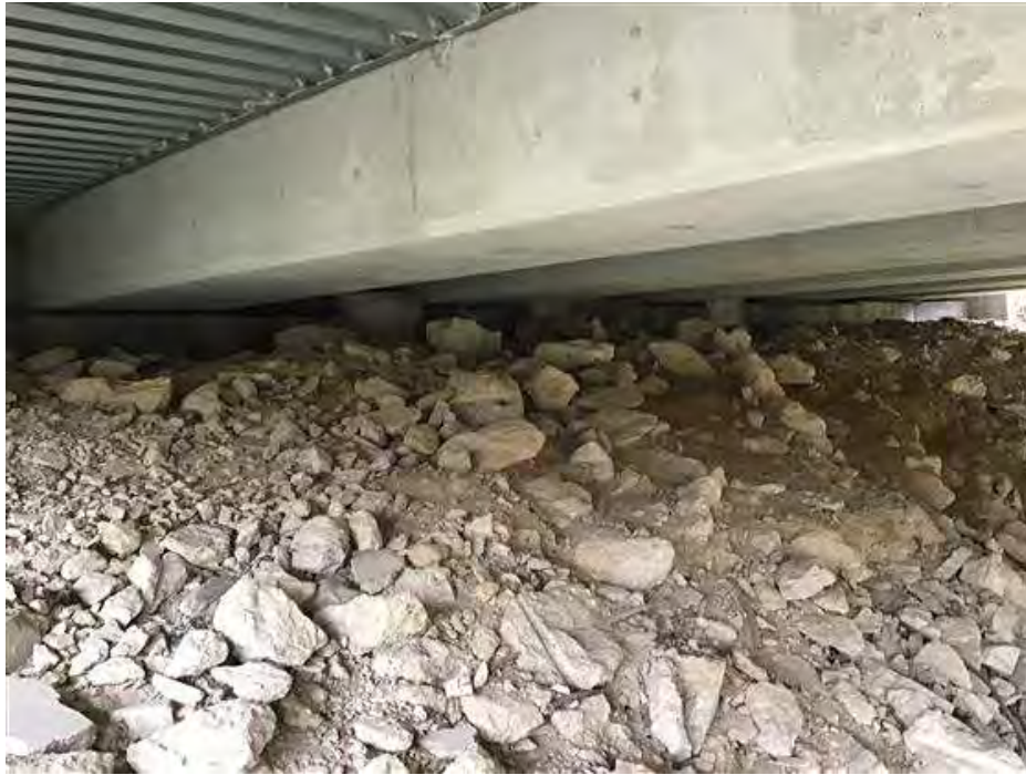
PHOTO 19 Condition Description North abutment.
