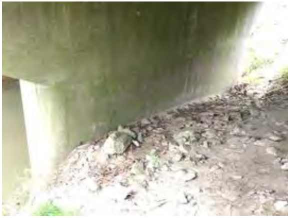
File Description Pier 3 north side.
