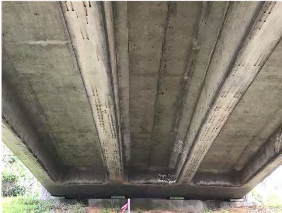
PHOTO 7 Condition Description Span A facing west.
