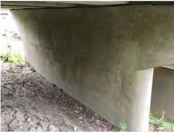
File Description Pier 3 north side.
