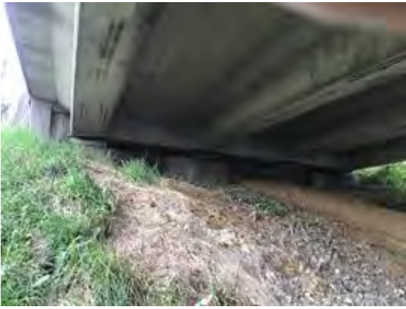
File Description Abutment #5 facing East File Type Category Condition
