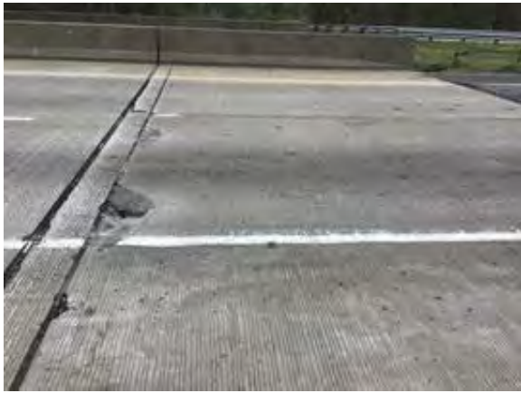
File Description South joint and approach slab.
