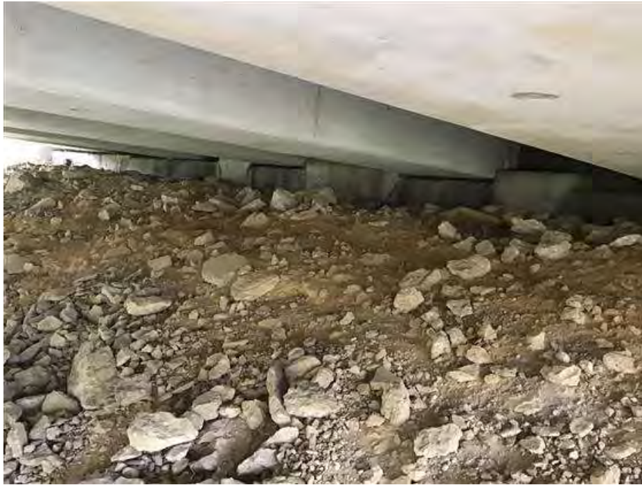
PHOTO 13 Condition Description South abutment.
