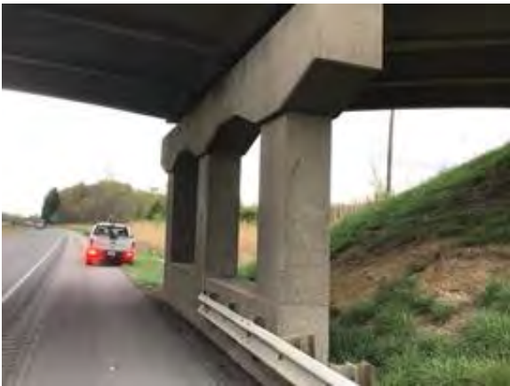
File Description Bent #4 facing Northeast
