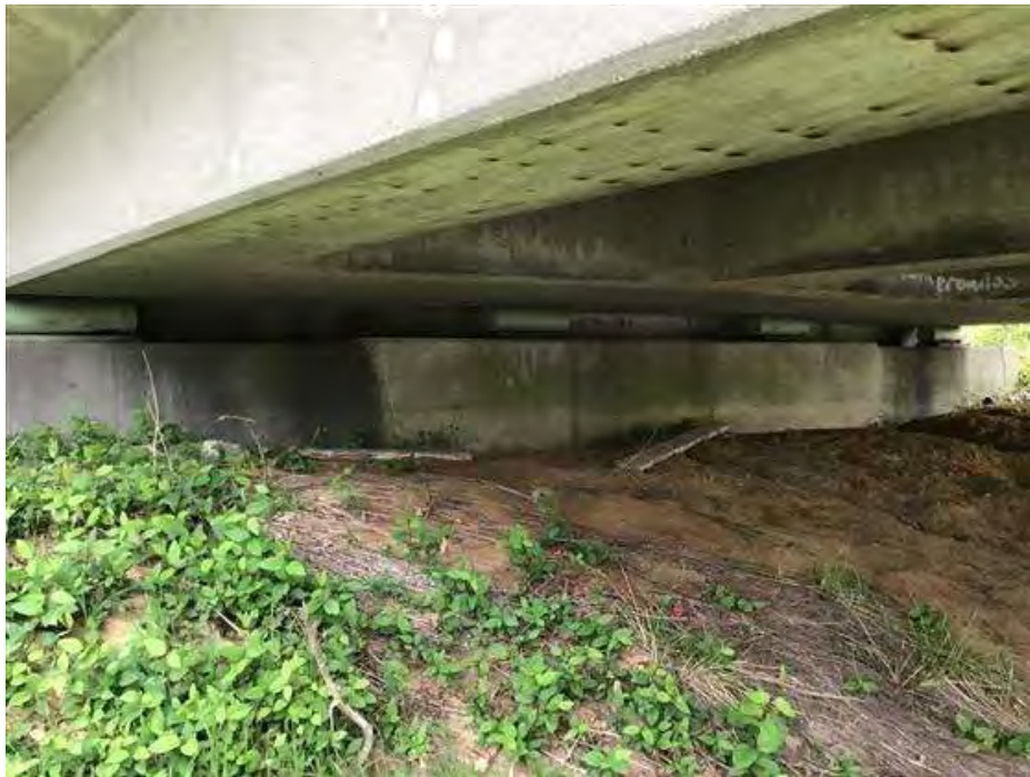
PHOTO 12 Condition Description West abutment.
