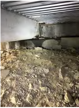
File Description Span A Beam 6. 3'x6"x6". File Type Category Condition, Other
