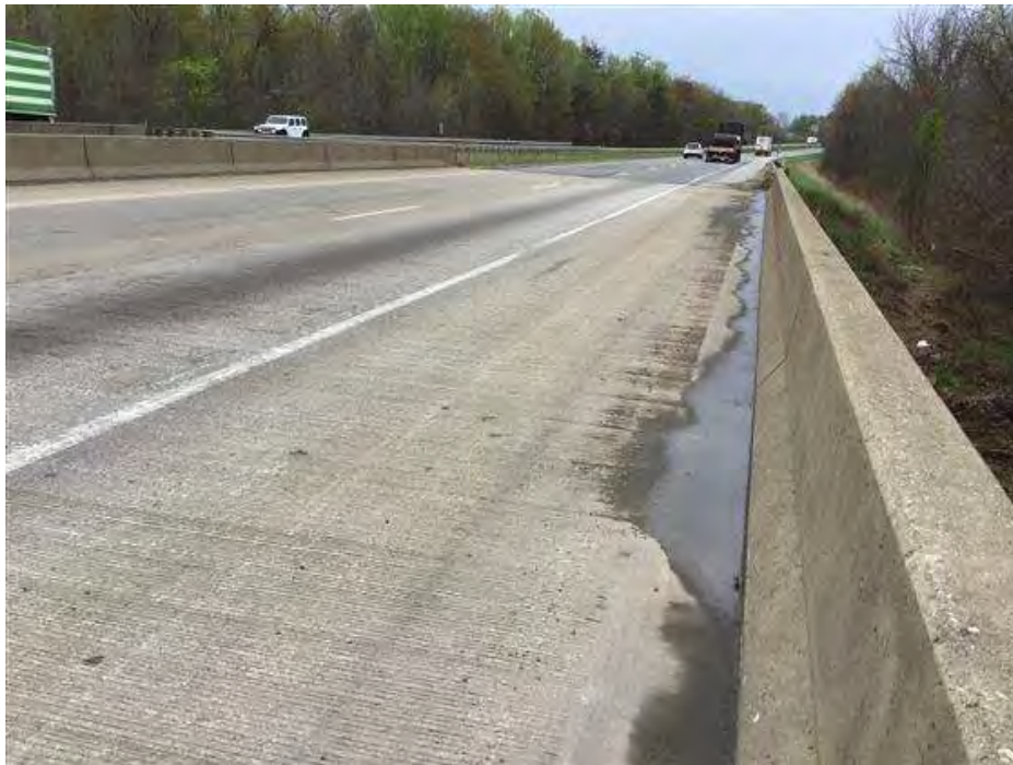
PHOTO 4 Condition Description Roadway south.
