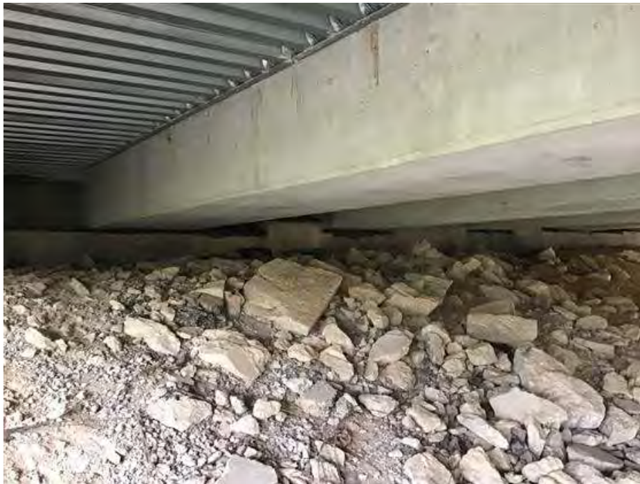
PHOTO 12 Condition Description South abutment.
