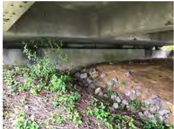
File Description East abutment.
