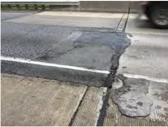
File Description South joint and approach slab.
