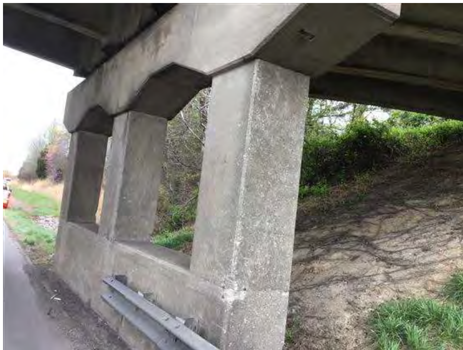
PHOTO 12 Condition Description Bent #2 facing Southwest
