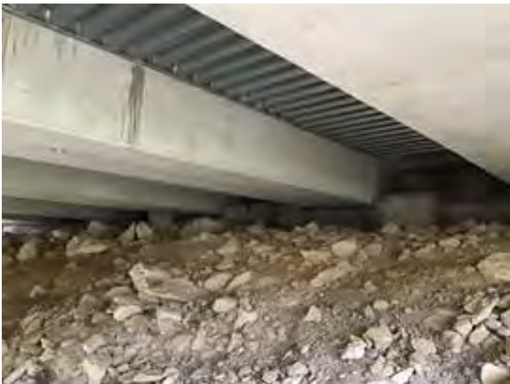
File Description North abutment.
