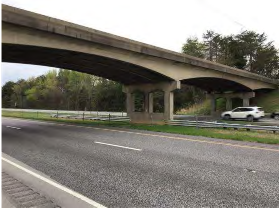
PHOTO 3 Elevation, Condition Description North side.
