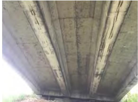
File Description Underside Span D facing East
