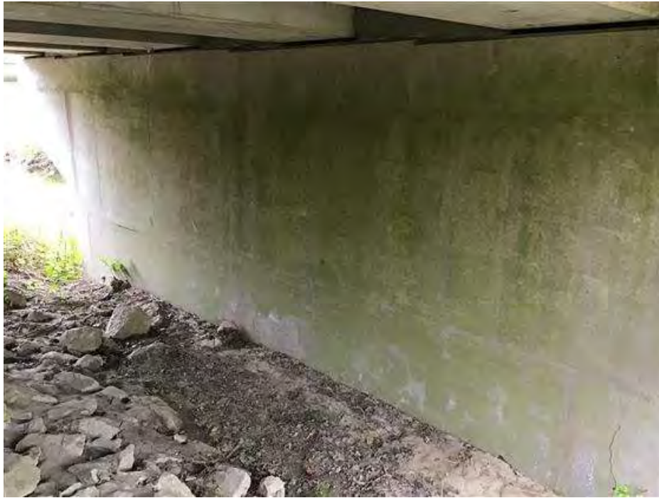
PHOTO 13 Condition Description Pier 2 south side.
