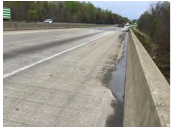
File Description Roadway south.
