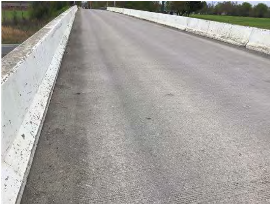
PHOTO 2 Condition Description Deck facing East
