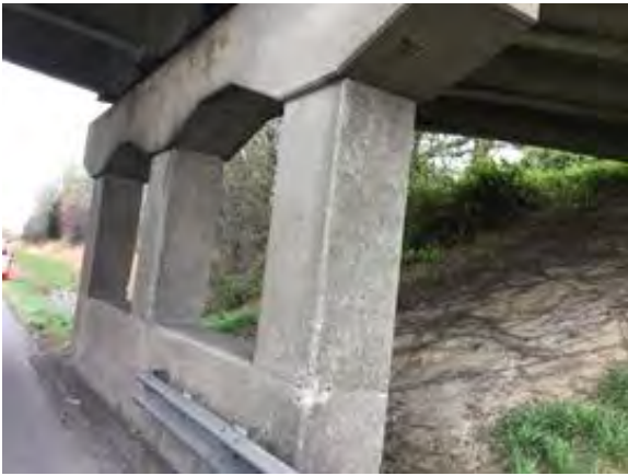
File Description Bent #2 facing Southwest
