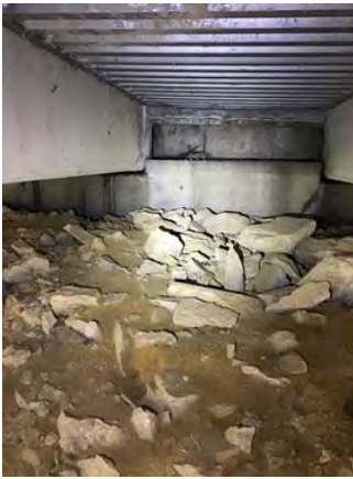
File Description Span A Beam 4.
