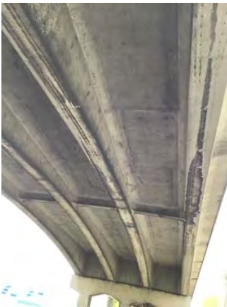
File Description Span B facing east. File Type Category Condition
