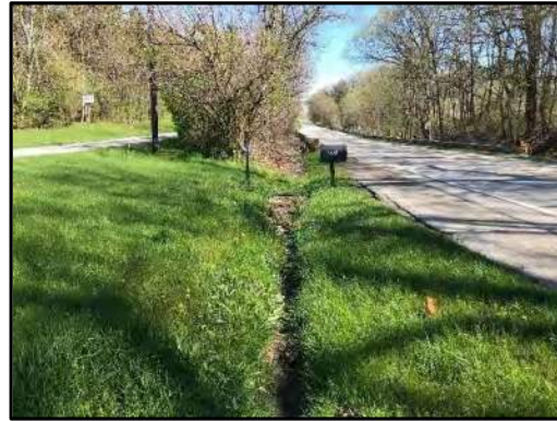
Photo 8. North of Robbins Rd., looking north along west side of SR 149
