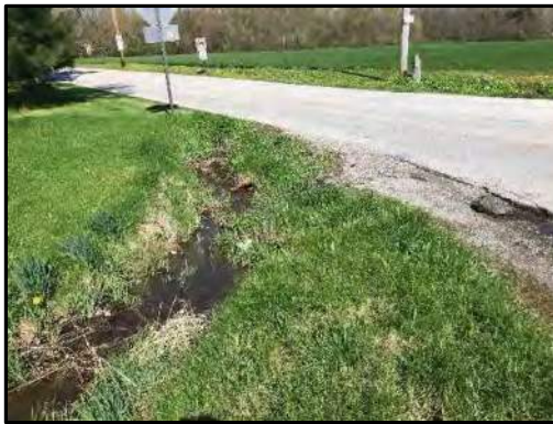
Photo 9. Southwest corner of intersection- Looking northwest- along Robbins.
