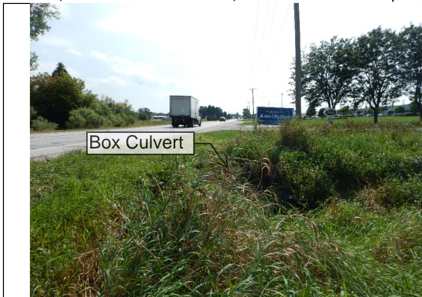
Photo 9: Facing south at Preston Miles Ditch box culvert and SR 15
