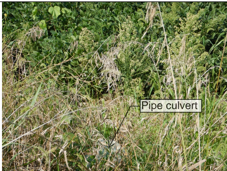
Photo 19: Facing north at culvert
