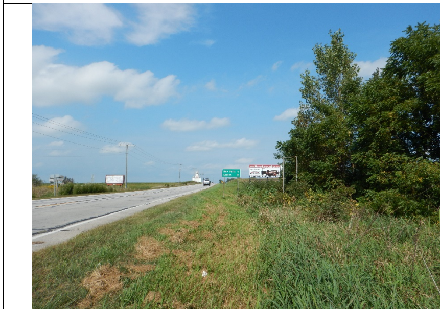
Photo 11: Facing north at east side of SR 15 and Wetland 2
