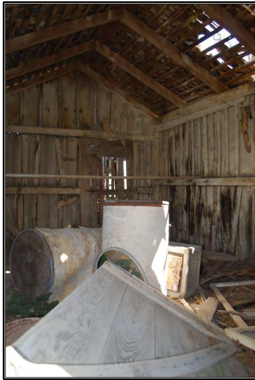
Figure B-22. Interior of shed, facing north (Resource D).
