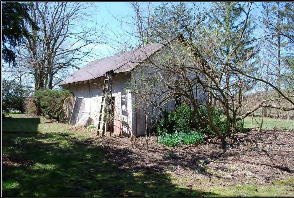
Figure B-23. East and south elevations, facing southwest (Resource E).
