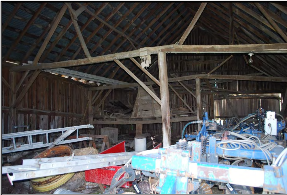
Figure B-14. View of interior of barn (Resource A), facing southwest.
