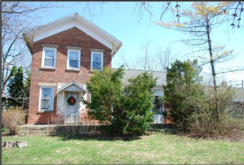
Figure 8. View of facade (west) elevation.
