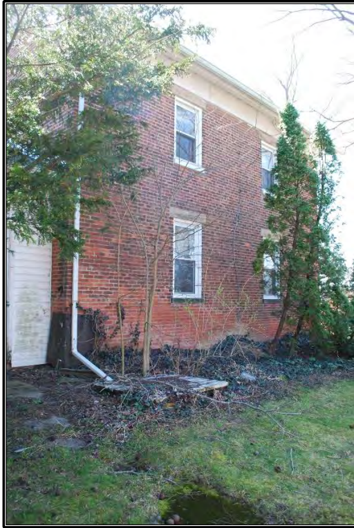
Figure B-11. North elevation, facing southwest.
