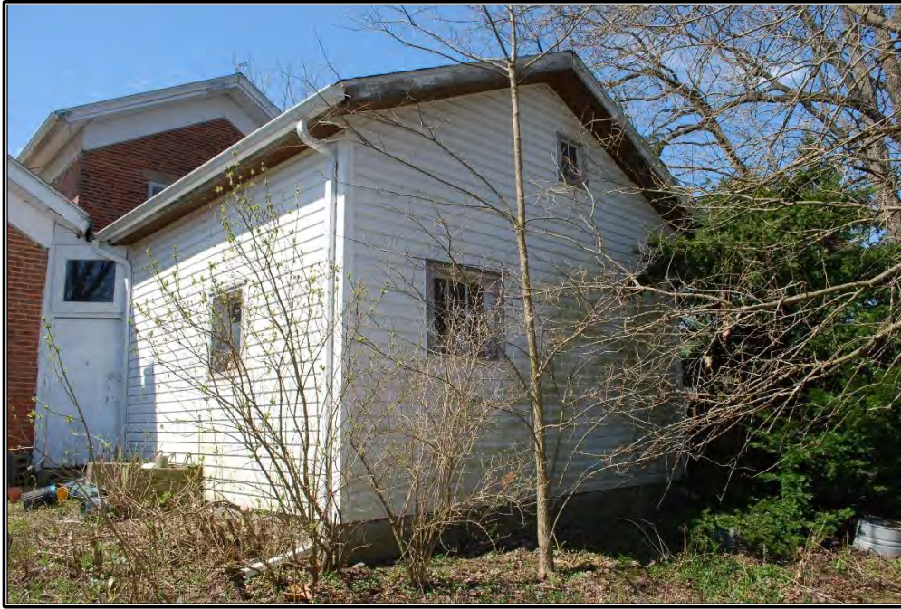
Figure B-9. Rear (east) elevation of frame addition, facing southwest.
