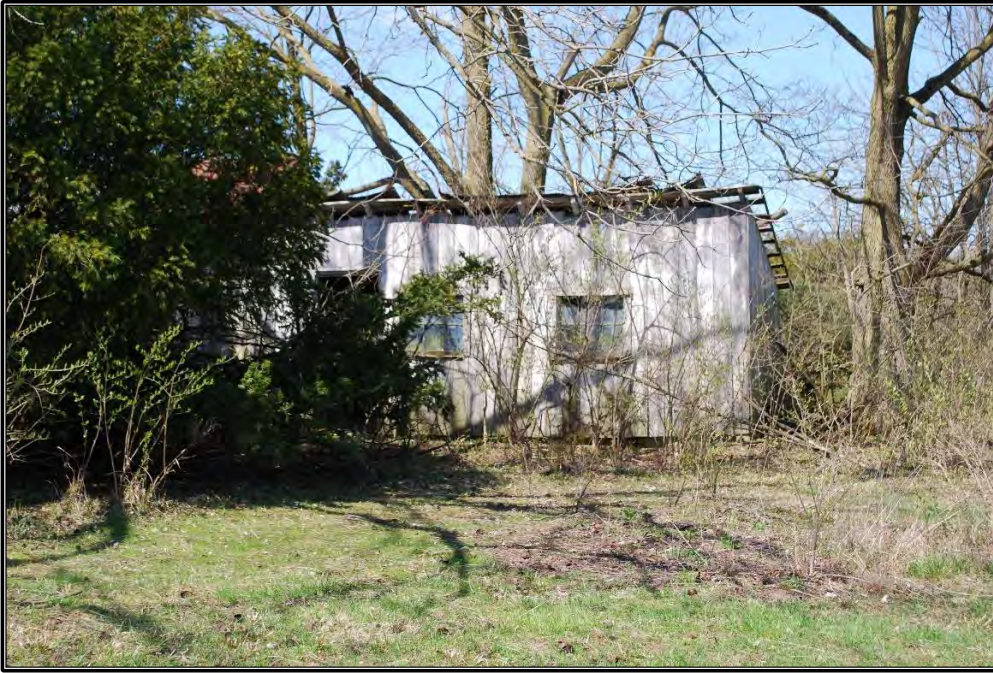
Figure B-21. East elevation, facing northwest (Resource D).
