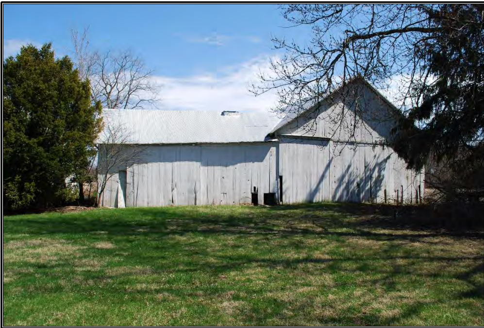
Figure B-16. West elevation, facing northeast (Resource B).
