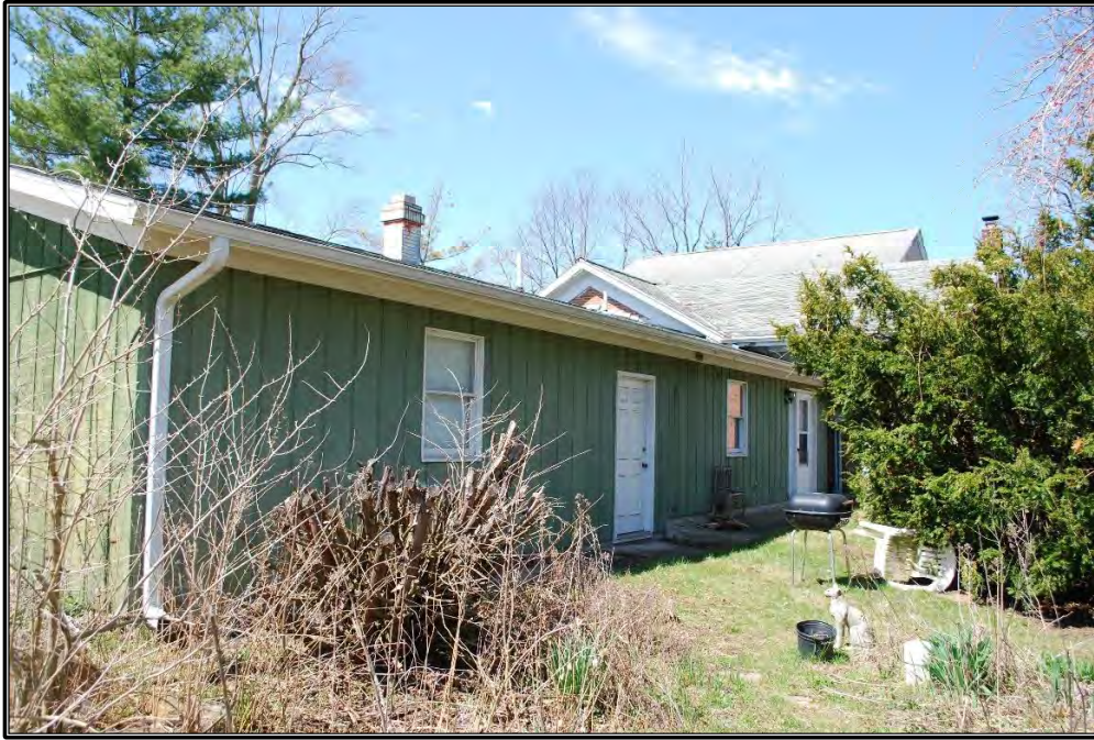
Figure B-7. Rear (east) elevation, facing southwest.
