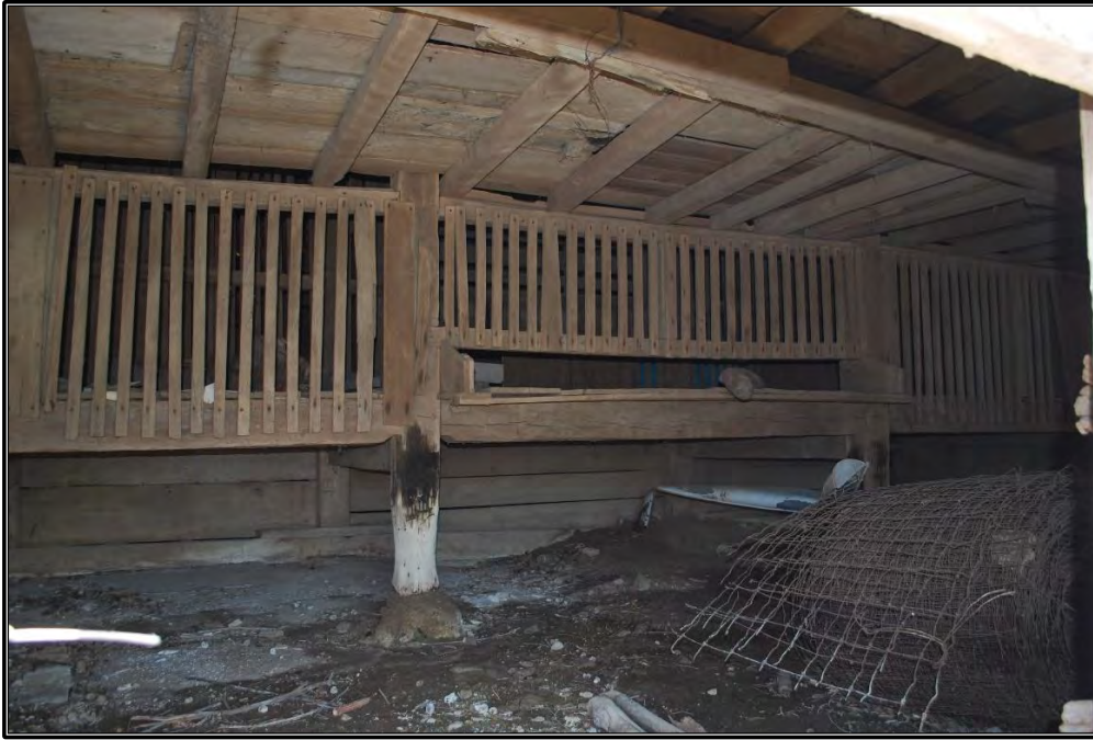
Figure B-17. View of interior, facing northwest (Resource B).
