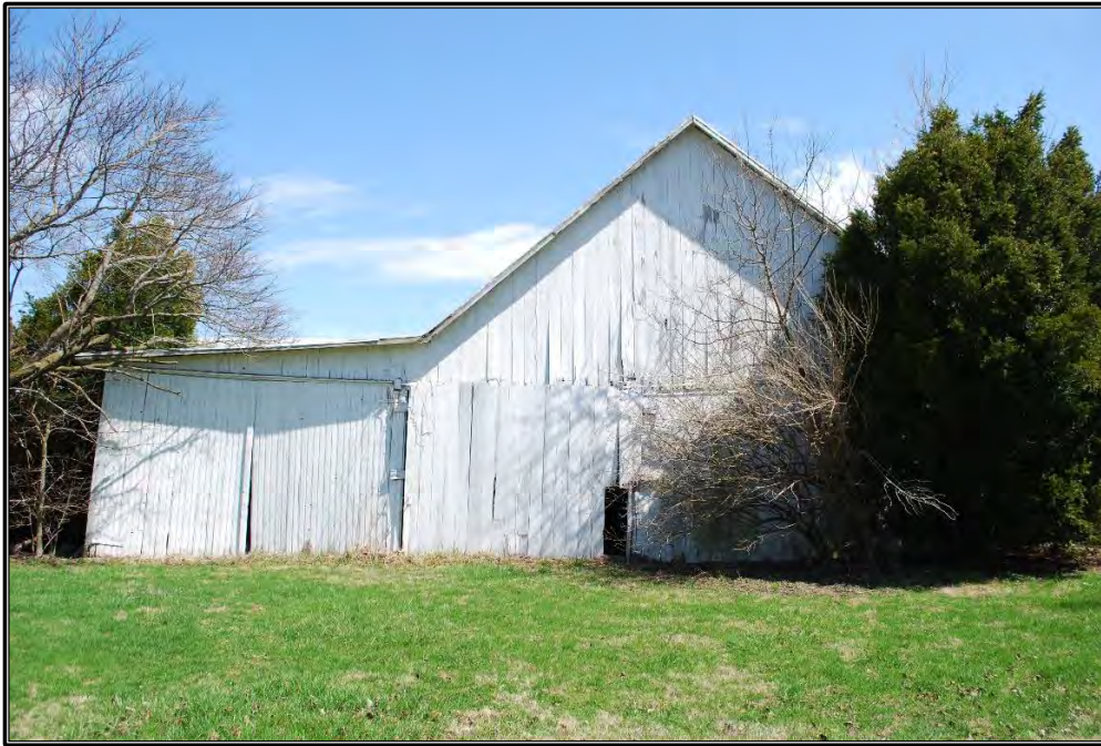
Figure B-12. West elevation, facing northeast (Resource A).
