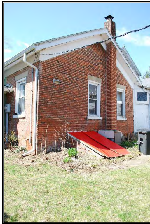
Figure B-8. Rear (east) elevation, facing southwest.
