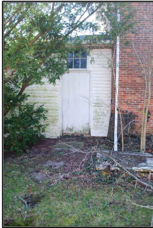
Figure B-10. North elevation of frame addition, facing southeast.
