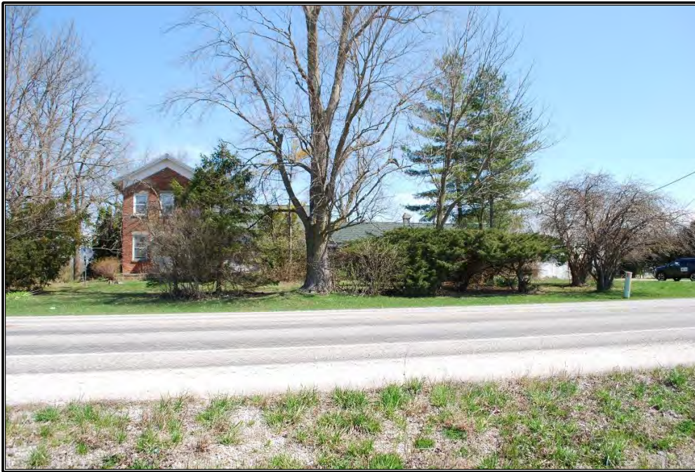
Figure B-3. Overview of the Abram T. Studabaker Farm (IHSSI No. 179-361-20049), facing northeast.
