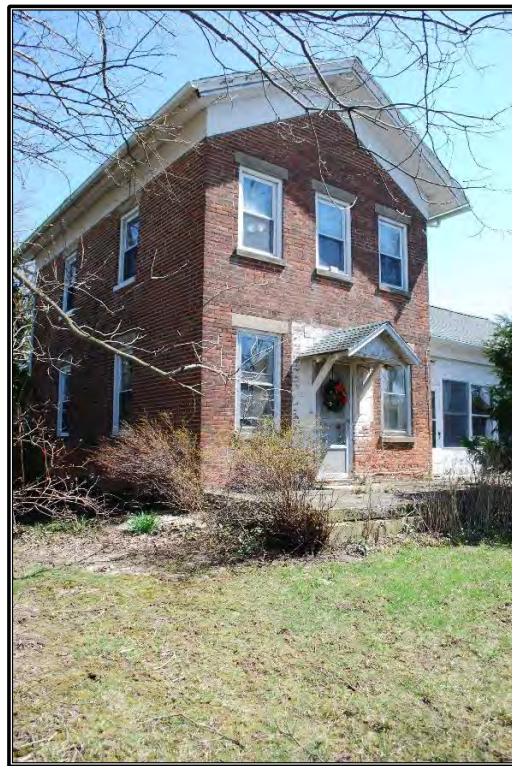
Figure B-4. Facade (west) elevation and north elevation, facing east.
