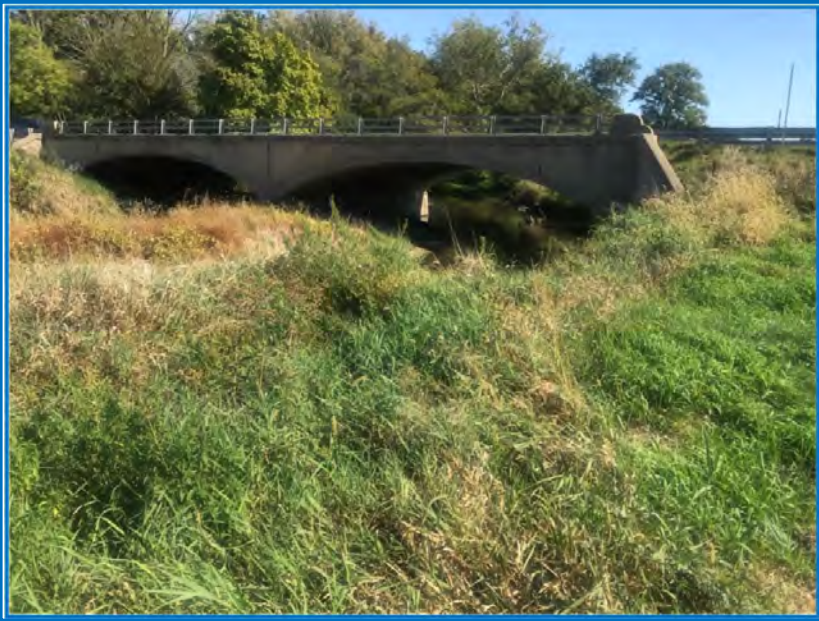
Photo 1 – View of the US 41 bridge over Coal Creek facing east (10/8/2019).
