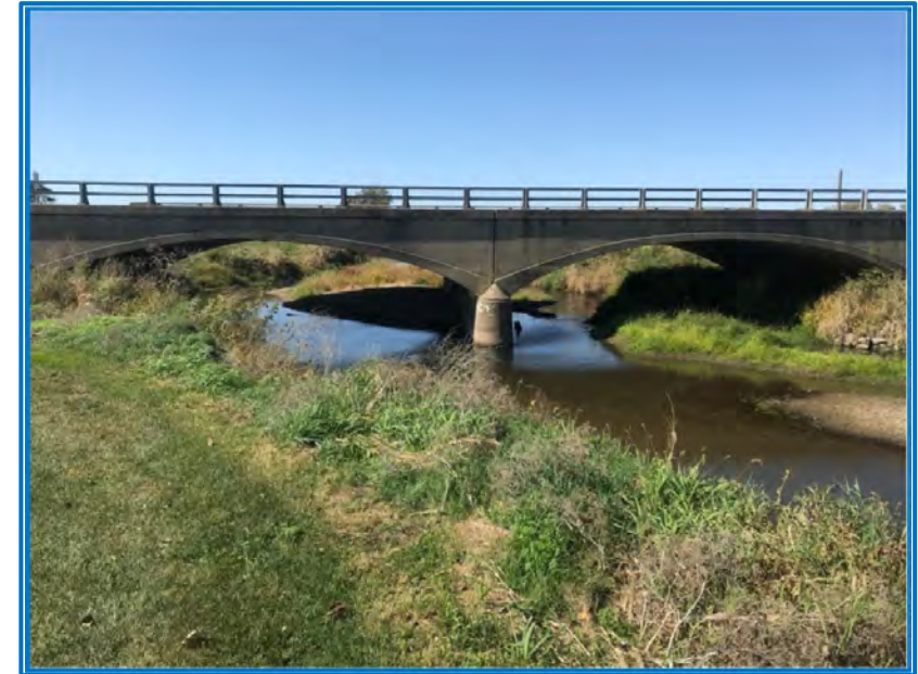
Photo 4 – View of the US 41 bridge over Coal Creek facing west (10/8/2019).
