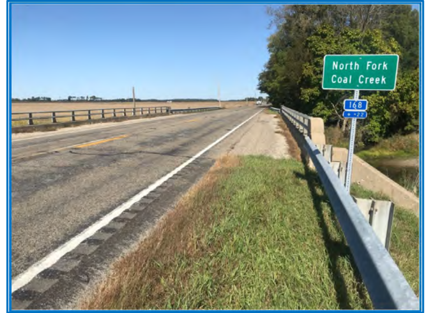
Photo 2 – View of the US 41 bridge over Coal Creek facing north (10/8/2019).
