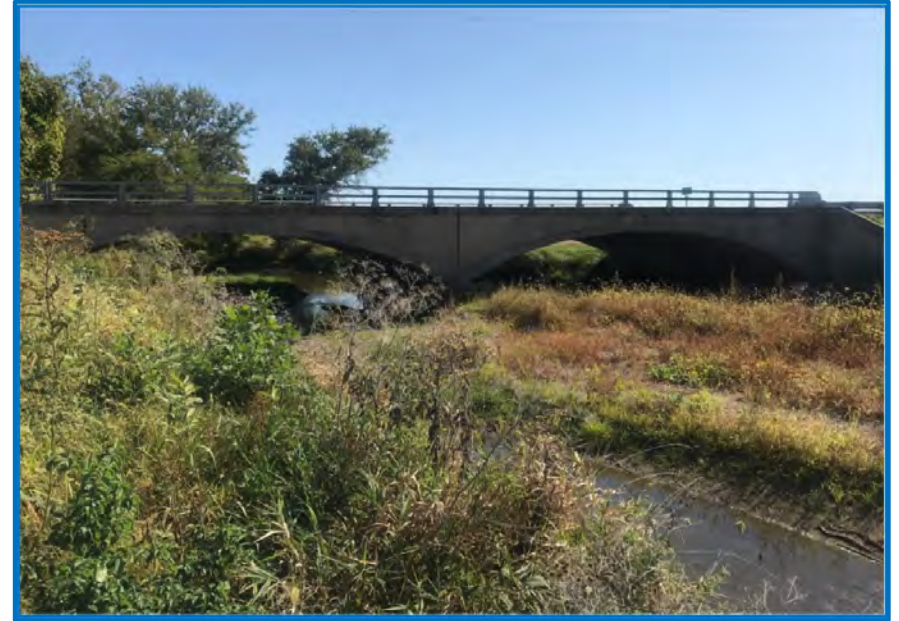
Photo 6 – View of the US 41 bridge over Coal Creek facing southeast (10/8/2019).
