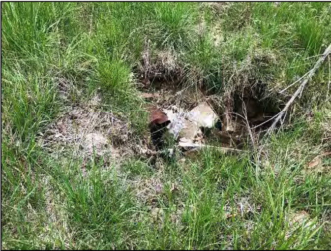
Photo 5. Inlet of Structure 2, viewing southeast, 5/13/2022
