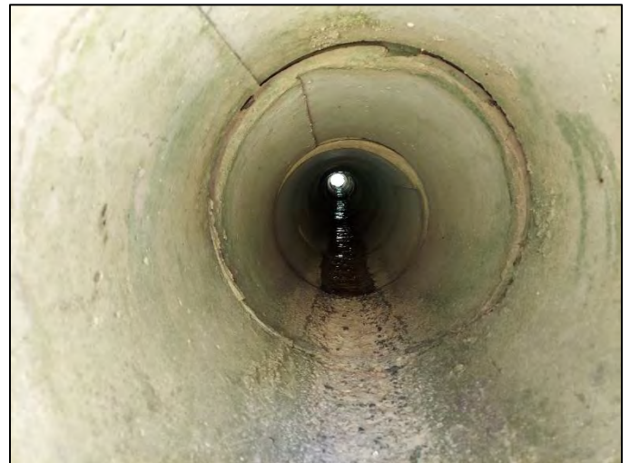
Photo 12. Looking through CLV-67652 at outlet, viewing south, 5/13/2022
