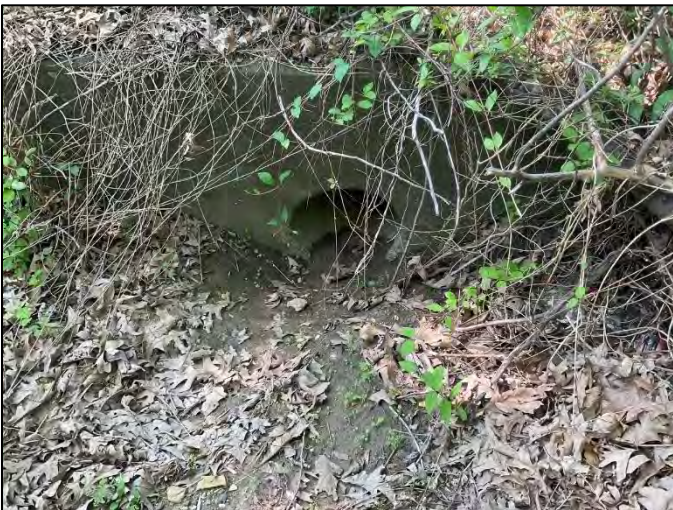
Photo 3. Outlet of CLV-67648, viewing south, 5/13/2022
