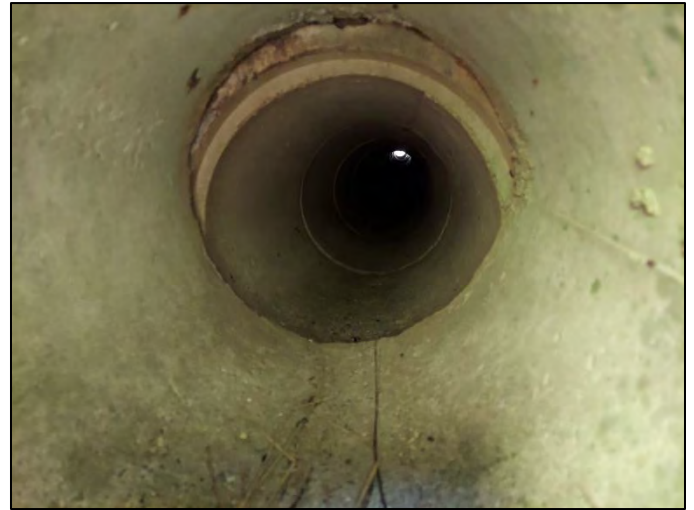
Photo 2. Looking through CLV-67648 at inlet, viewing north, 5/13/2022
