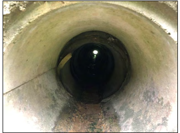
Photo 10. Looking through CLV-67652 at inlet, viewing north, 5/13/2022
