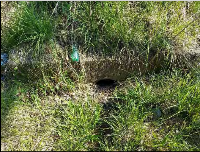
Photo 1. Inlet of CLV-67648, viewing north, 5/13/2022
