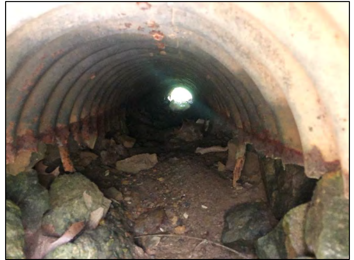
Photo 6. Looking through Structure 2 at inlet, viewing east, 5/13/2022
