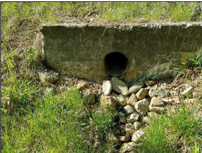
Photo 11. Outlet of CLV-67652, viewing south, 5/13/2022
