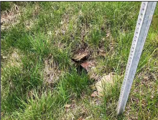
Photo 7. Outlet of Structure 2, viewing southwest, 5/13/2022
