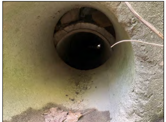
Photo 4. Looking through CLV-67648 at outlet, viewing south, 5/13/2022
