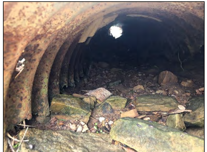
Photo 8. Looking through Structure 2 at outlet, viewing west, 5/13/2022
