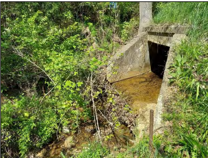
Photo 15. Outlet of CV 445-28-000.52, viewing west, 5/13/2022
