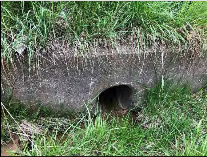
Photo 9. Inlet of CLV-67652, viewing north, 5/13/2022
