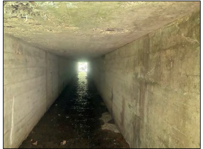
Photo 14. Looking through CV 455-28-000.52 at inlet, viewing southeast, 5/13/2022
