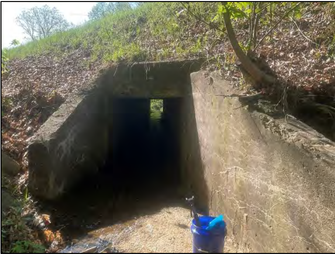
Photo 13. Inlet of CV 455-28-000.52, viewing southeast, 5/13/2022
