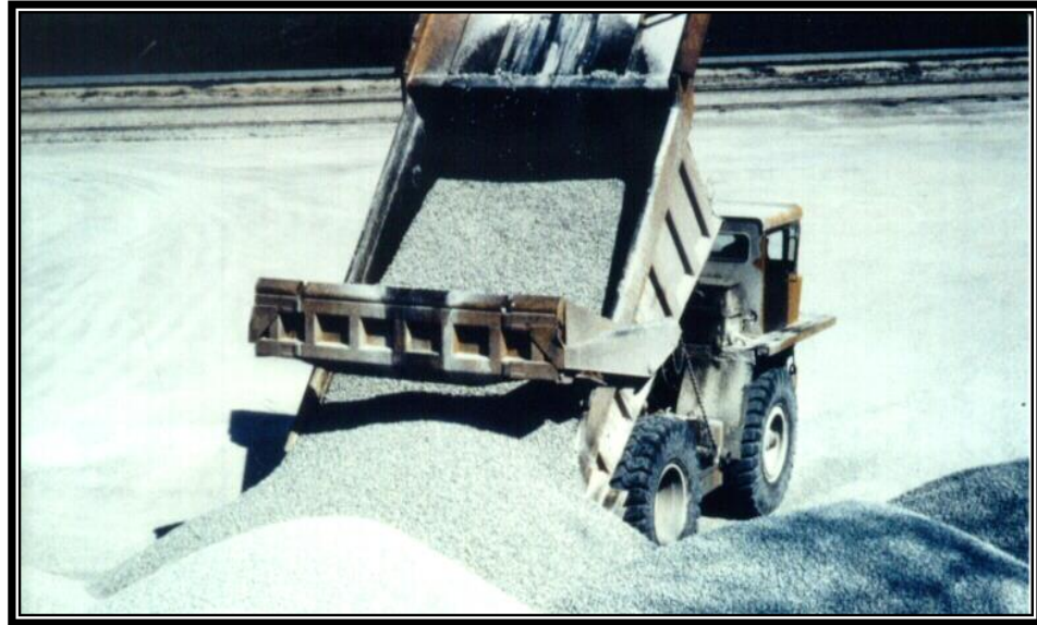
Figure 5-29. Low Profile Truck Stockpiles
