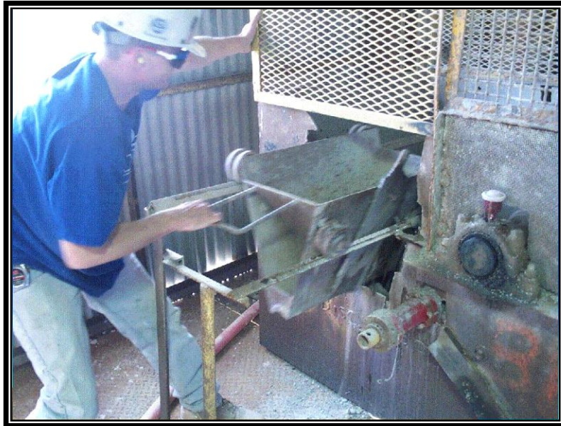
Figure 9-1. Discharge Sampling of Belt
