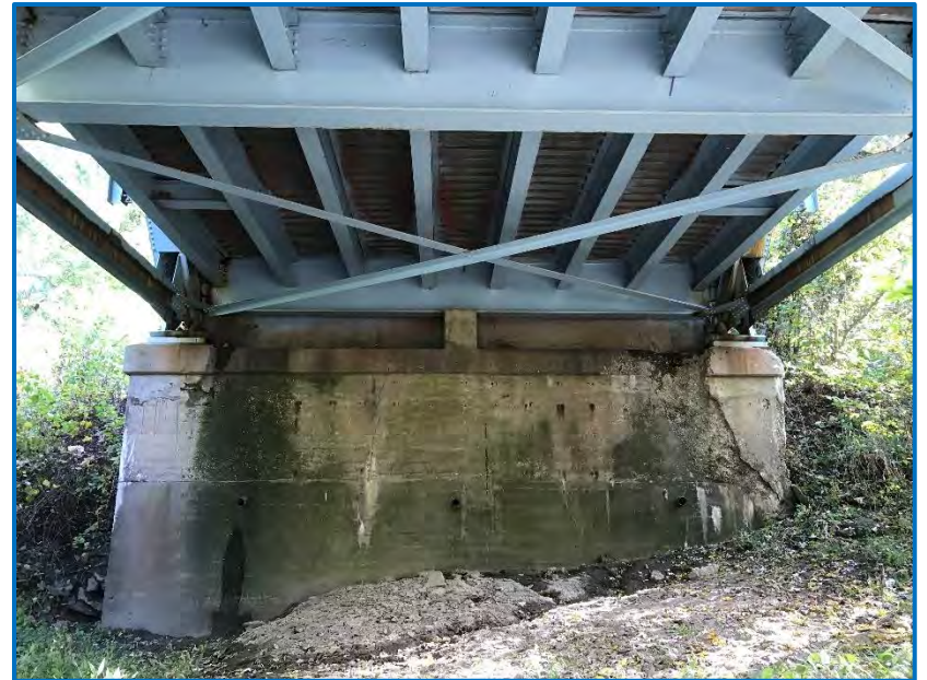
Photo 4 – View of the SR 163 bridge abutment facing east (10/23/19).
