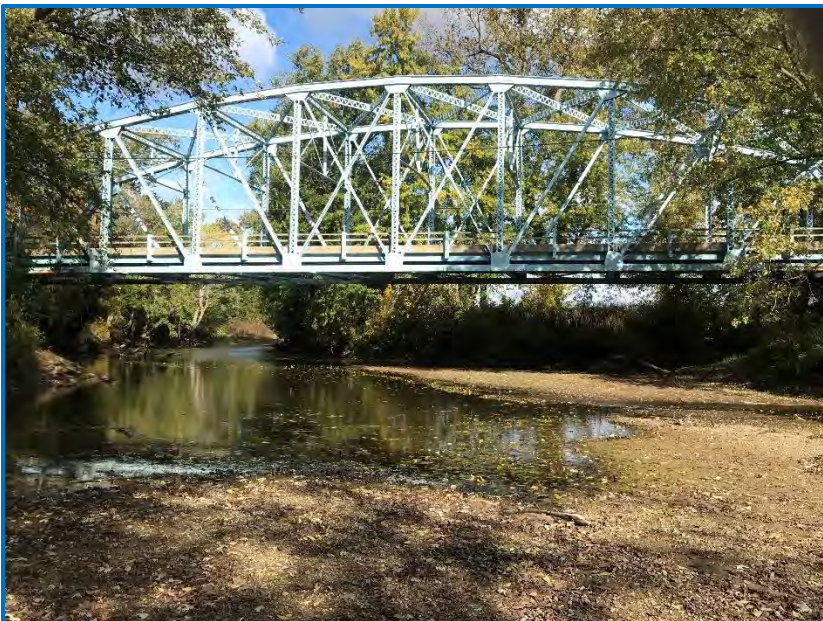
Photo 3 – View of the SR 163 bridge over Brouilletts Creek facing northwest (10/22/2019).
