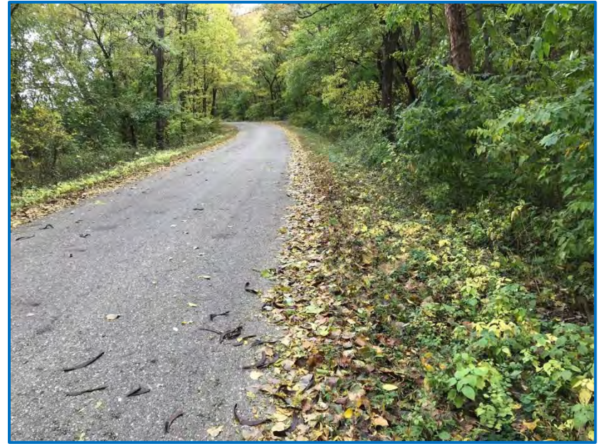
Photo 6 – View of CR 170 West facing north (10/22/2019).
