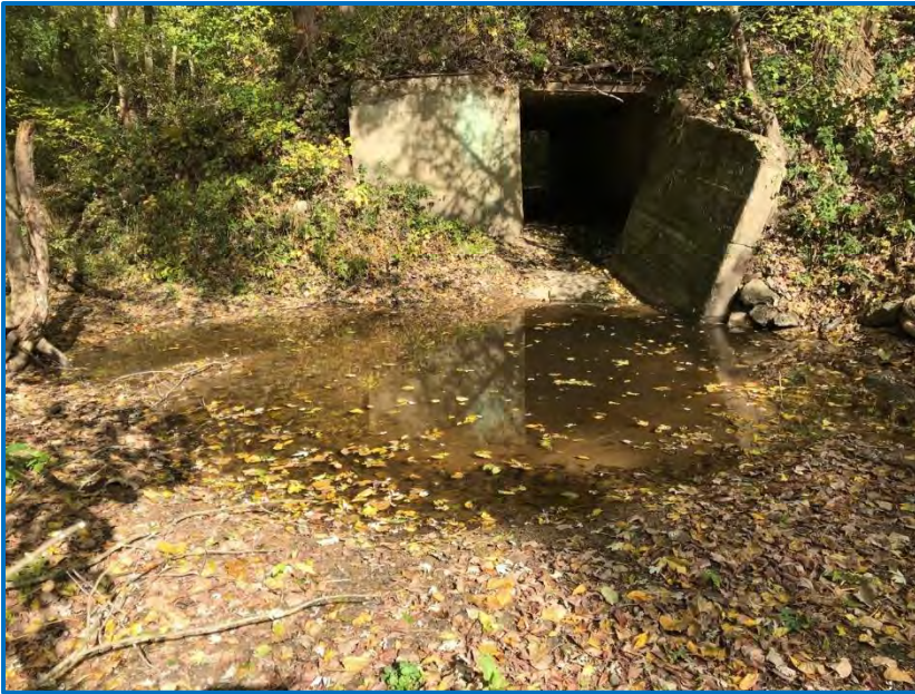
Photo 1 – View of the culvert outlet under CR 170 W facing east (10/23/19).
