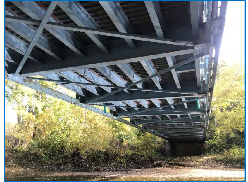
Photo 2 – View of the SR 163 bridge over Brouilletts Creek northeast (10/23/19).
