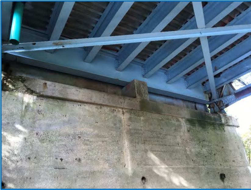
Photo 1 – View of the SR 163 bridge abutment facing northwest (10/23/19).
