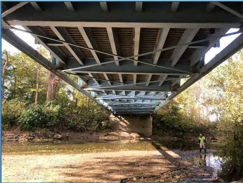
Photo 3 – View of the SR 163 bridge over Brouilletts Creek facing west (10/23/19).
