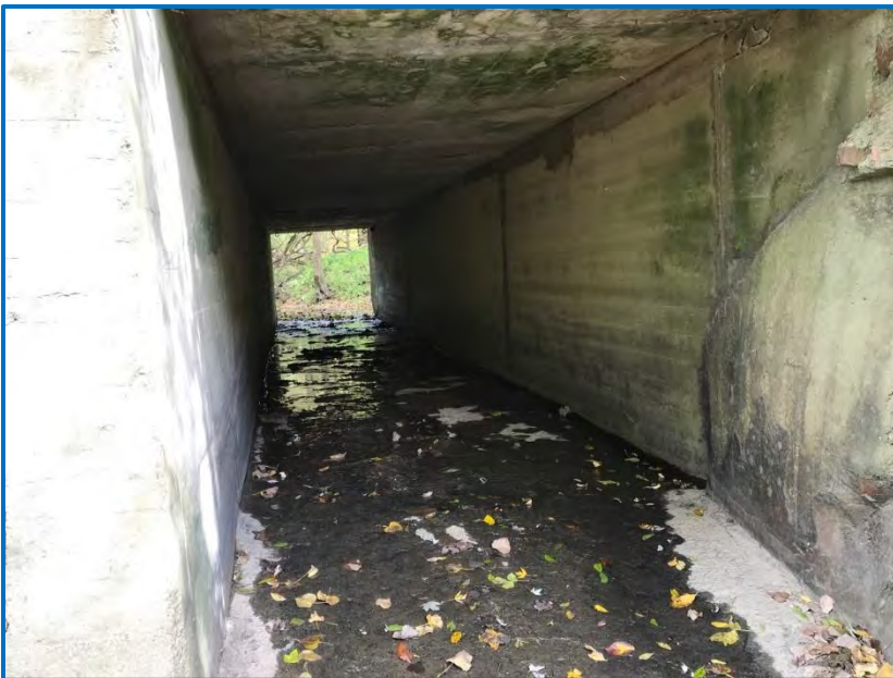
Photo 3 – View inside the culvert under CR 170 W facing east (10/23/19).
