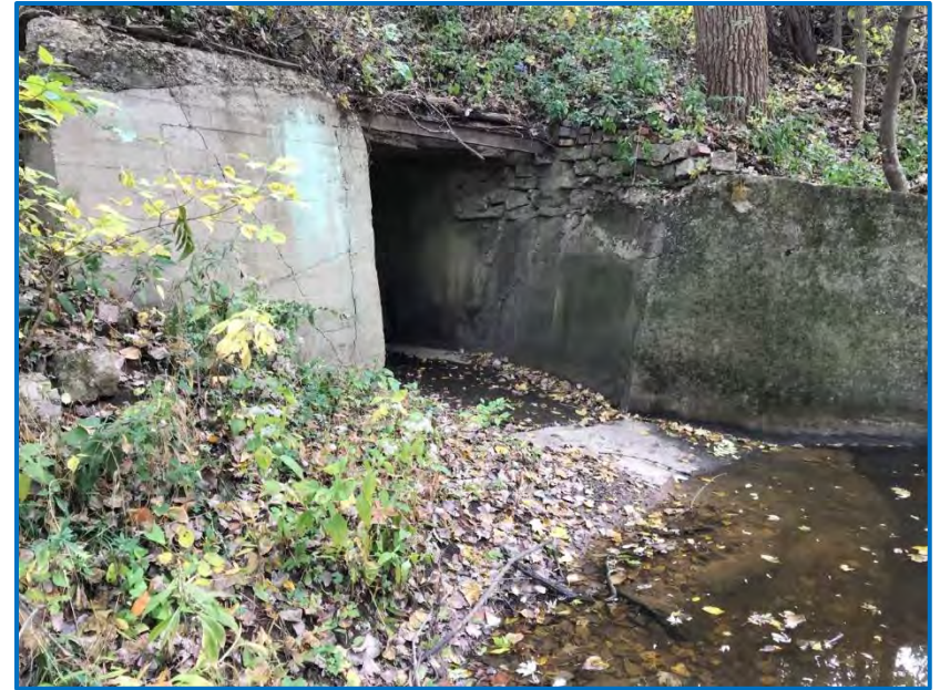
Photo 2 – View of the culvert outlet under CR 170 W facing southeast (10/23/19).
