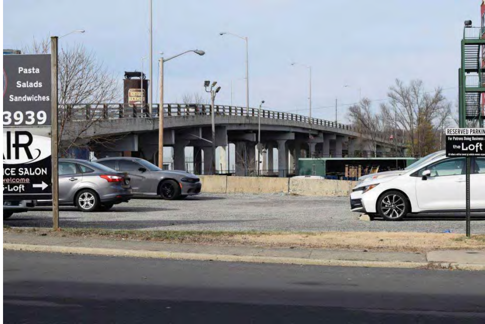
Photograph 45. View of the US 27 over NSRR and local streets bridge from North D Street, facing northwest.
