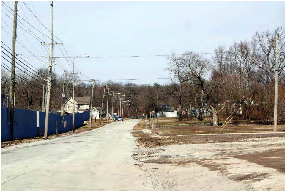
Photograph 24. View of North 8 th Street from North F Street, facing north.
