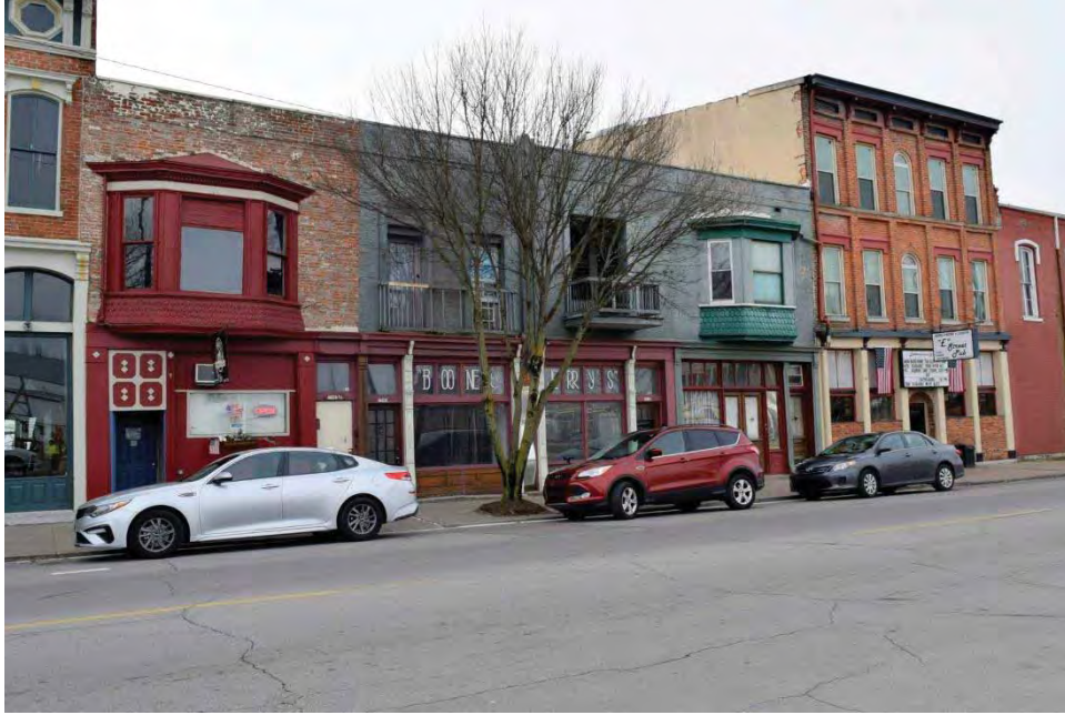
Photograph 39. View of the 800 block of North E Street in the Richmond Railroad Station Historic District, facing southwest.
