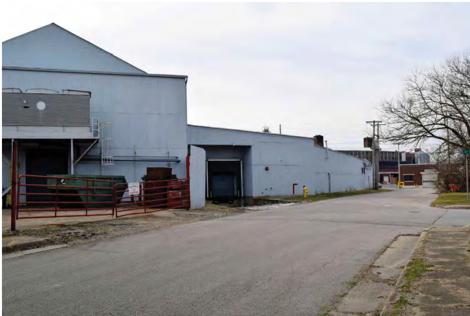
Photograph 28. View of North F Street just west of the US 27 bridge, facing west.
