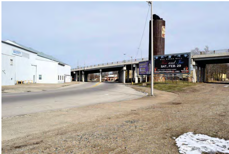
Photograph 32. View of Fort Wayne Avenue from North 8 th Street, showing the US 27 over Norfolk Southern Railroad (NSRR) and local streets bridge, facing northeast.
