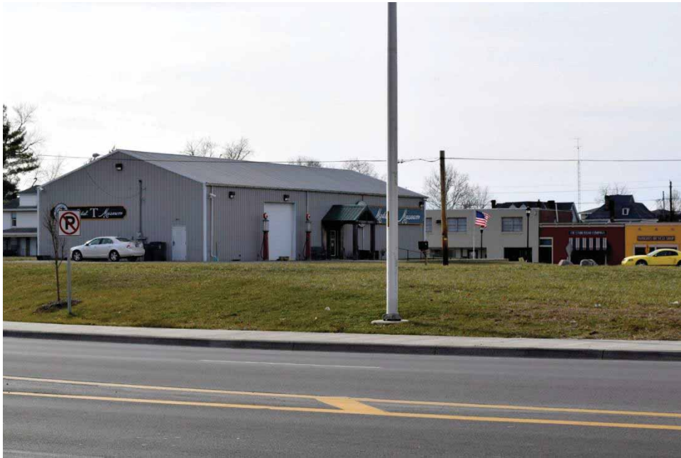
Photograph 42. View of the Model T Museum at 309 North 8 th Street, facing southwest.
