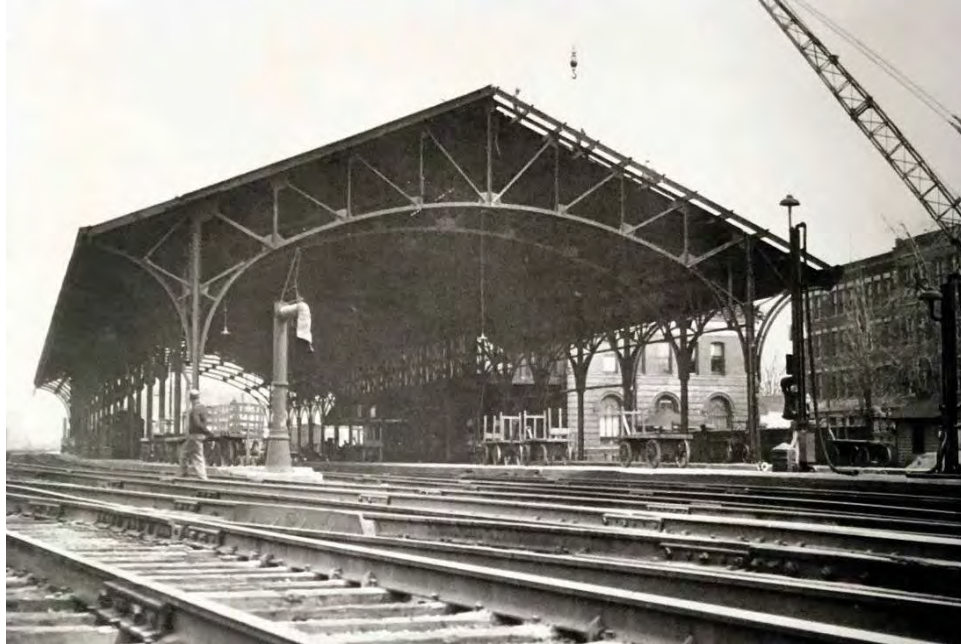
Photograph 5. View of train shed originally located north of the Richmond Railroad Station (visible in the background) prior to demolition, facing east.
