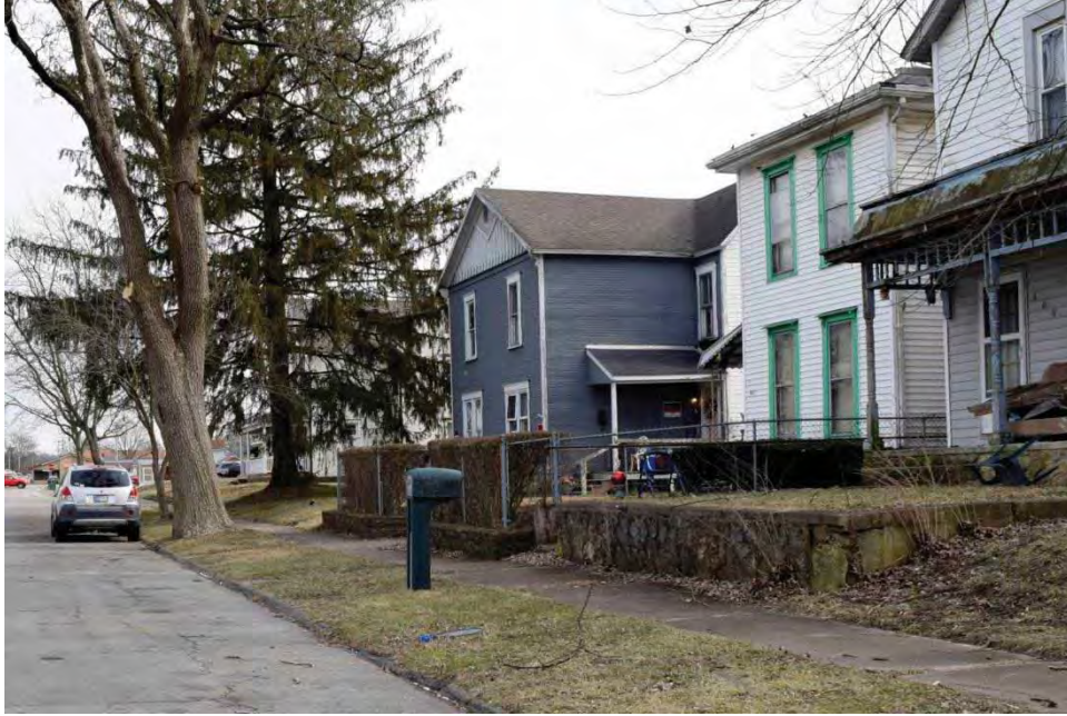
Photograph 21. View of the 800 block of North H Street, including IHSSI # 177-536-55184; AL004 at 813–815 North H Street, facing southeast.
