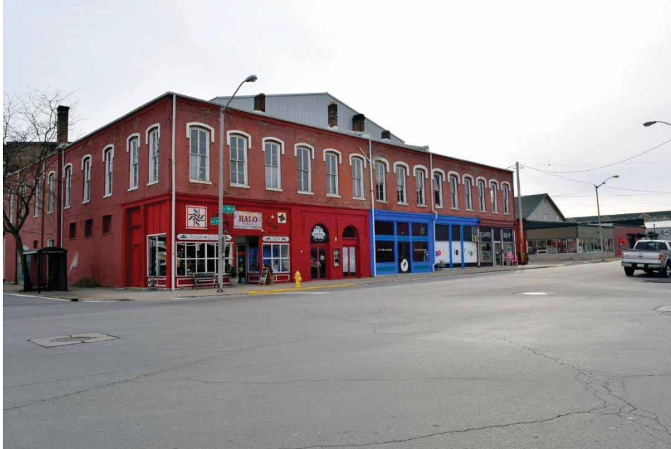
Photograph 37. View of the 400 block of North 8 th Street from Fort Wayne Avenue, facing southeast.
