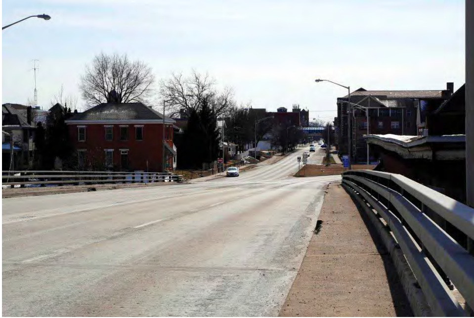
Photograph 29. View of US 27 and North 9 th Street, facing south from the US 27 bridge.
