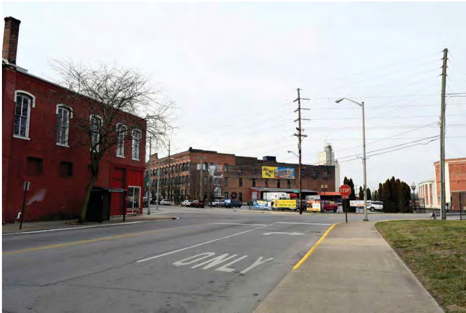
Photograph 40. View of the intersection of Fort Wayne Avenue, North E Street, and North 8 th Street, facing southwest on North E Street.
