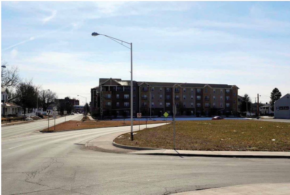
Photograph 30. View of 9 North Apartments at the junction of US 27 and North 9 th Street, facing south.
