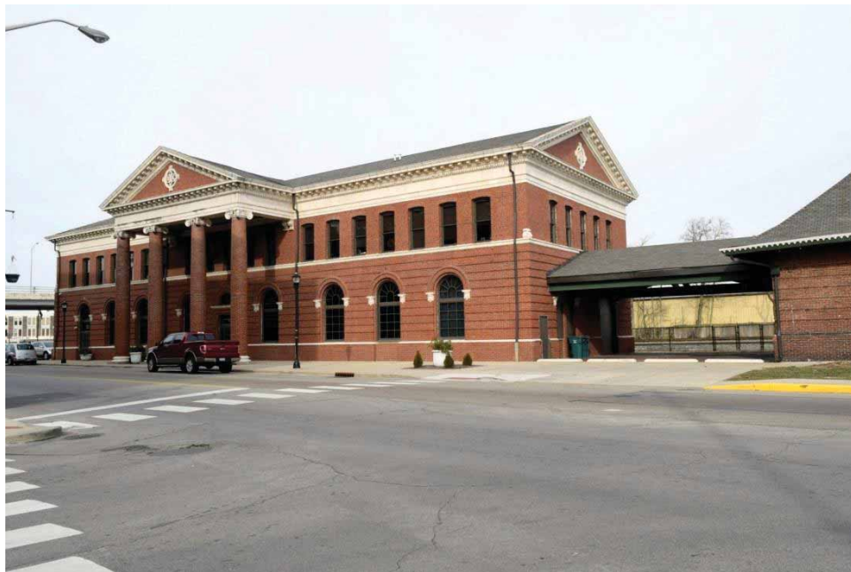
Photograph 8. View of the Richmond Railroad Station (IHSSI # 177-536-44002), the building after which the Richmond Railroad Station Historic District (NR-0781) was named, facing northwest.
