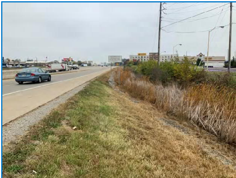
Photo 7 - View of EB I-465 entrance ramp at the Emerson Avenue and I-465 interchange facing east (10/20/2020).
