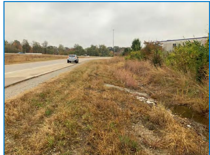
Photo 4 - View of SB I-465 entrance ramp at the Brookville Road and I-465 interchange facing south (10/20/2020).
