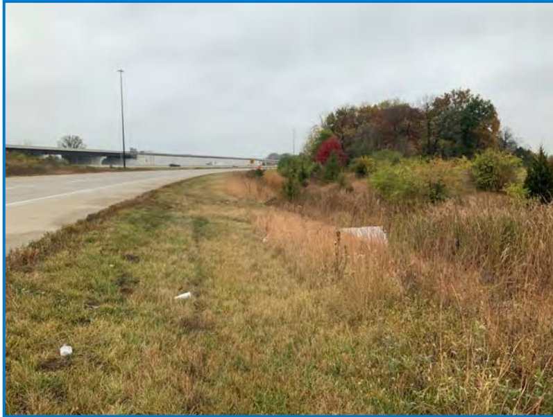
Photo 5 - View of SB Shadeland Avenue entrance ramp to SB I-465 facing southeast (10/20/2020).
