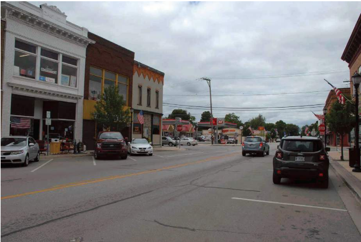
1. Fremont Historic Commercial District - This view looks west along SR 120 at the north end of the APE.
