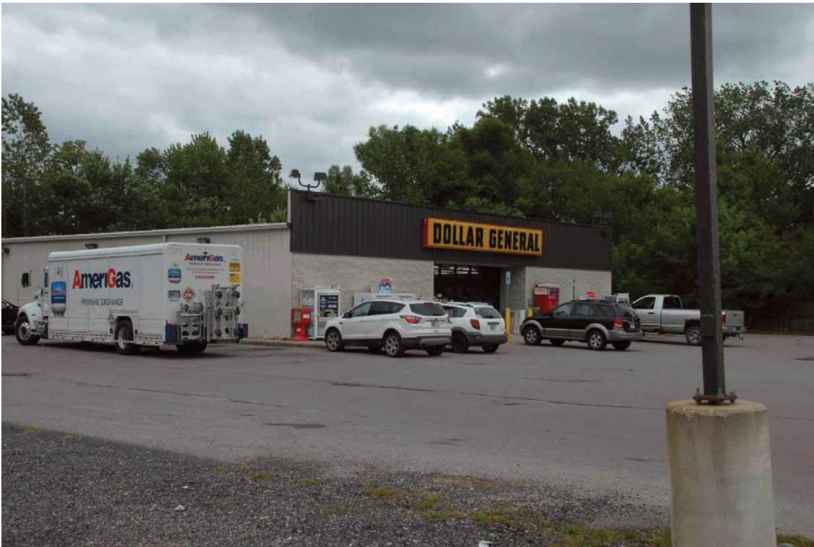
7. The Dollar General store was built on the site of the Fremont Lumber House (151-017-07047) that was demolished.
