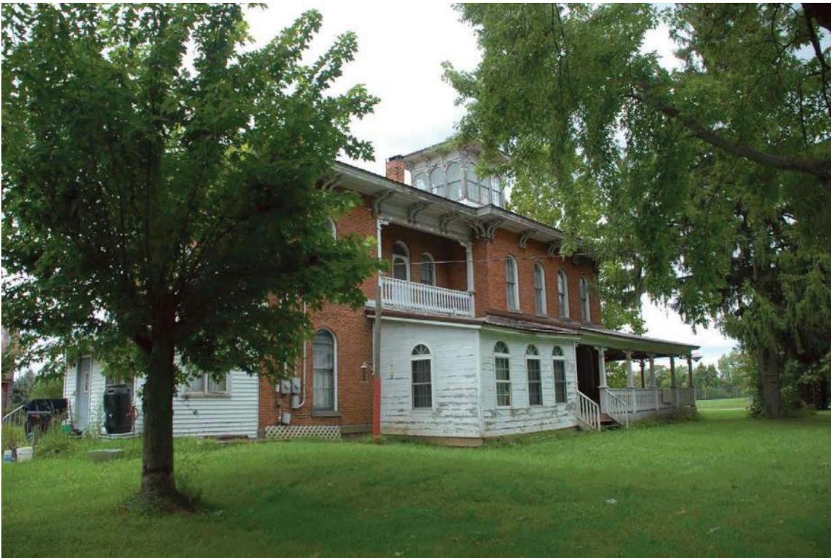
21. The Farnham House (151-017-05031) has some one story additions, looking northwest.
