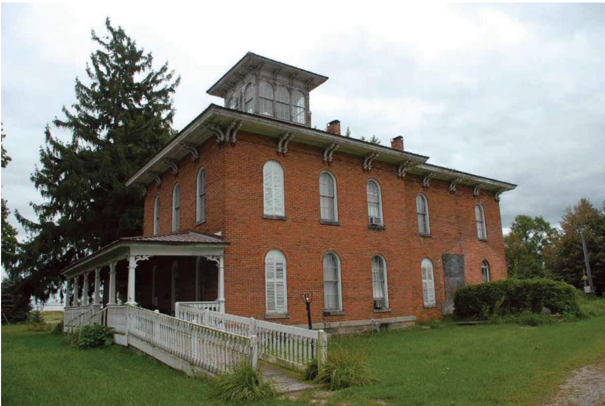
20. The brick Italianate-style Farnham house (151-017-05031) has paired brackets, round arch windows, and a cupola, looking east.
