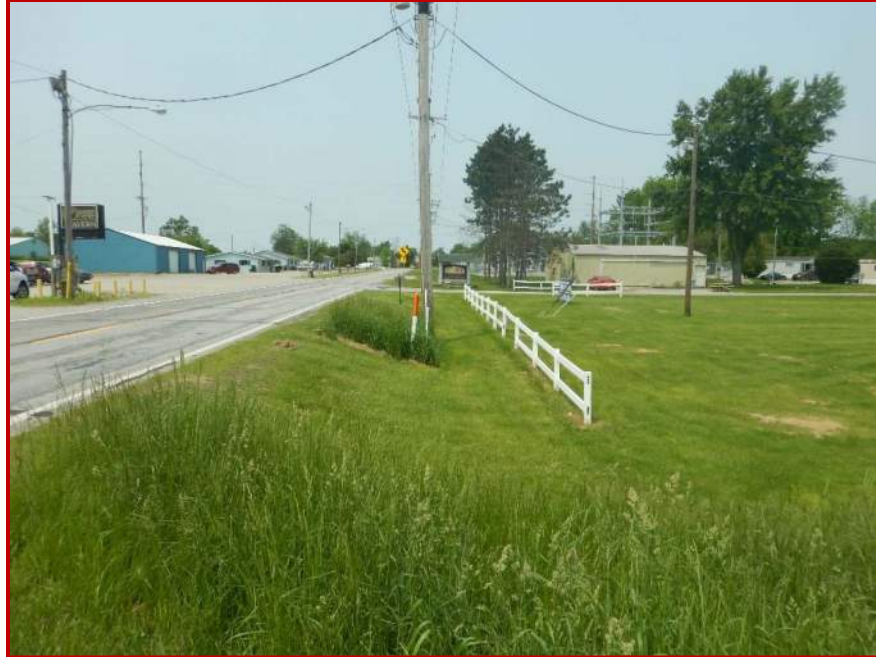
Photo 27. Looking west along SR 1 along the investigated area by AEP Electricity.
