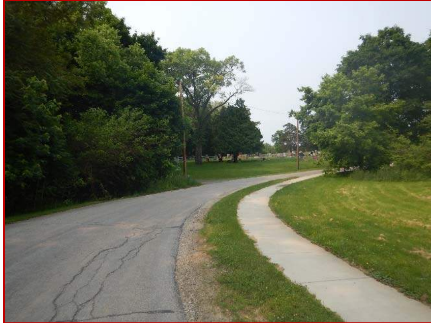
Photo 13. Looking southwest along Widney Street towards CR 60.
