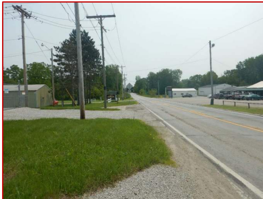
Photo 26. Looking east along SR 1 along the investigated area by AEP Electricity.
