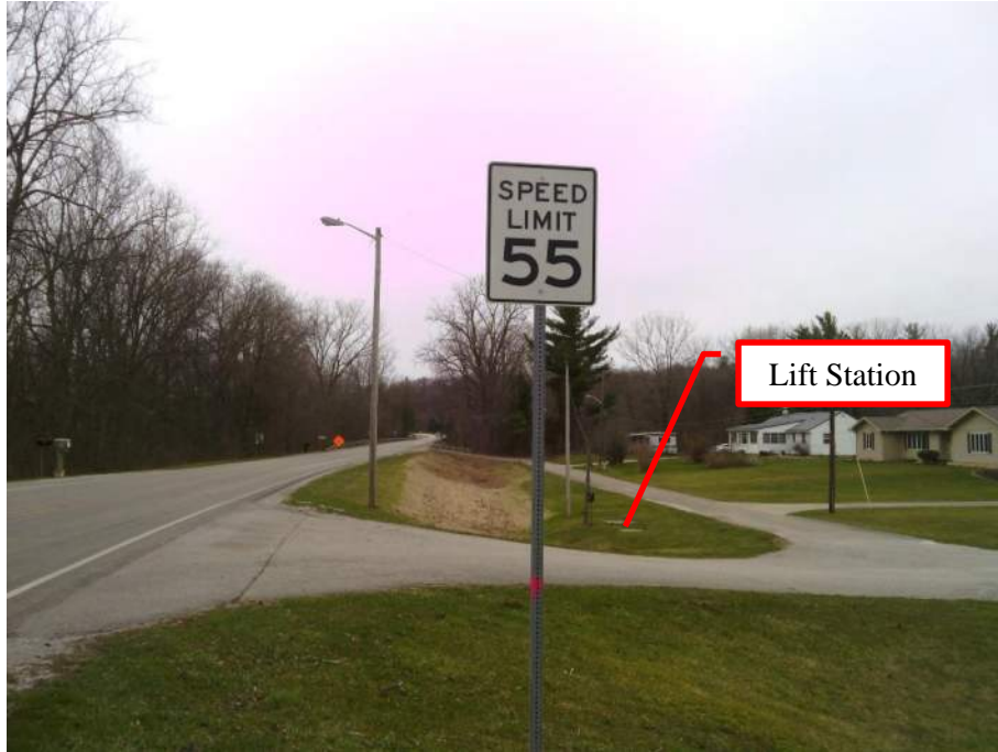
Approximately 200' west of North Street looking west at an open ditch.
