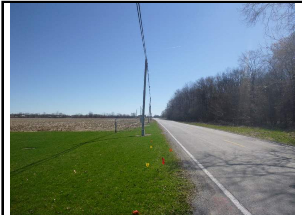
Looking east from the Fire Station driveway. Proposed ditch will follow the pole line approximately 800 feet east to a culvert under SR 16.
