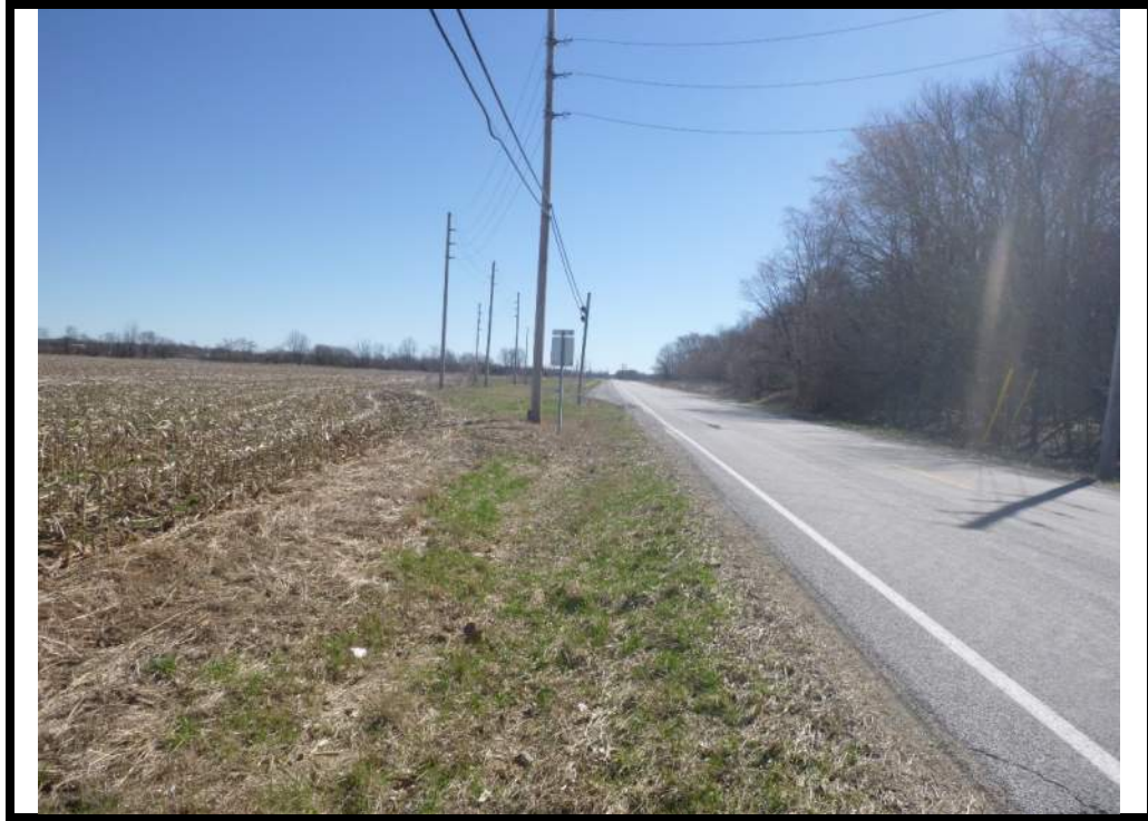
Looking east along the proposed ditch line approximately 500' east of the Fire Station driveway.
