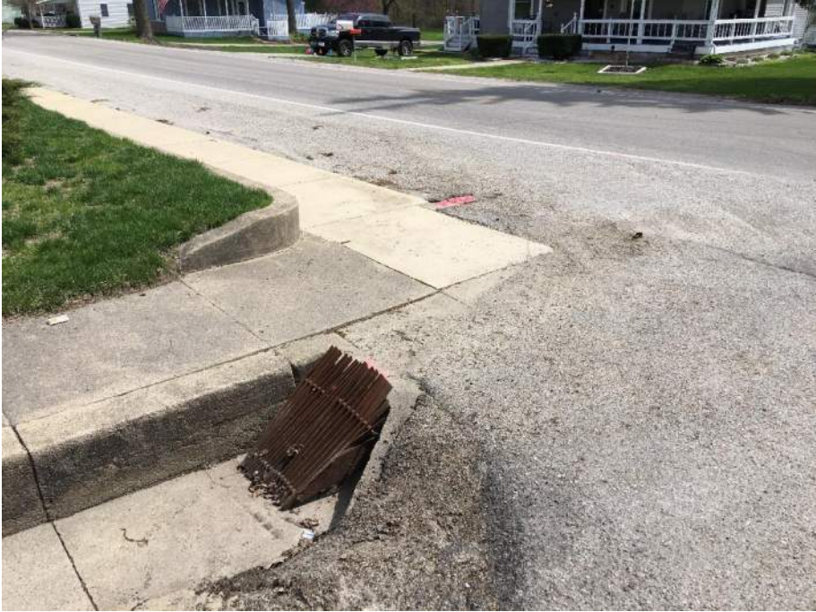
Drainage structure looking southeast at Yorick Street.
