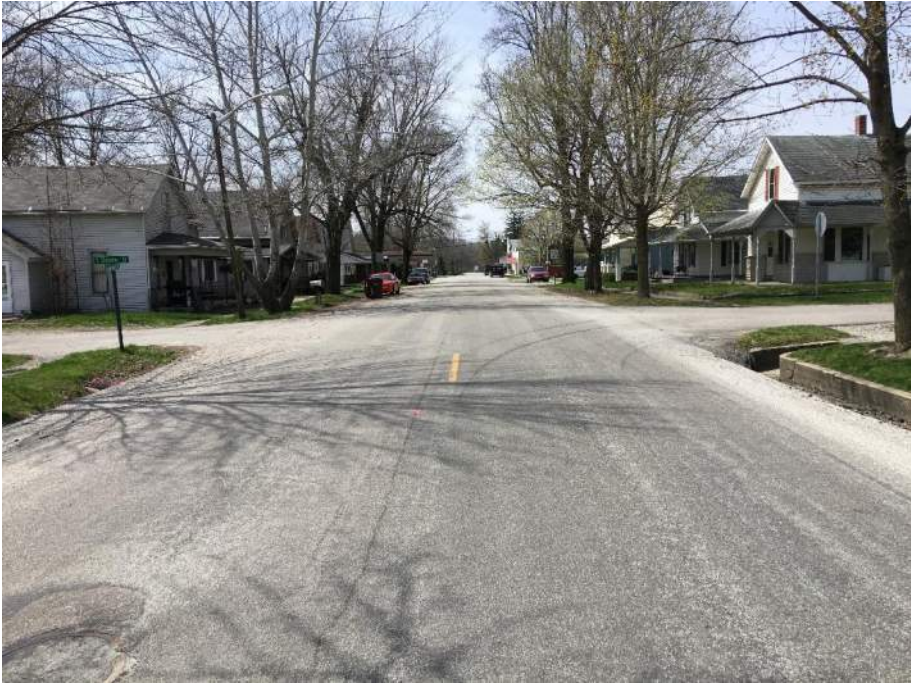
Looking east along SR 16 at Chandler Street.
