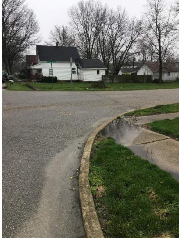
Ponding water on the southwest corner of Emmons Street and SR 28.
