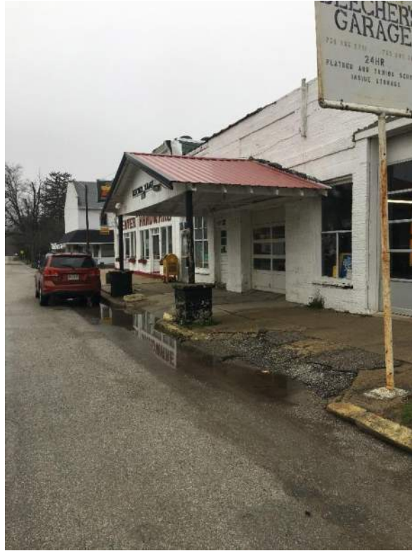
Ponding water at mid-block between Payson Street and Emmons Street looking west.
