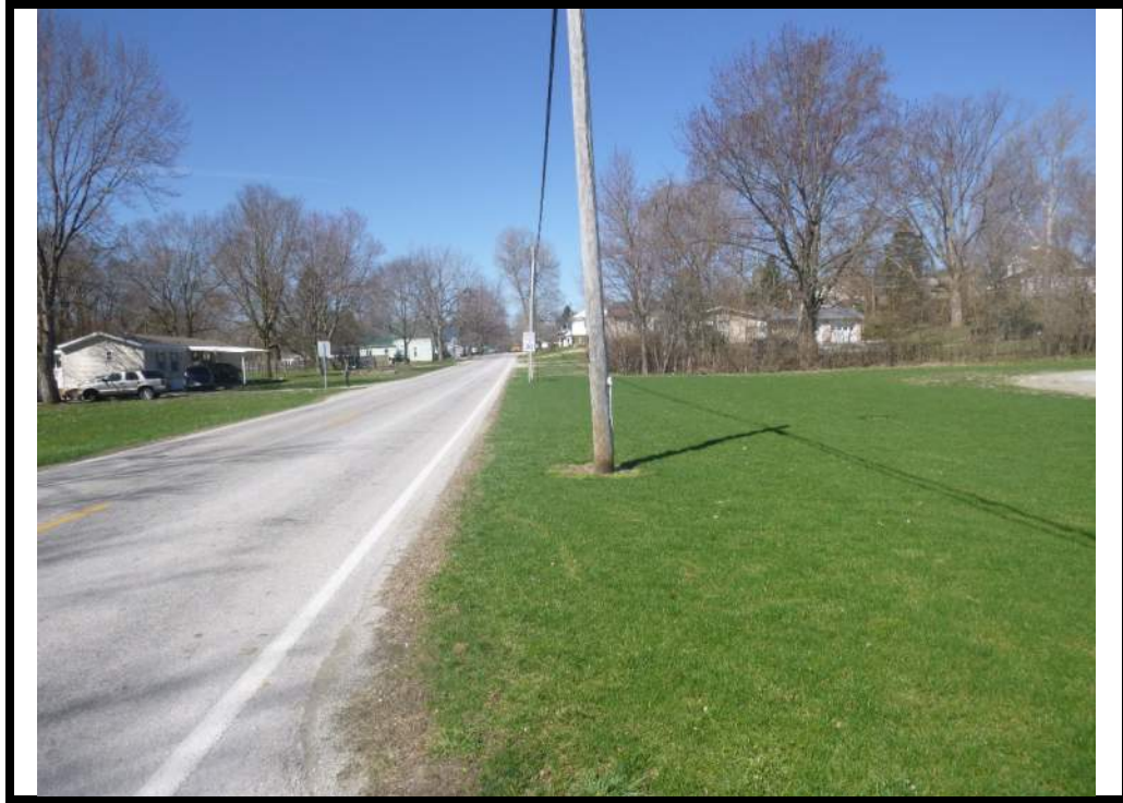
Looking west from the Fire Station driveway toward the start of the proposed ditch at the east end of the project.
