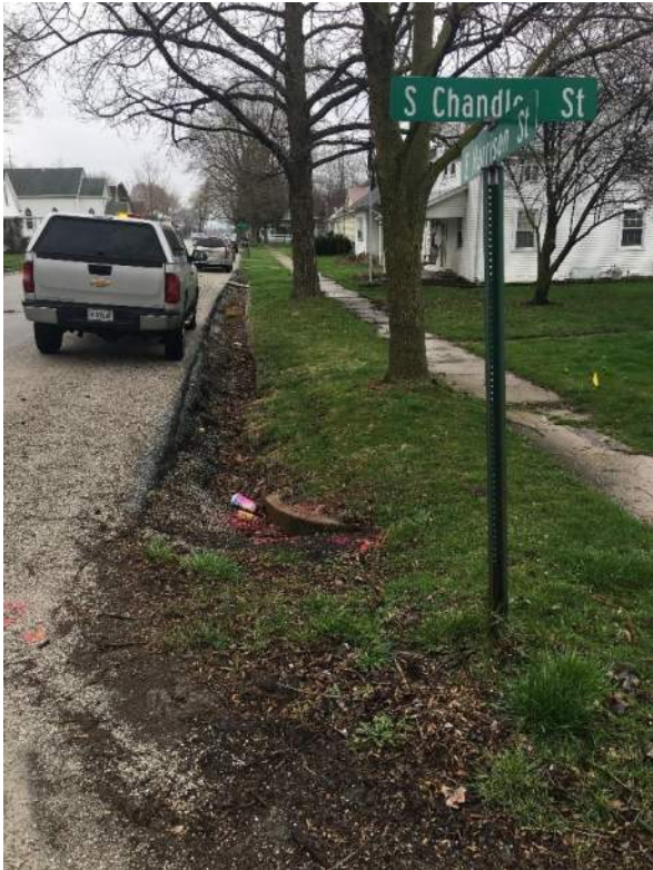
Safety and drainage issues along the south side of SR 16 at Chandler Street.
