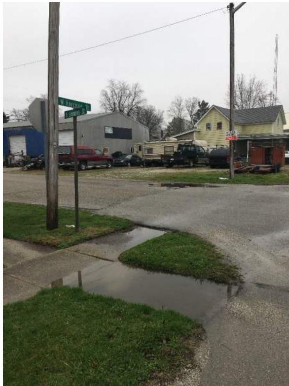
Ponding water on the northwest corner of Emmons Street and SR 28 looking northeast.
