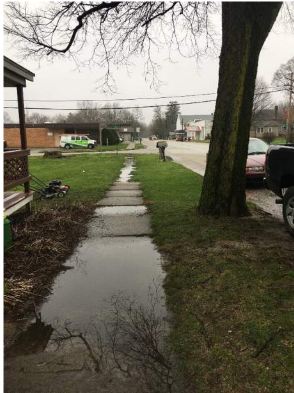
Ponding water at mid-block of Emmons Street and Chandler Street looking east.
