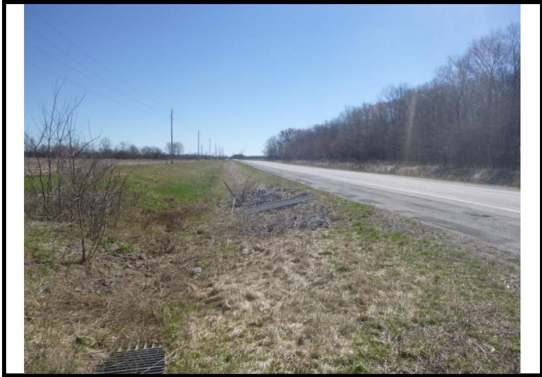
Looking east from the farm drive toward the north end of the culvert under SR 16 where the ditch will tie into the culvert.
