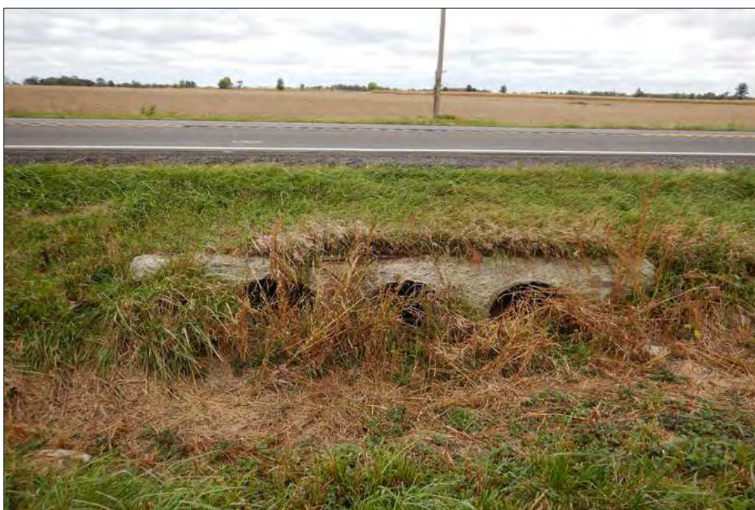
Photo 8: Project culvert outlet south of SR 234, facing north.
