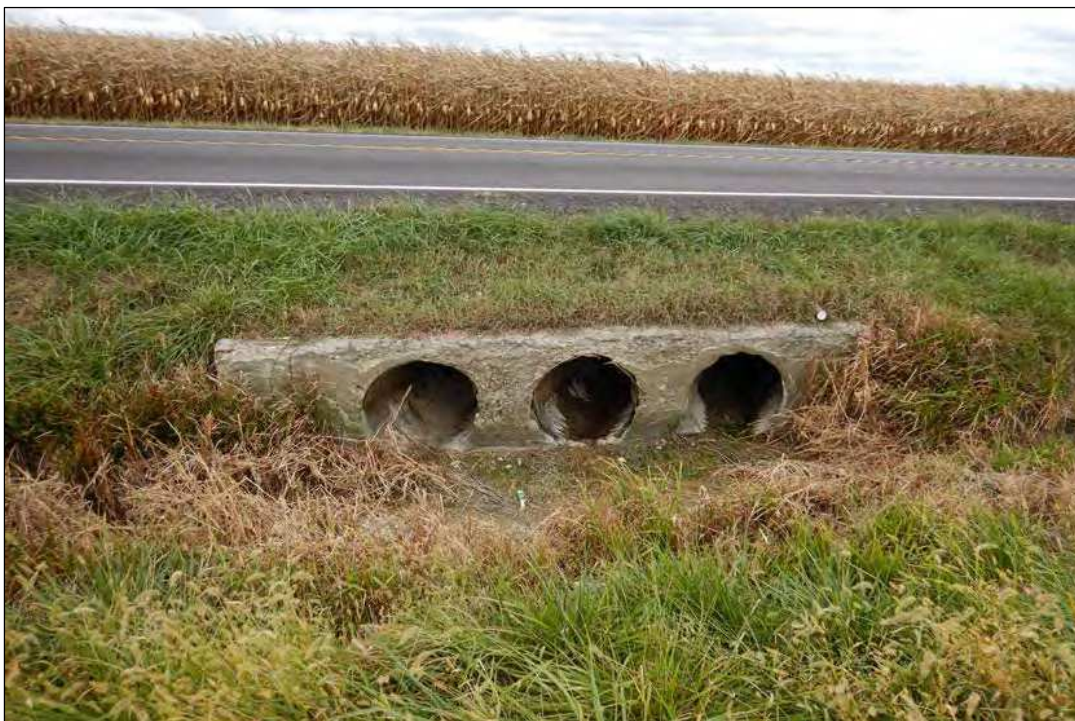
Photo 6: Project culvert inlet north of SR 234, facing south.
