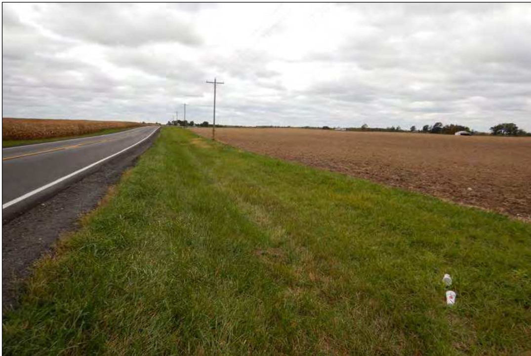
Photo 3: Roadway embankment north of SR 234 and east of the project culvert, facing west.
