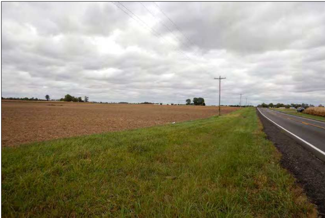
Photo 1: Roadway embankment north of SR 234 and west of the project culvert, facing east.
