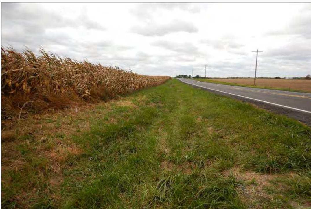
Photo 4: Roadway embankment south of SR 234 and east of the project culvert, facing west.
