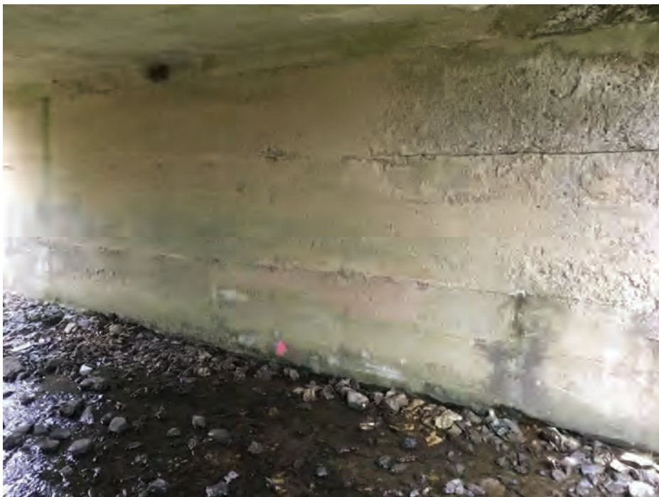
PHOTO 8 Condition Description West abutment condition
