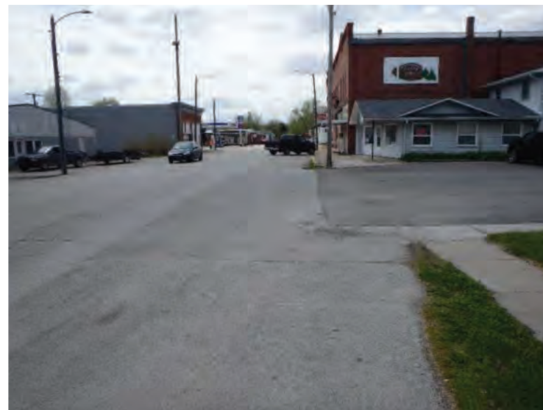
Picture 568: Looking west, toward the southern junction of SR 26 and SR 55, along the north side of SR 26 within Pine Village, 05/07/2020 (Exhibit 6AD)
