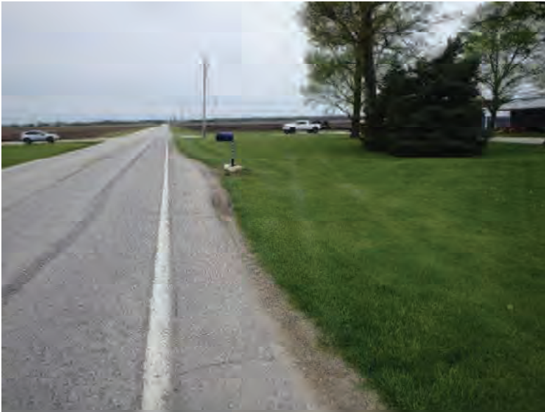
Picture 639: looking west along a mowed grass lawn on the north side of SR 26, east of Wetland 24, 05/04/2020 (Exhibit 6A1)
