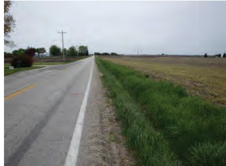
Picture 702: looking east along a roadside ditch on the south side of SR 26, west of N 725 E, 05/04/2020 (Exhibit 6AM)
