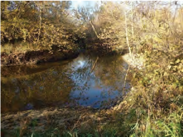
Picture 543: Looking southwest along Big Pine Creek towards UNT7 to Big Pine Creek from the south side of SR 26, 11/05/2019 (Exhibit 6AB)
