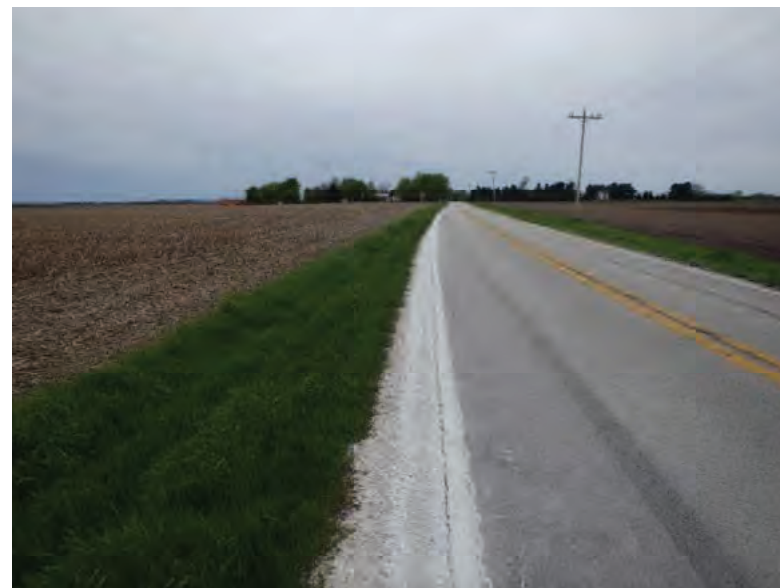
Picture 722: looking west along a roadside ditch on the south side of SR 26, east of N 725 E and west of N 875 E, 05/04/2020 (Exhibit 6AO)
