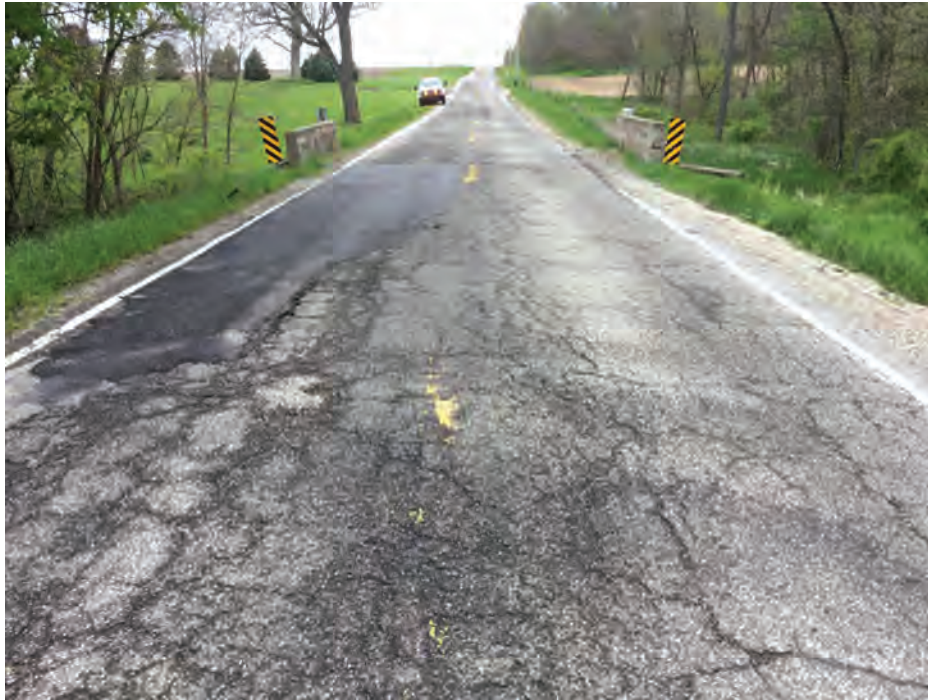
PHOTO 1 Condition Description Road alignment looking west
