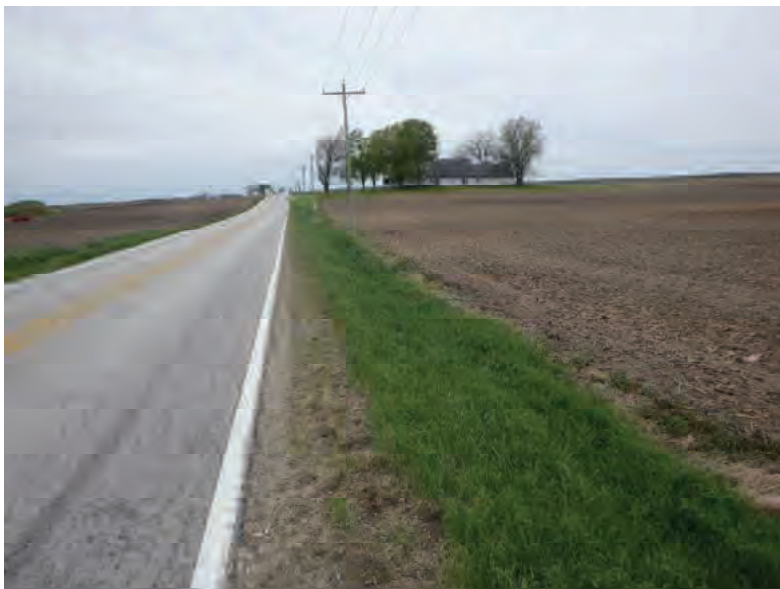
Picture 691: looking west along a roadside ditch on the north side of SR 26, 05/04/2020 (Exhibit 6AK)
