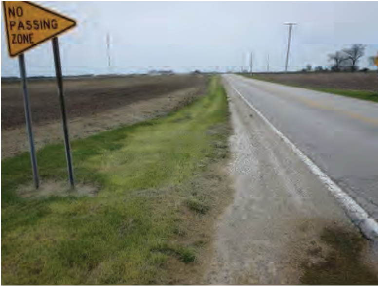
Picture 589: looking east along a roadside ditch on the north side of SR 26, adjacent to N 450 E, 05/04/2020 (Exhibit 6AF)
