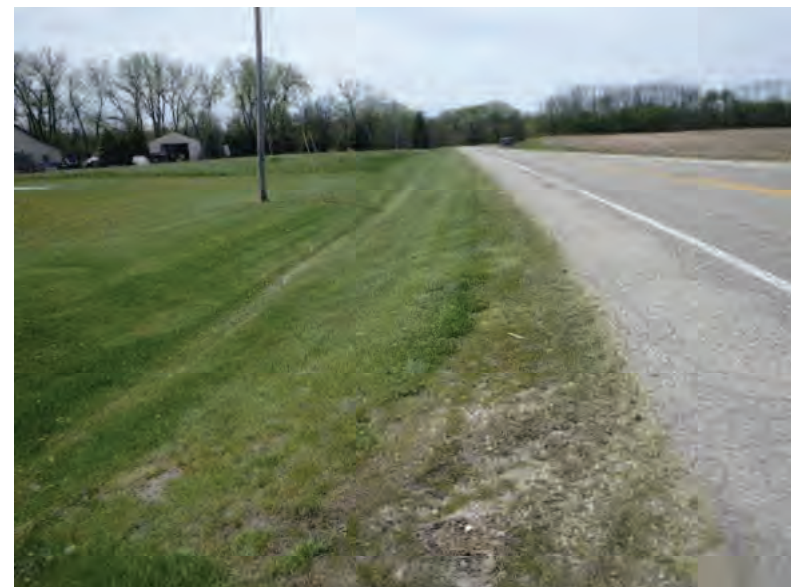
Picture 504: Looking southwest along a roadside ditch on the south side of SR 26, 05/04/2020 (Exhibit 6AA)
