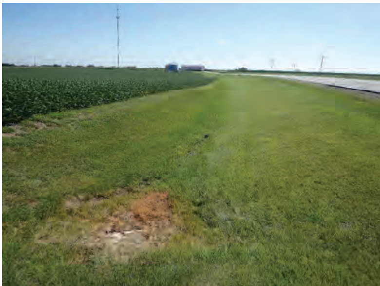
Picture 593: looking east along a grassed roadside ditch on the north side of SR 26, east of N 450 E, 09/04/2019 (Exhibit 6AF)
