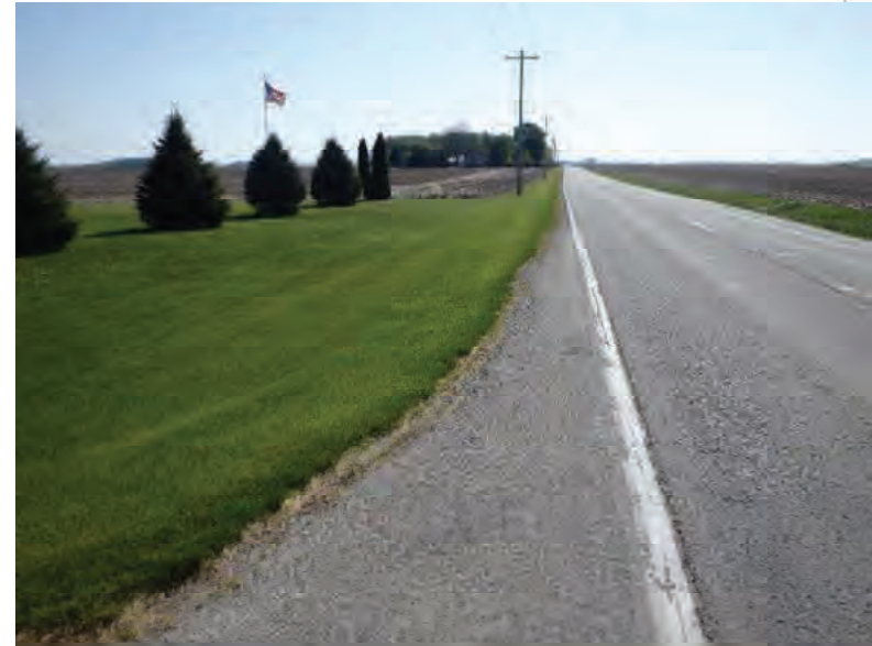
Picture 804: looking east along a roadside ditch on the north side of SR 26, east of Holder Ditch and west of N 1100 E, 05/07/2020 (Exhibit 6AT)
