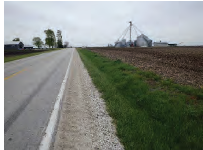
Picture 626: looking east along a roadside ditch on the south side of SR 26, toward Wetland 24, 05/04/2020 (Exhibit 6AH)
