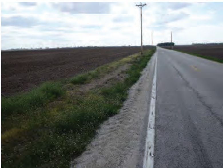
Picture 847: looking west along a roadside ditch on the south side of SR 26, east of Gephart-Magee Ditch and west of N 1100 E, 05/07/2020 (Exhibit 6AX)
