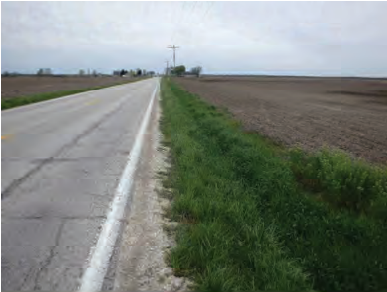
Picture 695: looking west along a roadside ditch on the north side of SR 26, 05/04/2020 (Exhibit 6AK)
