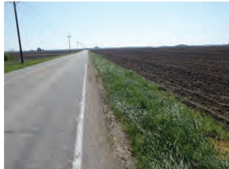
Picture 810: looking east along a roadside ditch on the south side of SR 26, east of Holder Ditch and west of N 1100 E, 05/07/2020 (Exhibit 6AU)
