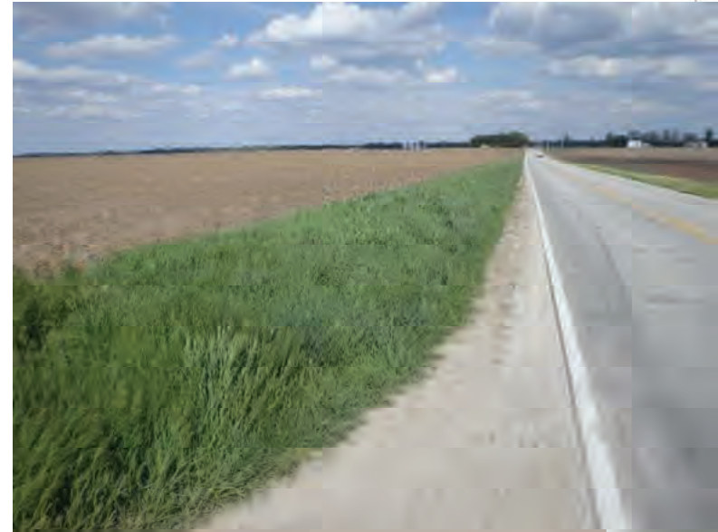
Picture 856: looking east along a roadside ditch on the north side of SR 26, adjacent to N 1150 E, 05/07/2020 (Exhibit 6AY)
