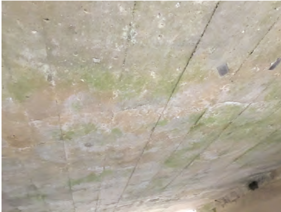
PHOTO 13 Condition Description Bottom of slab condition
