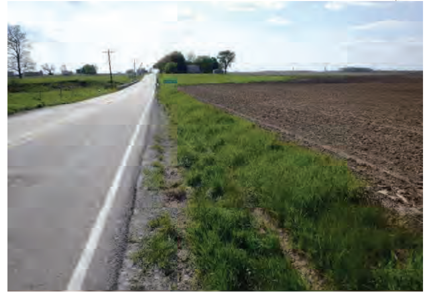
Picture 898: looking west along a roadside ditch on the north side of SR 26, adjacent to the eastern end of the project, 05/07/2020 (Exhibit 6AZ)
