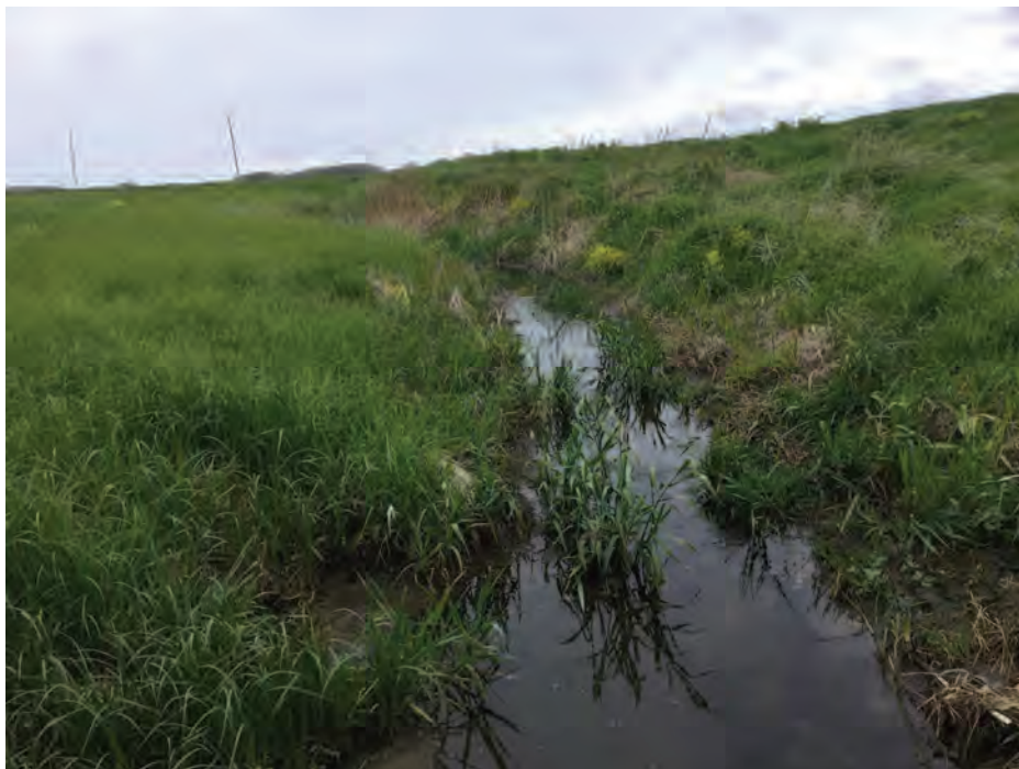
PHOTO 11 Condition Description Up stream alignment or looking north
