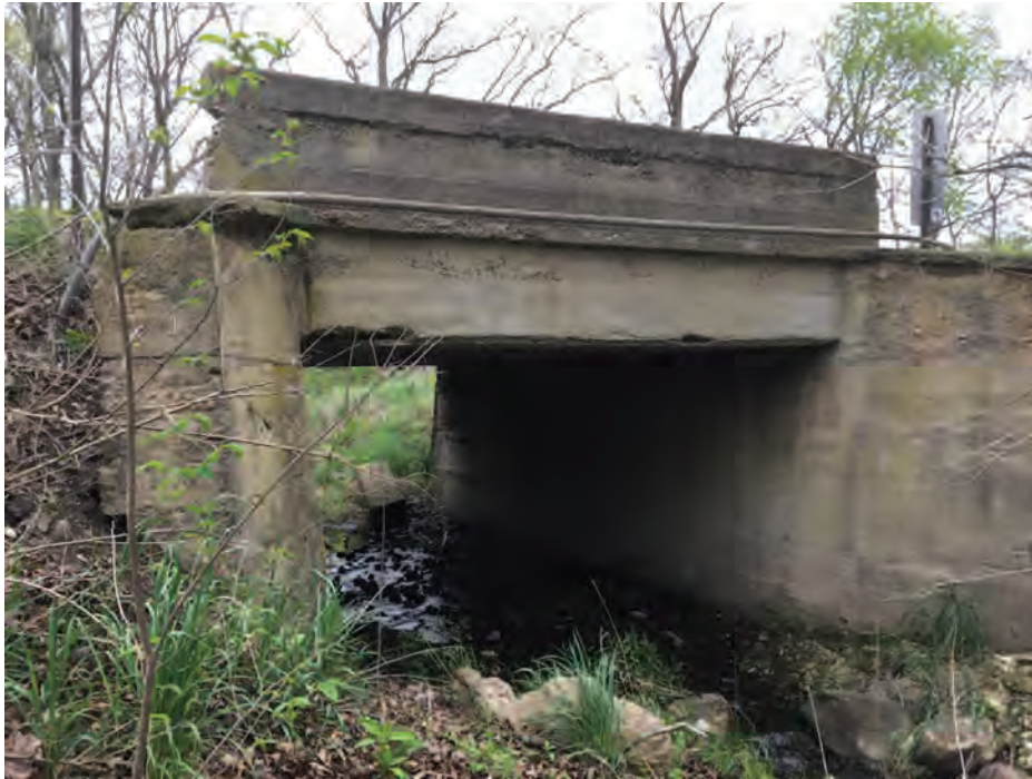
PHOTO 7 Condition Description Profile looking North
