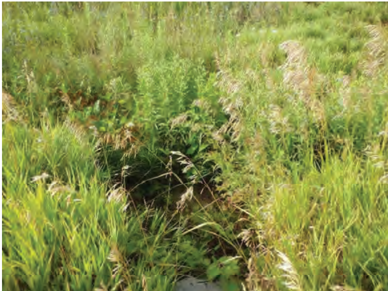
Picture 601: looking south, at the southern opening of structure CLV 026 86 17.19 on the south side of SR 26; no channel present, 07/19/2019 (Exhibit 6AF)
