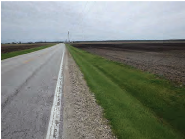
Picture 627: looking west along a roadside ditch on the north side of SR 26, 05/04/2020 (Exhibit 6AH)
