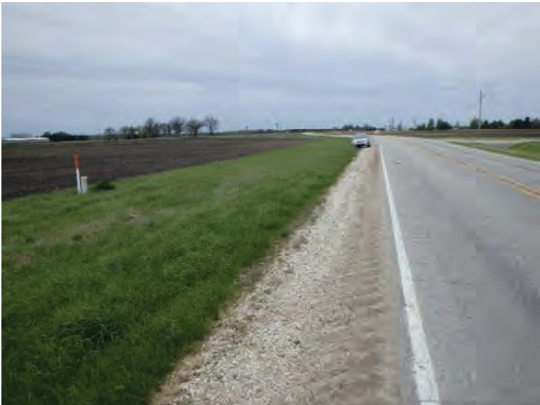
Picture 609: looking west along a roadside ditch on the south side of SR 26, 05/04/2020 (Exhibit 6AG)
