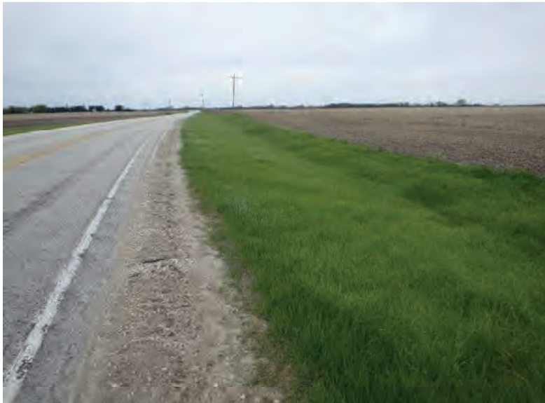
Picture 737: looking northwest along a roadside ditch on the north side of SR 26, east of N 725 E and west of N 875 E, 05/04/2020 (Exhibit 6AP)
