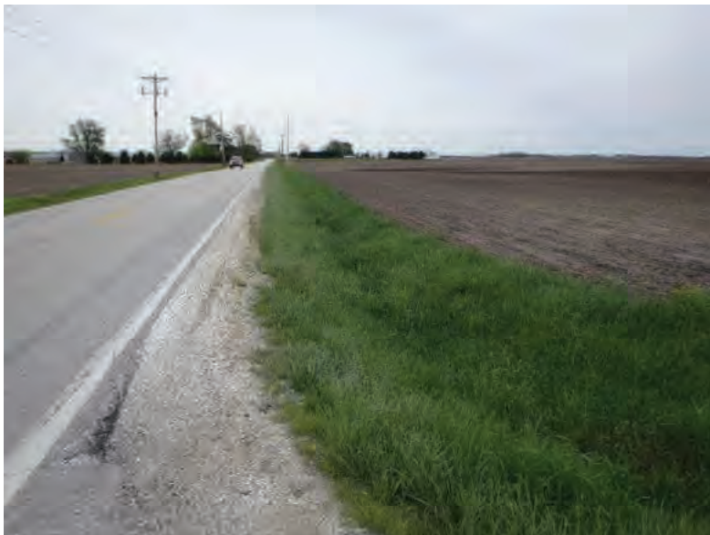
Picture 761: looking east along a roadside ditch on the south side of SR 26, adjacent to N 875 E, 05/04/2020 (Exhibit 6AQ)
