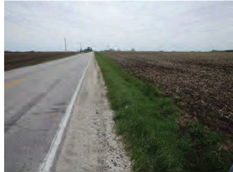
Picture 612: looking east along a roadside ditch on the south side of SR 26, 05/04/2020
