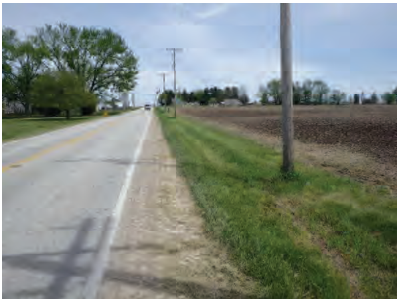
Picture 573: Looking east along a roadside ditch on the south side of SR 26, adjacent to Pine Village Elementary School, 05/04/2020 (Exhibit 6AD)
