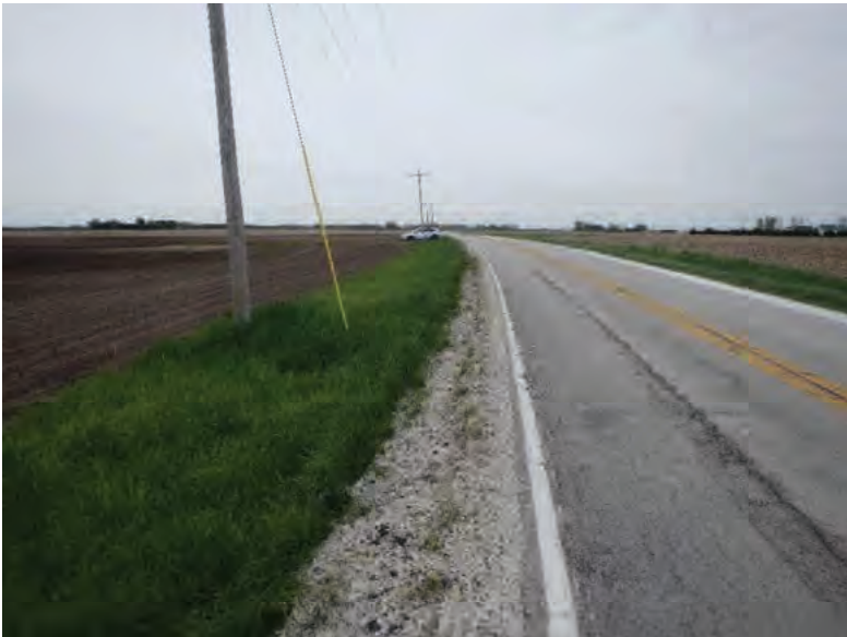
Picture 725: looking east along a roadside ditch on the north side of SR 26, east of N 725 E and west of N 875 E, 05/04/2020 (Exhibit 6AO)
