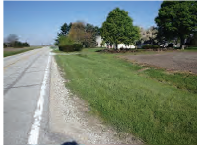
Picture 780: looking west along a roadside ditch on the north side of SR 26, east of N 875 E and west of Holder Ditch, 05/07/2020 (Exhibit 6AS)
