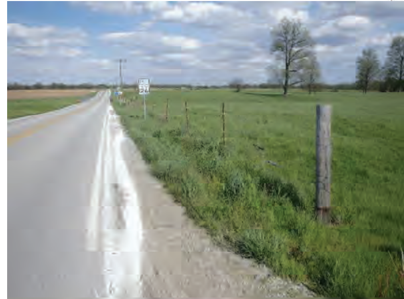
Picture 868: looking east along a roadside ditch on the south side of SR 26, adjacent to County Line Road, 05/07/2020 (Exhibit 6AZ)
