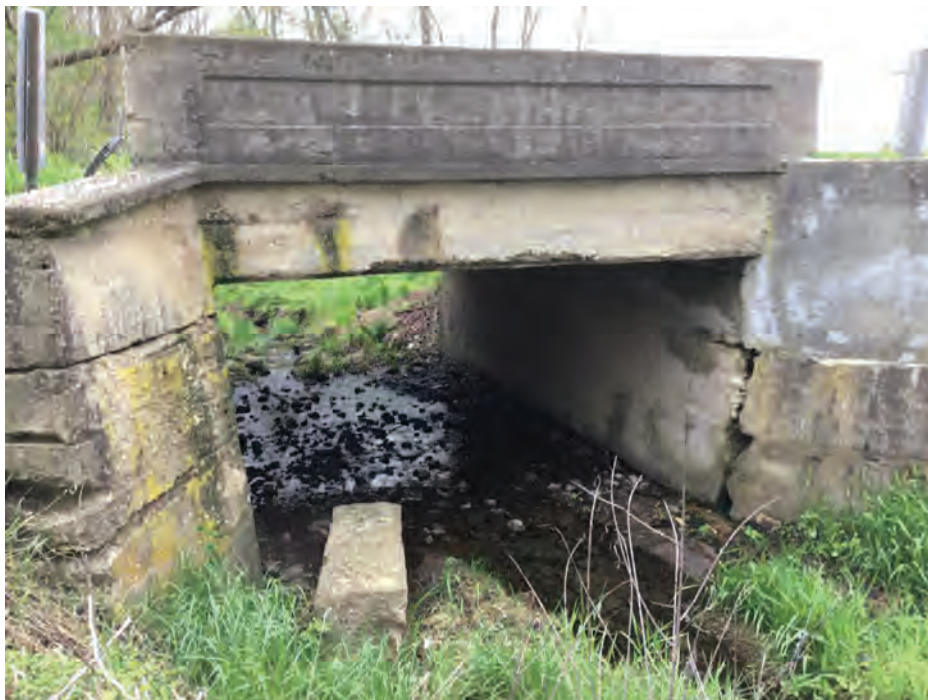
PHOTO 6 Elevation, Condition Description Profile looking south
