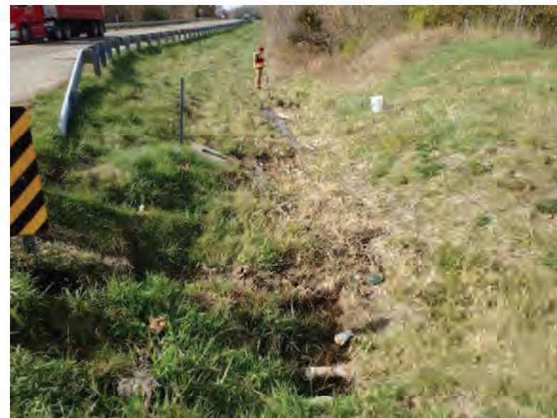
Picture 540: Looking west at Wetland 33, located on the north side of SR 26, within a roadside ditch, adjacent to E Akers Rd, 11/05/2019 (Exhibit 6AB)
