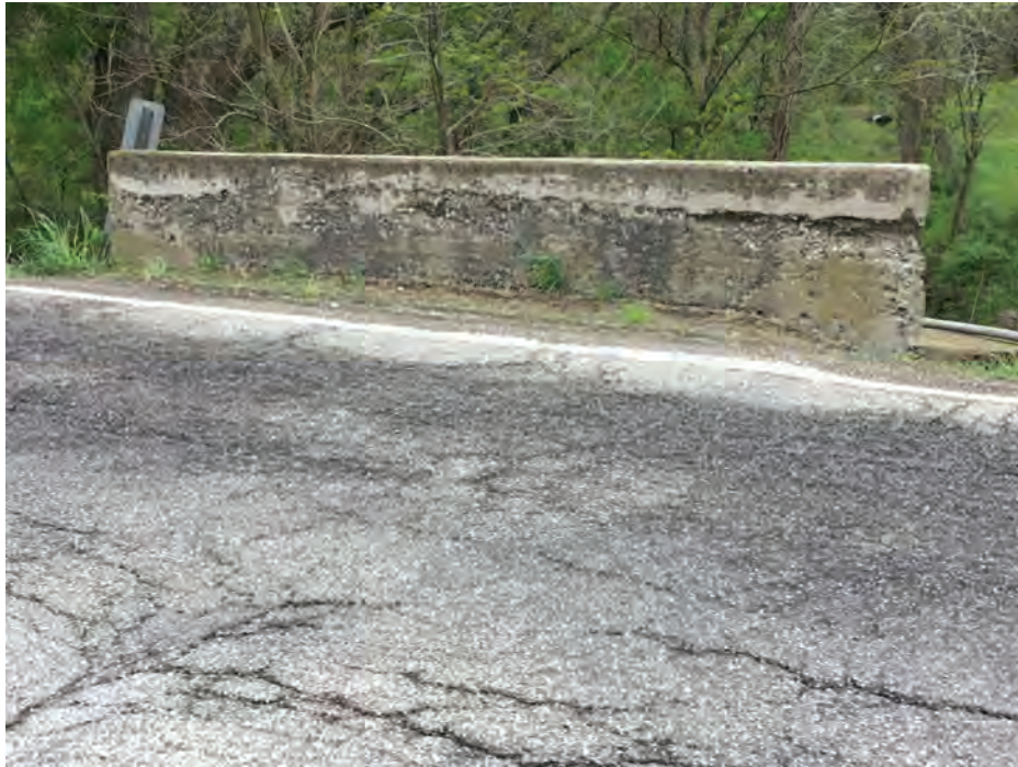
PHOTO 5 Condition Description South parapet wall condition
