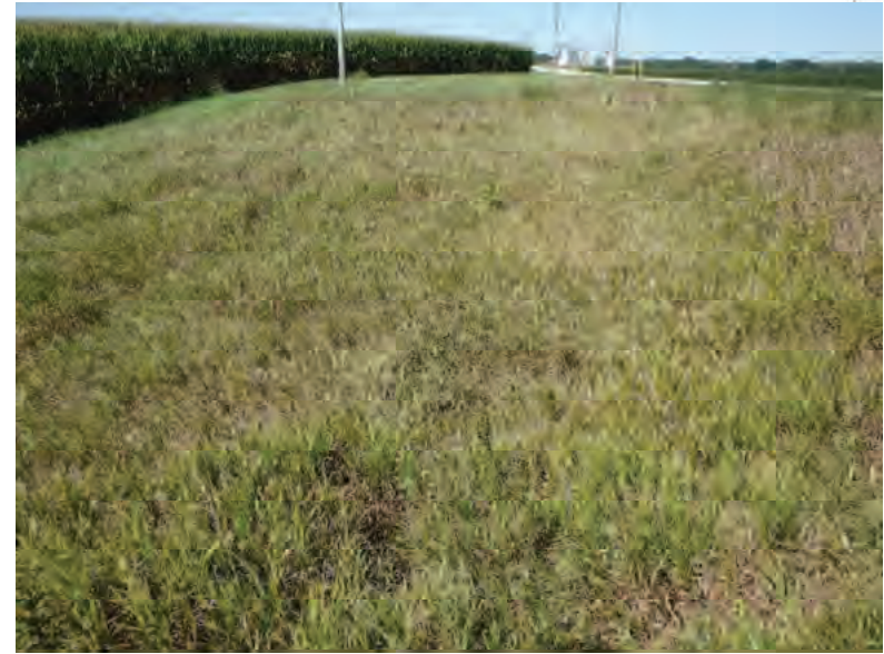
Picture 590: looking west along a grassed roadside ditch on the south side of SR 26, east of N 450 E, 09/04/2019 (Exhibit 6AF)
