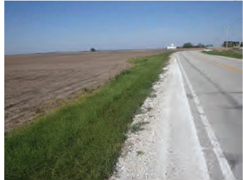
Picture 788: looking west along a grassed slope on the south side of SR 26, east of N 875 E and west of Holder Ditch, 05/07/2020 (Exhibit 6AS)
