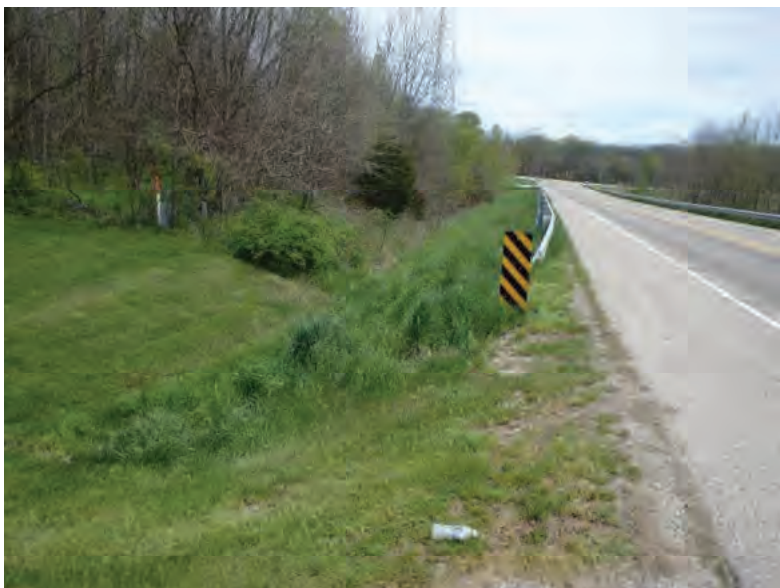
Picture 519: Looking east along a roadside ditch, towards UNT7 to Big Pine Creek, on the north side of SR 26, 05/04/2020 (Exhibit 6AB)
