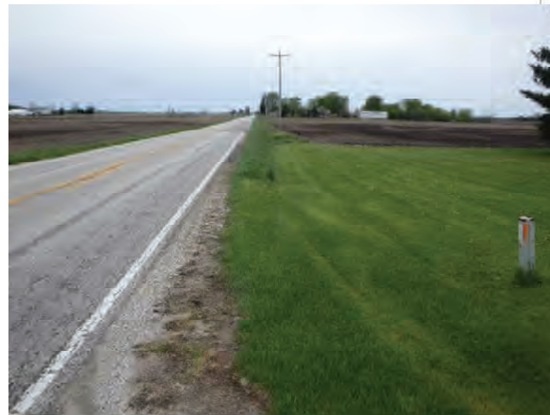
Picture 720: looking west along a roadside ditch and mown lawn on the north side of SR 26, east of N 725 E, 05/04/2020 (Exhibit 6AN)
