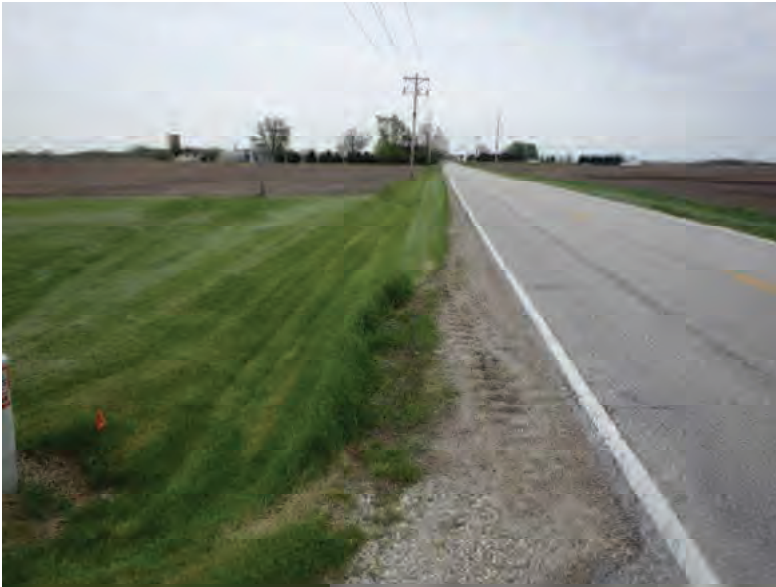
Picture 763: looking east along a roadside ditch on the north side of SR 26, adjacent to N 875 E, 05/04/2020 (Exhibit 6AQ)
