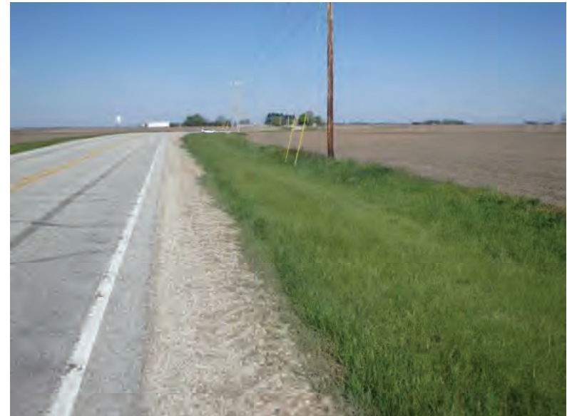
Picture 790: looking west along a roadside ditch on the north side of SR 26, east of N 875 E and west of Holder Ditch, 05/07/2020 (Exhibit 6AS)
