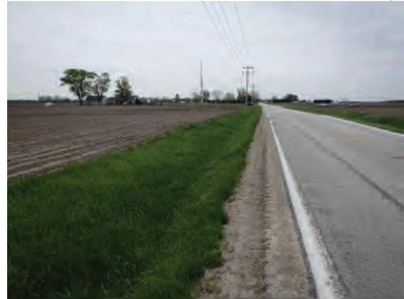
Picture 750: looking east, toward N 875 E, along a roadside ditch on the north side of SR 26, 05/04/2020 (Exhibit 6AQ)
