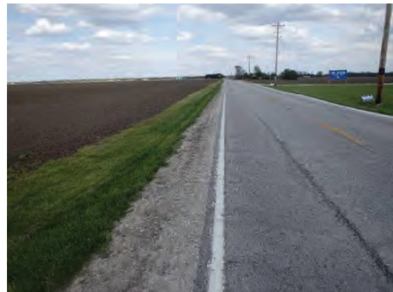
Picture 850: looking east along a roadside ditch on the north side of SR 26, east of Gephart-Magee Ditch and west of N 1100 E, 05/07/2020 (Exhibit 6AX)
