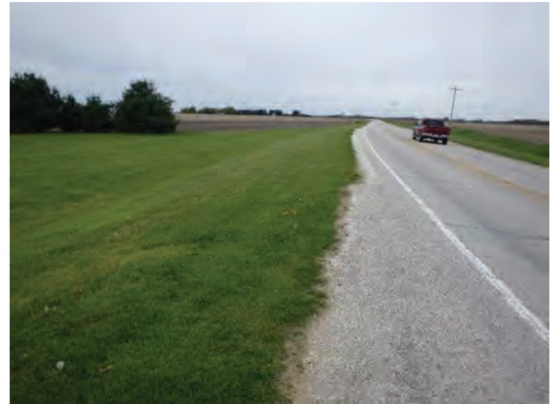
Picture 734: looking northwest along a roadside ditch on the south side of SR 26, east of N 725 E and west of N 875 E, 05/04/2020 (Exhibit 6AP)
