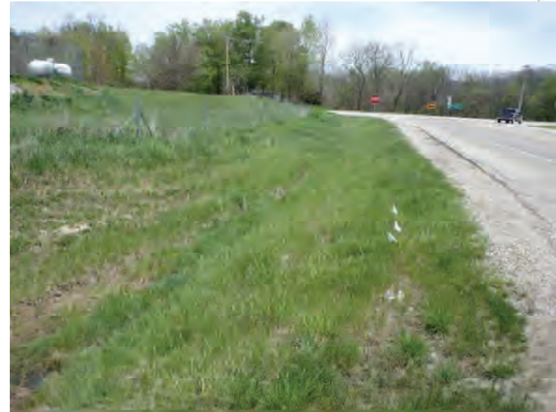
Picture 542: Looking east along a roadside ditch towards SR 55, on the north side of SR 26, adjacent to E Akers Rd, 05/04/2020 (Exhibit 6AB)
