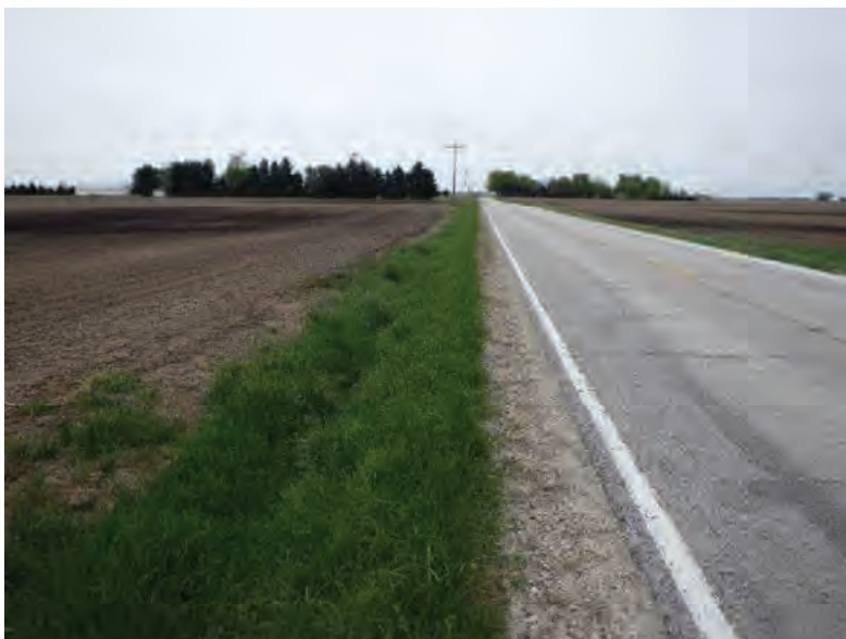
Picture 717: looking east along a roadside ditch on the north side of SR 26, east of N 725 E, 05/04/2020 (Exhibit 6AM)
