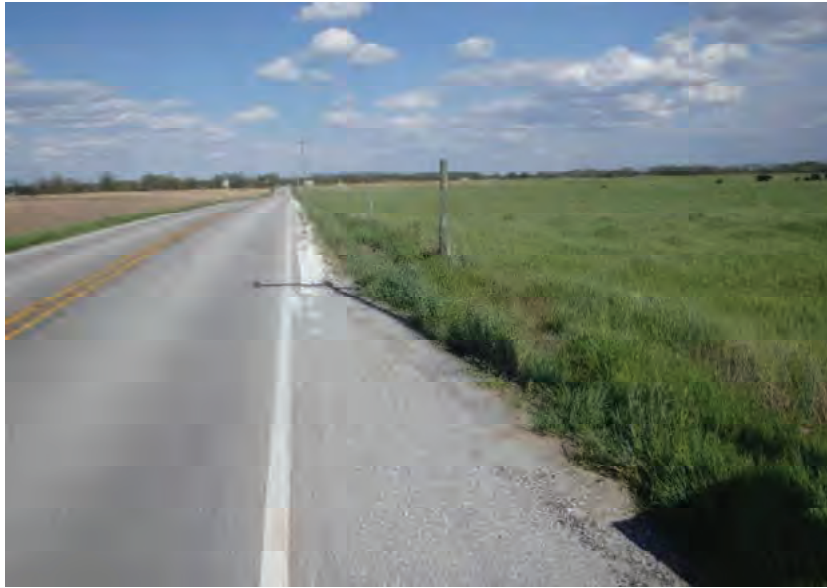
Picture 897: looking east, beyond the project limits, along a roadside ditch on the south side of SR 26, adjacent to the eastern end of the project, 05/07/2020 (Exhibit 6AZ)
