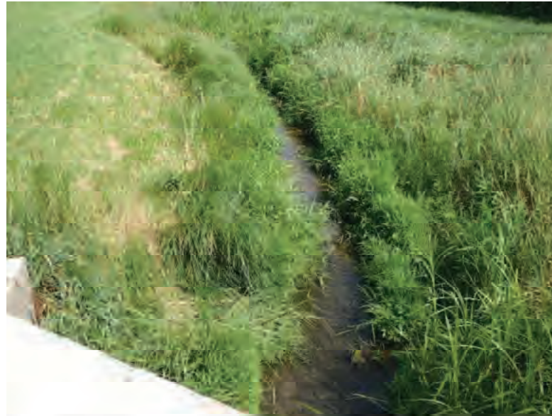
Picture 882: looking north, upstream, along UNT1 to Little Pine Creek at Wetland 35, from the top of the structure, on the north side of SR 26 and east of County Line Rd., 07/19/2019 (Exhibit 6AZ)
