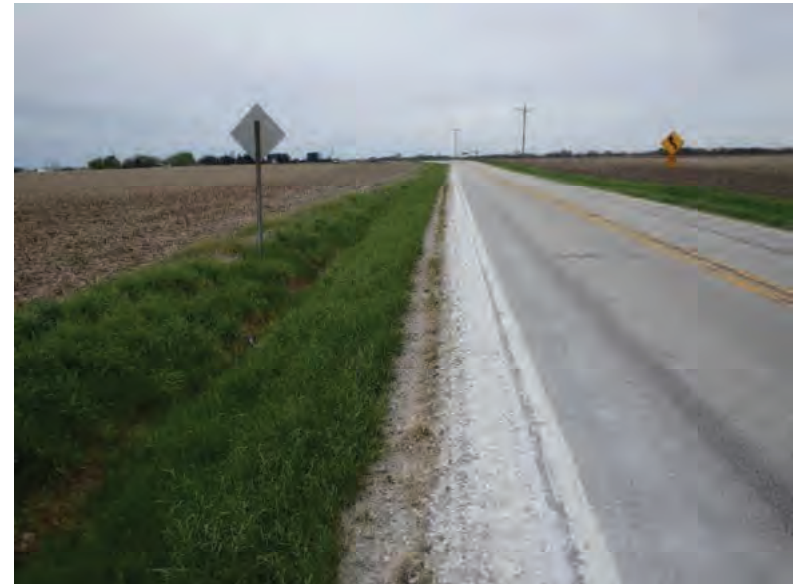
Picture 730: looking northwest along a roadside ditch on the south side of SR 26, east of N 725 E and west of N 875 E, 05/04/2020 (Exhibit 6AO)
