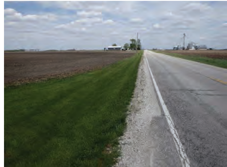
Picture 622: looking east along a roadside ditch on the north side of SR 26, 05/07/2020 (Exhibit 6AH)
