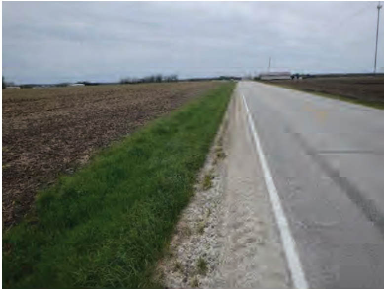
Picture 611: looking west along a roadside ditch on the south side of SR 26, 05/04/2020 (Exhibit 6AG)
