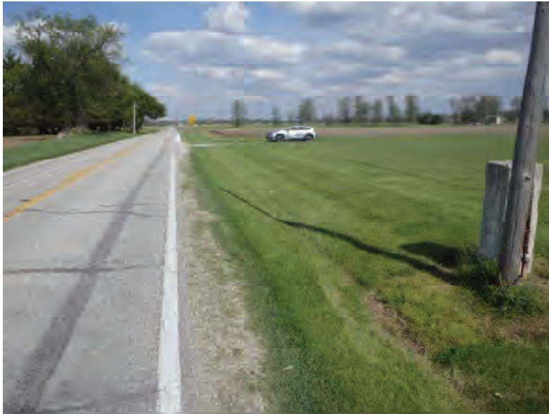
Picture 863: looking east along a roadside ditch on the south side of SR 26, east of N 1150 E and west of County Line Road, 05/07/2020 (Exhibit 6AZ)
