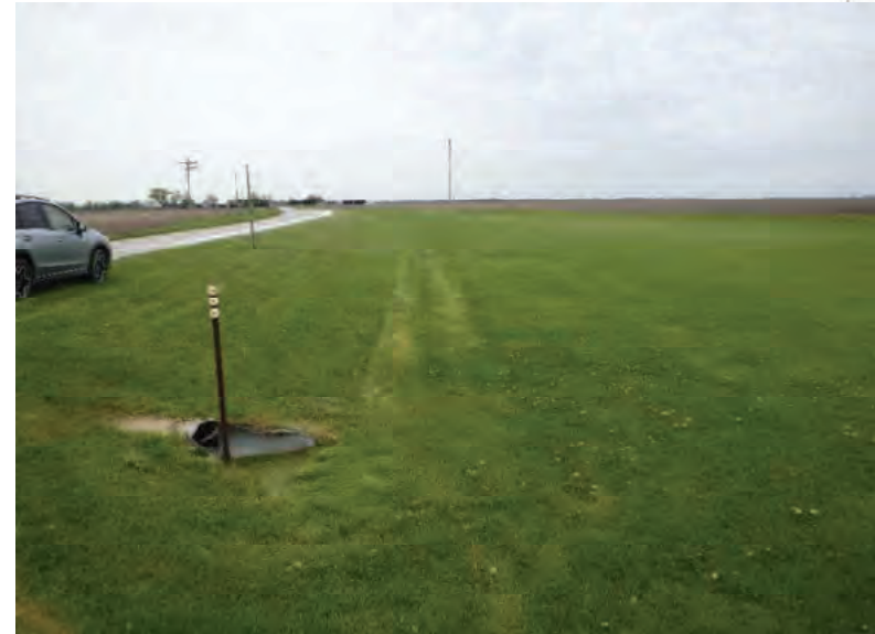
Picture 736: looking southeast along a roadside ditch, at the south opening of structure CLV 026 86 20.87 on the south side of SR 26, east of N 725 E and west of N 875 E, 05/04/2020 (Exhibit 6AP)
