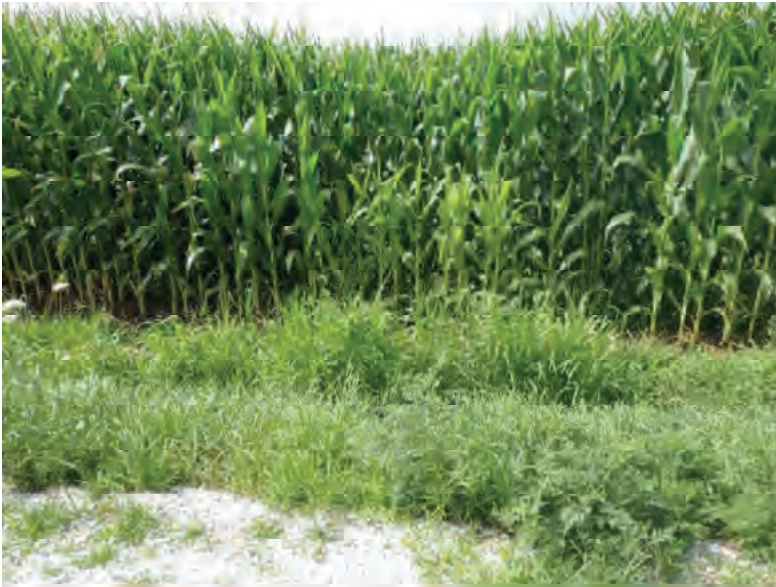
Picture 851: looking south at the buried opening of structure CLV 026 86 23.94 and a roadside ditch on the south side of SR 26, east of N 1100 E and west of N 1150 E, 07/19/2019 (Exhibit 6AY)
