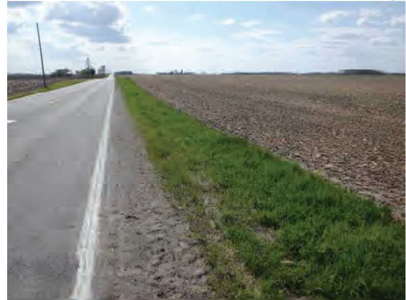
Picture 864: looking west along a roadside ditch on the north side of SR 26, east of N 1150 E and west of County Line Road, 05/07/2020 (Exhibit 6AZ)
