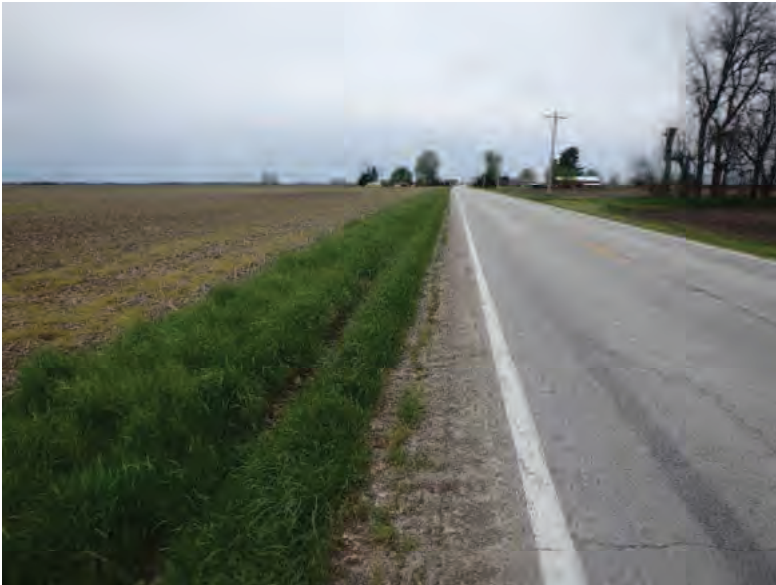
Picture 701: looking west along a roadside ditch on the south side of SR 26, west of N 725 E, 05/04/2020 (Exhibit 6AM)
