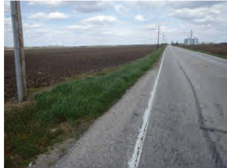
Picture 844: looking east along a roadside ditch on the north side of SR 26, east of Gephart-Magee Ditch and west of N 1100 E, 05/07/2020 (Exhibit 6AW)
