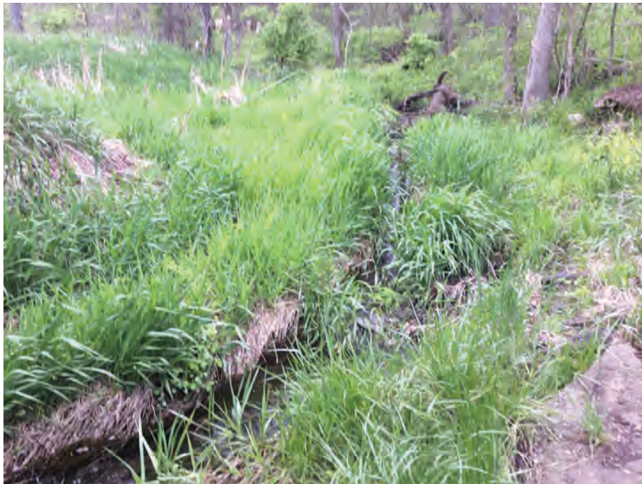
PHOTO 14 Condition Description Up stream alignment or looking north
