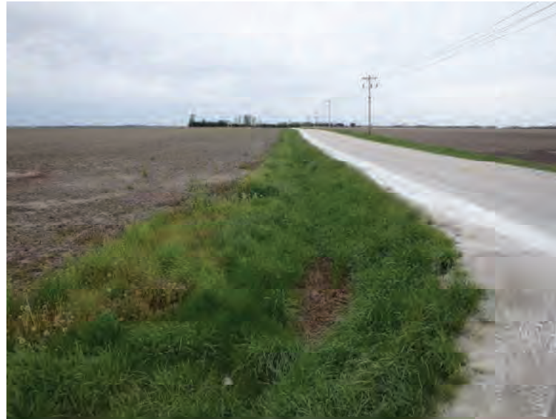
Picture 760: looking west along a roadside ditch on the south side of SR 26, adjacent to N 875 E, 05/04/2020 (Exhibit 6AQ)
