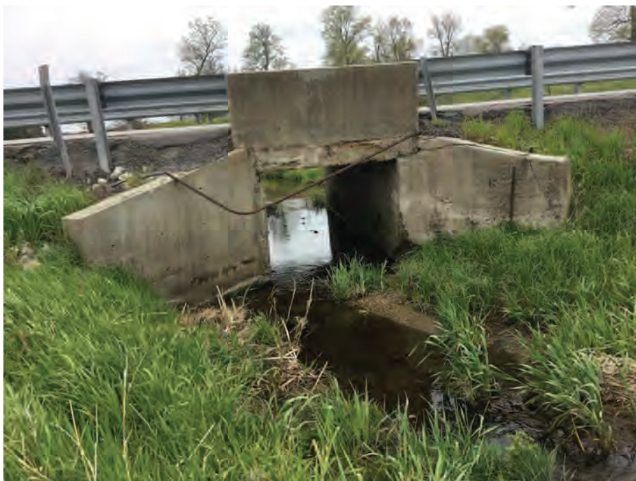
PHOTO 5 Elevation, Condition Description Profile looking south
