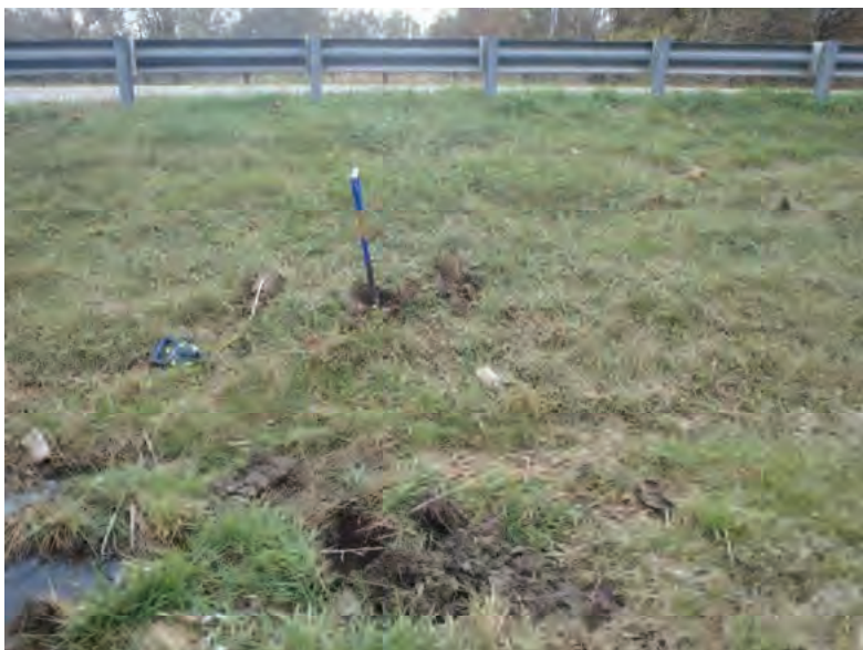
Picture 539: Looking south at the upland conditions surrounding DP 81, on the north side of SR 26, adjacent to E Akers Rd, 11/05/2019 (Exhibit 6AB)
