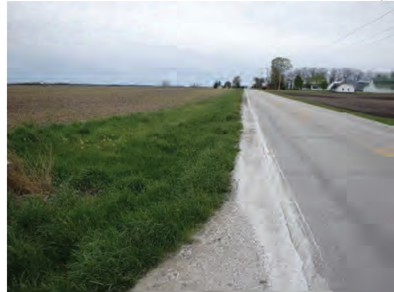
Picture 708: Looking west along a roadside ditch on the south side of SR 26, adjacent to N 725 E, 05/04/2020 (Exhibit 6AM)
