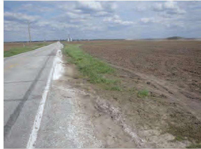
Picture 832: looking east along a roadside ditch on the south side of SR 26, east of Holder Ditch and west of N 1100 E, 05/07/2020 (Exhibit 6AV)
