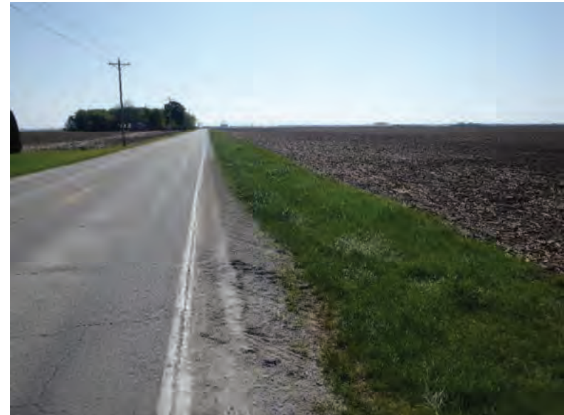
Picture 802: looking east along a roadside ditch on the south side of SR 26, east of Holder Ditch and west of N 1100 E, 05/07/2020 (Exhibit 6AT)
