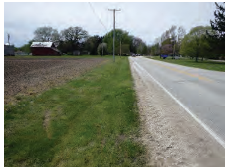
Picture 572: Looking west along a roadside ditch on the south side of SR 26, adjacent to Pine Village Elementary School, 05/04/2020 (Exhibit 6AD)
