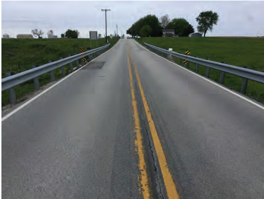
PHOTO 1 Condition Description Road alignment looking west
