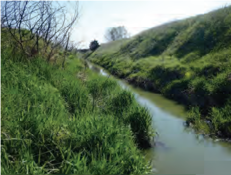
Picture 799: looking northeast, upstream along Holder Ditch on the north side of SR 26, 05/07/2020 (Exhibit 6AT)
