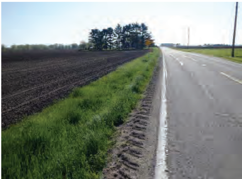
Picture 775: looking east along a roadside ditch on the north side of SR 26, east of N 875 E and west of Holder Ditch, 05/07/2020 (Exhibit 6AR)
