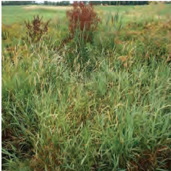
Picture 284: Looking north at the grassed waterway that precedes UNT1 to Big Pine Creek, from the top of structure CV 026 86 12.45 on the north side of SR 26, 07/16/2019 (Exhibit 6Q)
