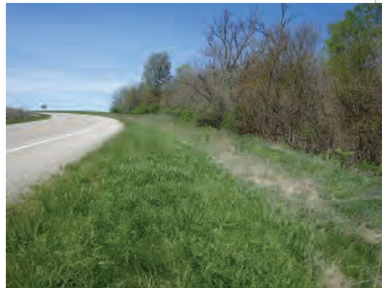
Picture 42: Looking west, west of Mud Pine Creek, along a roadside ditch on the north side of SR 26, 05/01/2020 (Exhibit 6C)
