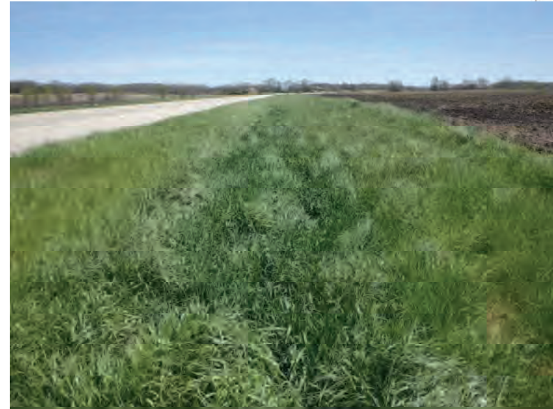
Picture 132: Looking northeast along a roadside ditch on the south side of SR 26, 05/01/2020 (Exhibit 6H)
