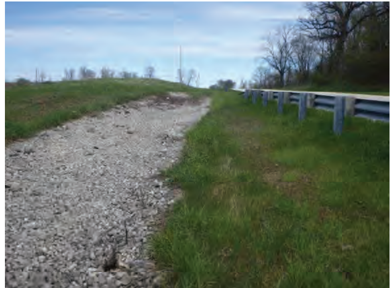
Picture 211: Looking east, east of UNT5 to Mud Pine Creek, along a riprapped roadside ditch on the north side of SR 26, 05/01/2020 (Exhibit 6K)
