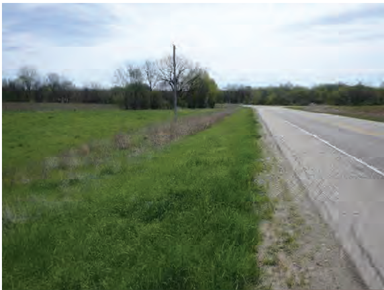
Picture 461: Looking southeast along a roadside ditch on the north side of SR 26, southeast of Wetland 21 and northwest of E Blvd 05/04/2020 (Exhibit 6Y)
