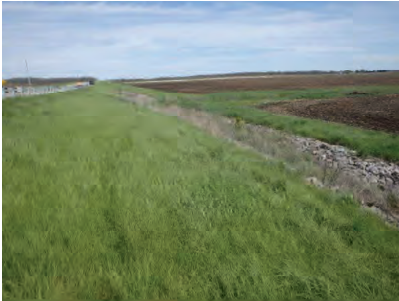
Picture 350: Looking east along a riprapped side ditch leading to UNT4 to Big Pine Creek, on the south side of SR 26, west of UNT 4 to Big Pine Creek, 05/01/2020 (Exhibit 6S)
