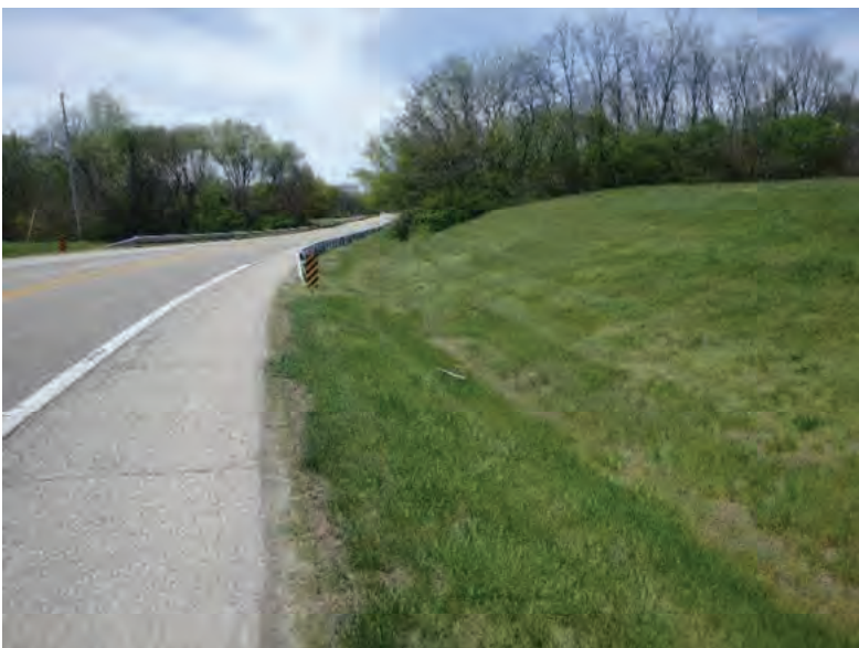
Picture 495: Looking west towards UNT6 to Big Pine Creek along a roadside ditch on the north side of SR 26, 05/04/2020 (Exhibit 6AA)
