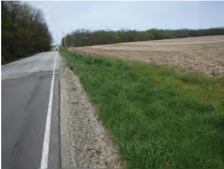
Picture 421: Looking west along a roadside ditch on the north side of SR 26, east of UNT5 to Big Pine Creek, 05/04/2020 (Exhibit 6W)
