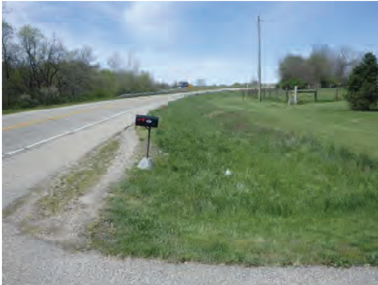
Picture 473: Looking west along a roadside ditch on the north side of SR 26, east of E Blvd and west of UNT6 to Big Pine Creek, 05/04/2020 (Exhibit 6Z)
