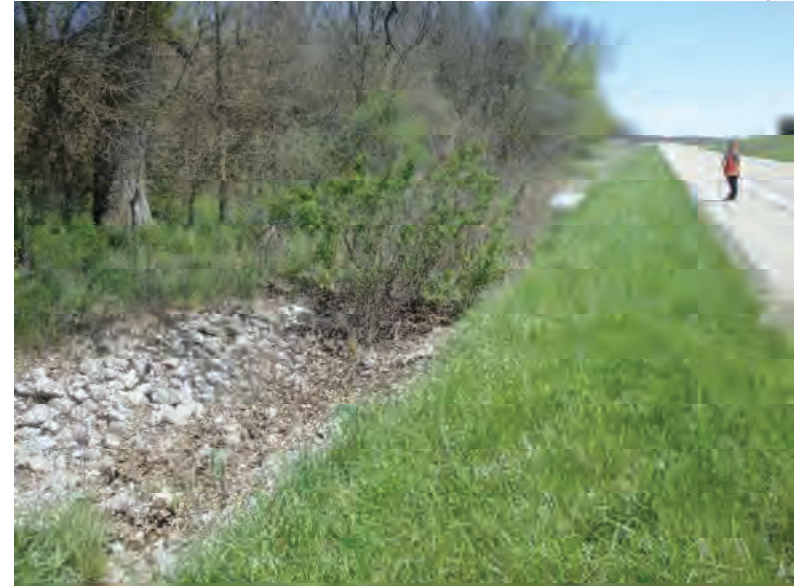
Picture 90: Looking east along a riprapped roadside ditch, on the north side of SR 26 and west of UNT3 to Mud Pine Creek, 05/01/2020 (Exhibit 6F)
