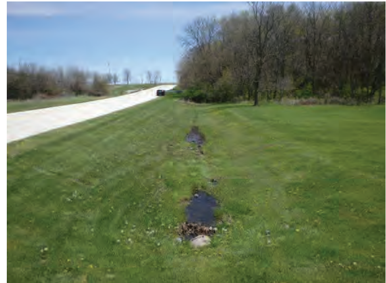
Picture 180: Looking east, towards UNT5 to Mud Pine Creek, along a roadside ditch on the south side of SR 26 05/01/2020 (Exhibit 6K)
