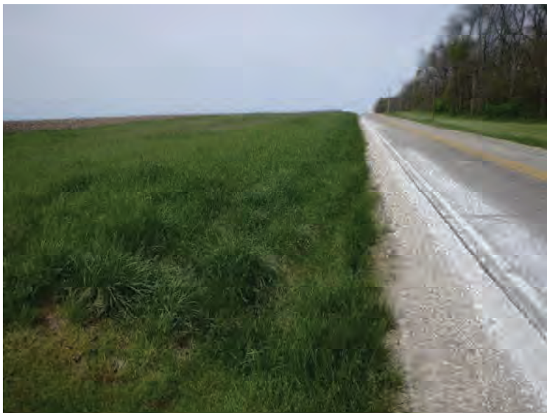
Picture 398: Looking west long the south side of SR 26, adjacent to the intersection of N 200 E, 05/04/2020 (Exhibit 6V)
