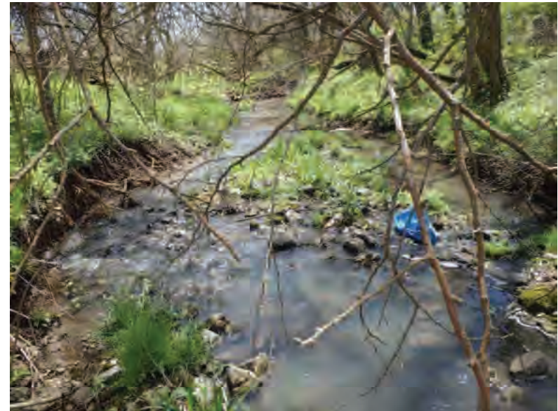
Picture 168: Looking south, downstream, along UNT4 to Mud Pine Creek, on the south side of SR 26, from the top of the structure, 05/01/2020 (Exhibit 6J)
