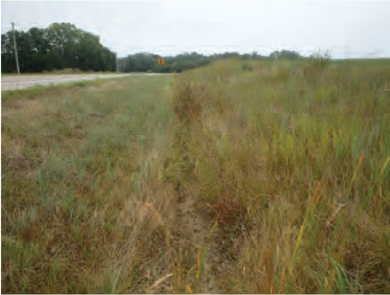
Picture 457: Looking southeast along a roadside ditch on the south side of SR 26, southeast of Wetland 21 and northwest of E Blvd, 08/19/2019 (Exhibit 6Y)
