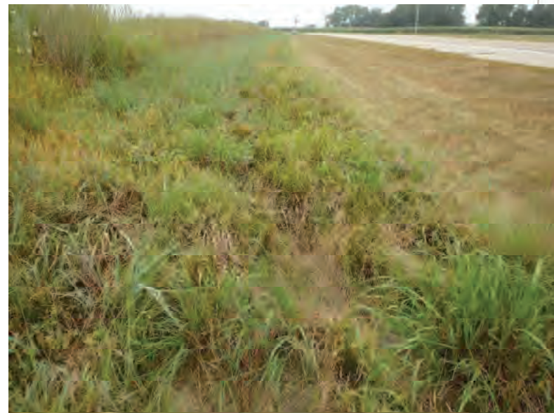
Picture 462: Looking northwest along a roadside ditch on the south side of SR 26, adjacent to the intersection of SR 26 and E Blvd, 08/19/2019 (Exhibit 6Z)
