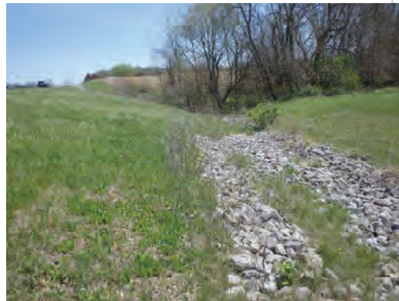
Picture 162: Looking east along a roadside ditch on the south side of SR 26, towards UNT4 to Mud Pine Creek, 05/01/2020 (Exhibit 6J)
