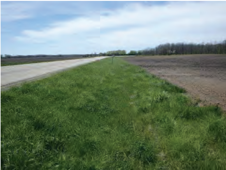
Picture 133: Looking southwest along a roadside ditch on the north side of SR 26, 05/01/2020 (Exhibit 6H)
