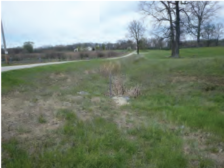
Picture 218: Looking north along a roadside ditch on the north side of SR 26, east of the Meridan Line Rd intersection, 05/01/2020 (Exhibit 6L)
