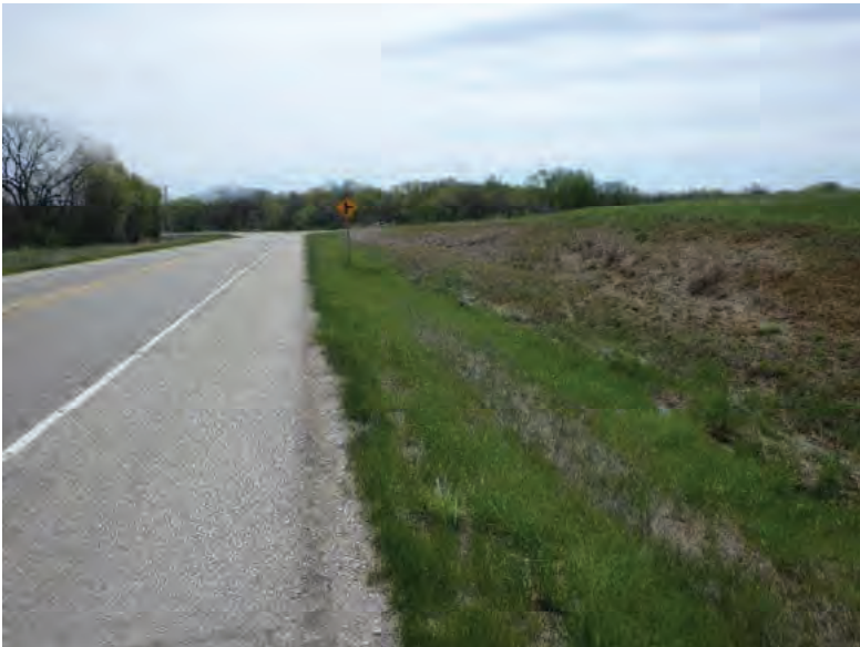
Picture 459: Looking southeast along a roadside ditch on the south side of SR 26, southeast of Wetland 21 and northwest of E Blvd, 05/04/2020 (Exhibit 6Y)
