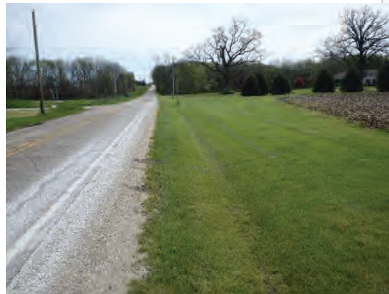
Picture 399: Looking east along a roadside ditch on the south side of SR 26, adjacent to the intersection of N 200 E, 05/04/2020 (Exhibit 6V)
