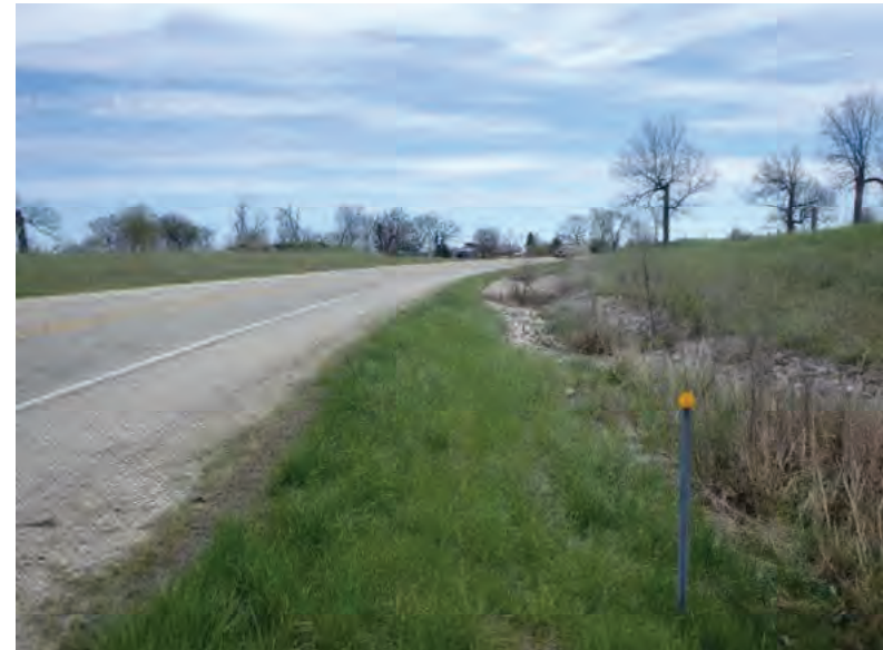
Picture 219: Looking east along a riprapped roadside ditch on the south side of SR 26, east of the Meridan Line Rd intersection, 05/01/2020 (Exhibit 6L)
