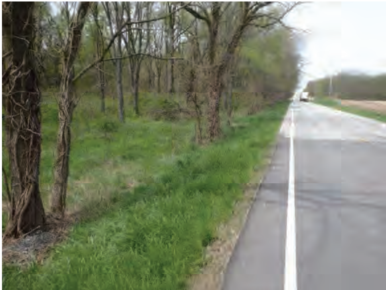
Picture 419: Looking west along the south side of SR 26, including the forested area east of UNT5 to Big Pine Creek, 05/04/2020 (Exhibit 6W)
