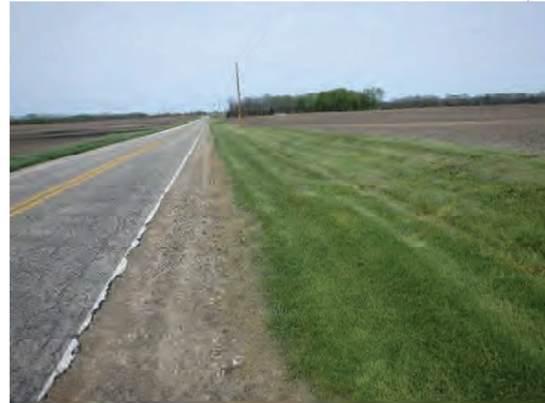
Picture 371: Looking west along roadside ditch on the north side of SR 26, 05/04/2020 (Exhibit 6T)
