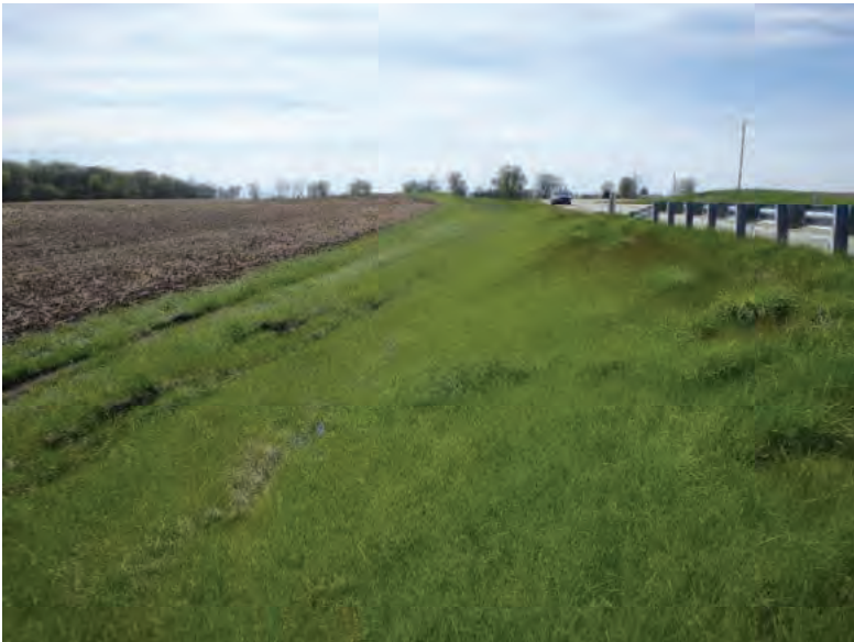
Picture 280: Looking west along roadside ditch on the south side of SR 26, west of UNT1 to Big Pine Creek, 05/01/2020 (Exhibit 6P)
