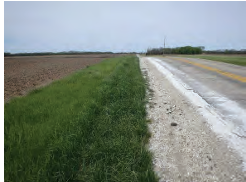
Picture 373: Looking west along roadside ditch on the south side of SR 26, 05/04/2020 (Exhibit 6T)
