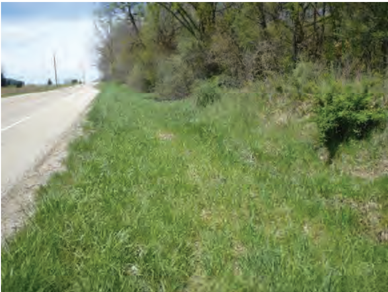
Picture 91: Looking west along a roadside ditch on the north side of SR 26, west of UNT3 to Mud Pine Creek, 05/01/2020 (Exhibit 6F)
