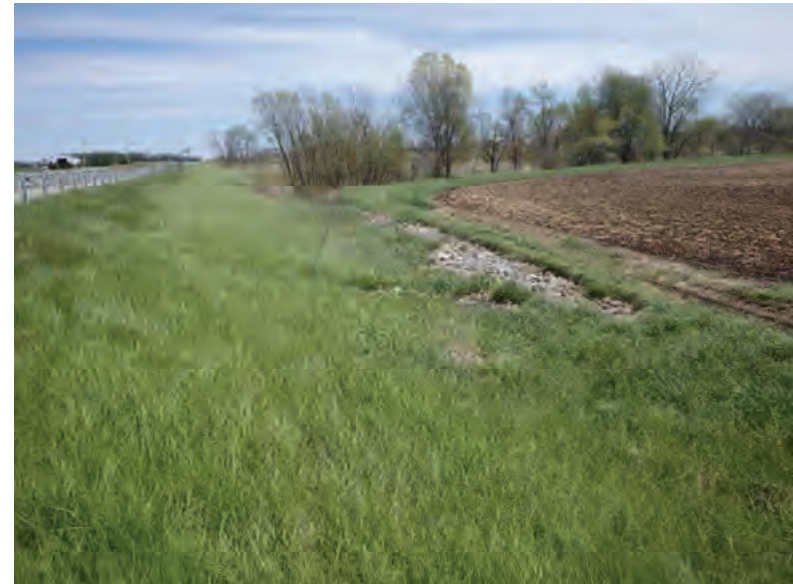
Picture 281: Looking east along roadside ditch on the south side of SR 26, west of UNT1 to Big Pine Creek 05/01/2020 (Exhibit 6P)
