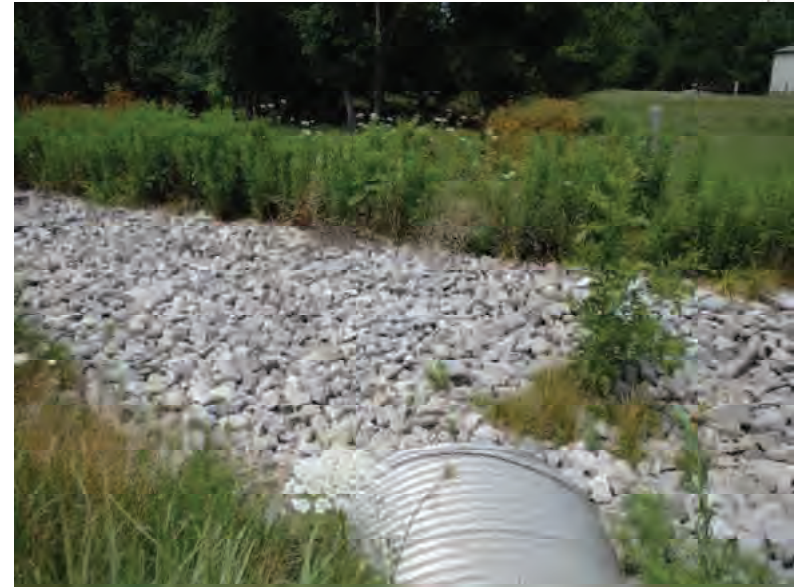
Picture 470: Looking north at a riprapped roadside ditch from the top of structure CV 026 86 15.00 on the north side of SR 26, 07/16/2019 (Exhibit 6Z)
