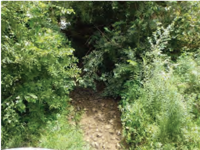
Picture 491: Looking south, downstream, at UNT6 to Big Pine Creek from the top of the south side of the structure on the south side of SR 26, 07/16/2019 (Exhibit 6AA)
