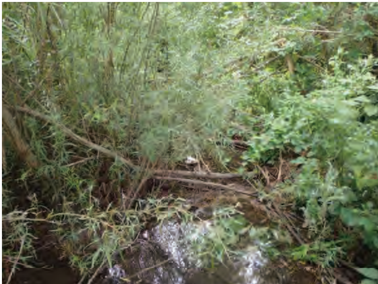
Picture 288: Looking south, downstream, at UNT1 to Big Pine Creek from the top of structure CV 026 86 12.45, on the south side of SR 26, 07/16/2019 (Exhibit 6Q)
