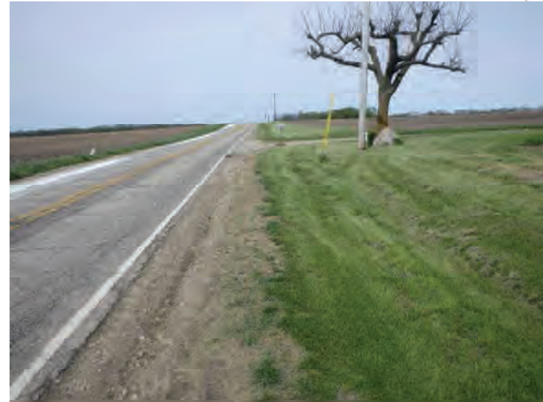
Picture 379: Looking west along roadside ditch on the north side of SR 26, west of N 175 E, 05/04/2020 (Exhibit 6U)
