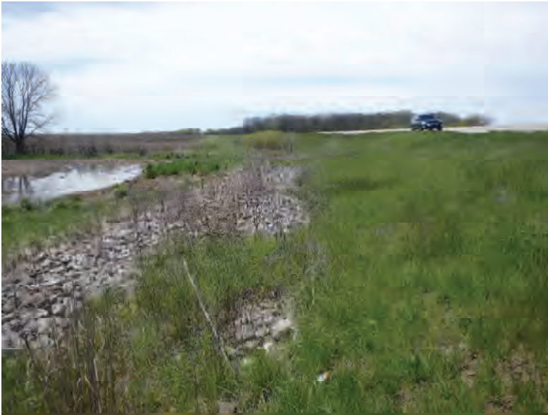
Picture 157: Looking southwest, towards Wetland 11, at a roadside ditch on the south side of SR 26, 05/01/2020 (Exhibit 6I)
