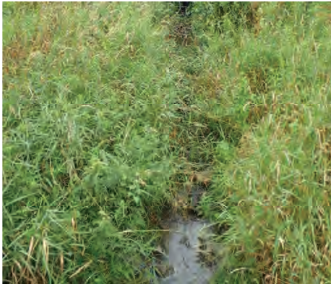
Picture 206: Looking north, upstream, along UNT5 to Mud Pine Creek from the top of the structure, on the north side of SR 26, 07/16/2019 (Exhibit 6K)
