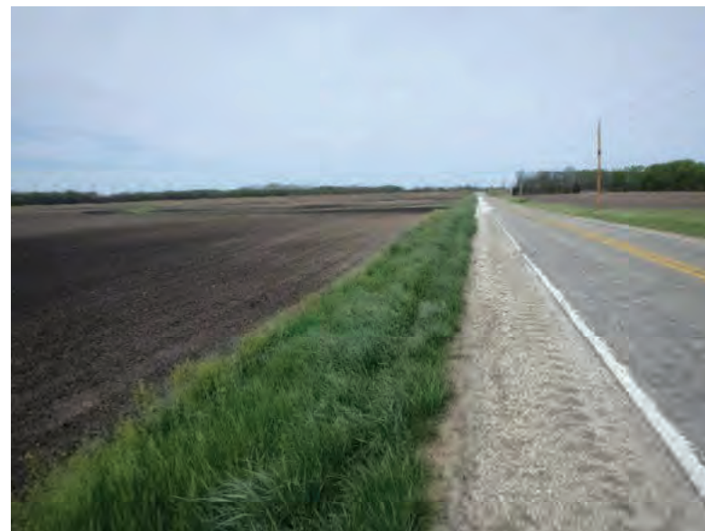
Picture 369: Looking west along roadside ditch on the south side of SR 26, 05/04/2020 (Exhibit 6T)
