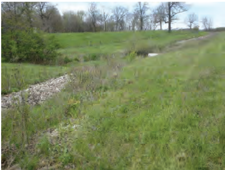
Picture 231: Looking northwest, towards UNT6 to Mud Pine Creek, along a riprapped roadside ditch on the west side of SR 26, 05/01/2020 (Exhibit 6M)
