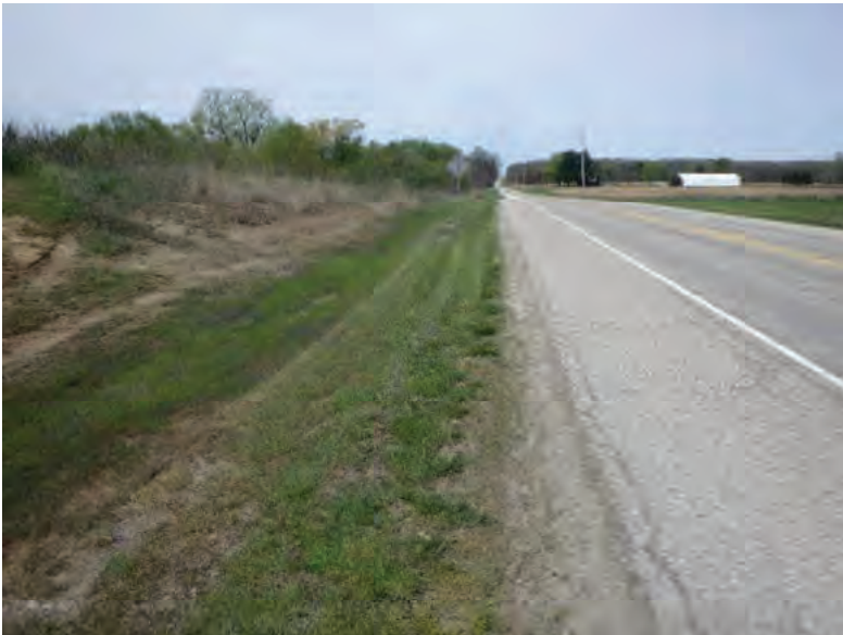
Picture 439: Looking west along a roadside ditch on the south side of SR 26, east of Channel 4 and west of Wetland 20, 05/04/2020 (Exhibit 6X)
