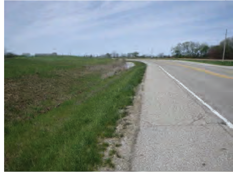
Picture 458: Looking northwest along a roadside ditch on the south side of SR 26, southeast of Wetland 21 and northwest of E Blvd, 05/04/2020 (Exhibit 6Y)
