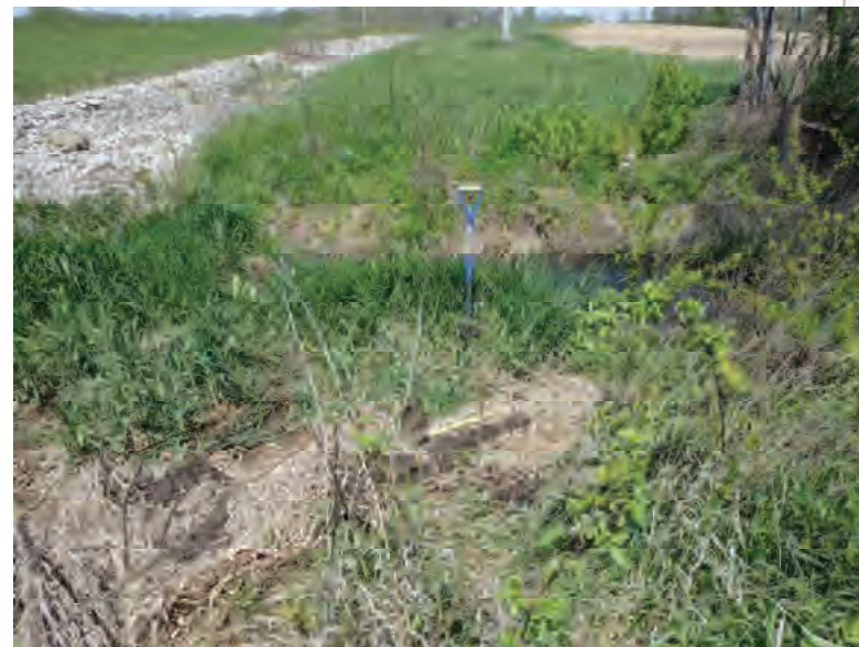
Picture 267: Looking northwest at the upland area surrounding DP90, adjacent to Channel 3, 05/07/2020 (Exhibit 60)
