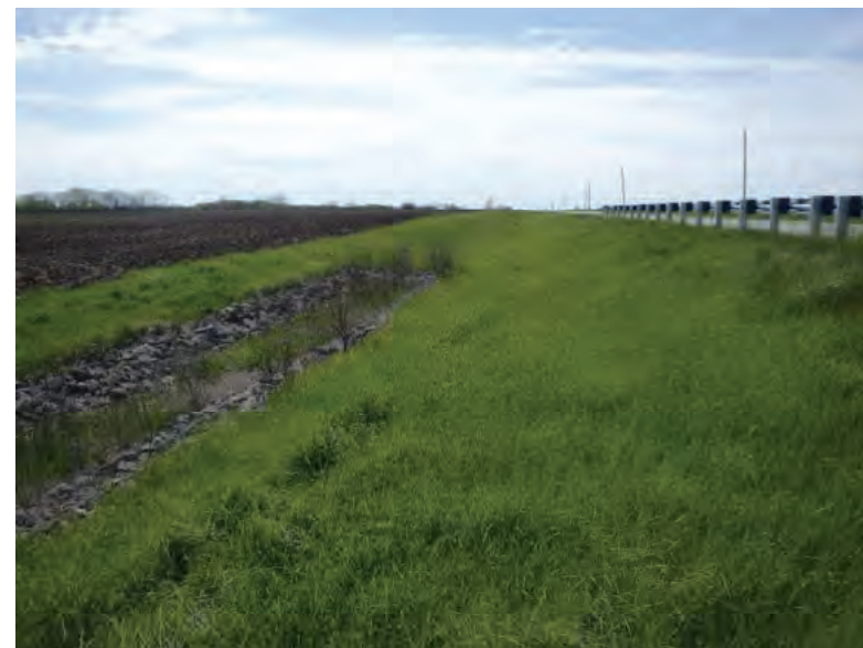
Picture 349: Looking west along a riprapped side ditch on the south side of SR 26, west of UNT 4 to Big Pine Creek, 05/01/2020 (Exhibit 6S)
