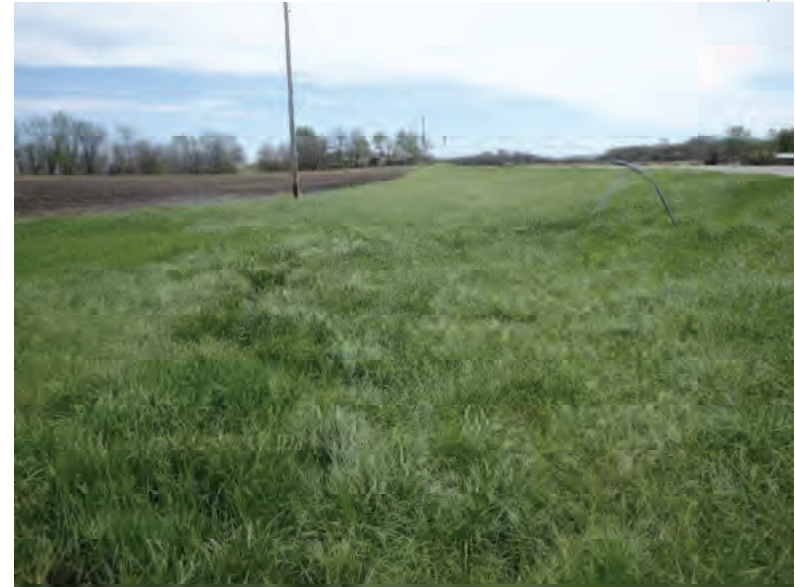
Picture 240: Looking southeast along a roadside ditch on the east side of SR 26, north of the N Rainsville Rd intersection, 05/01/2020 (Exhibit 6N)
