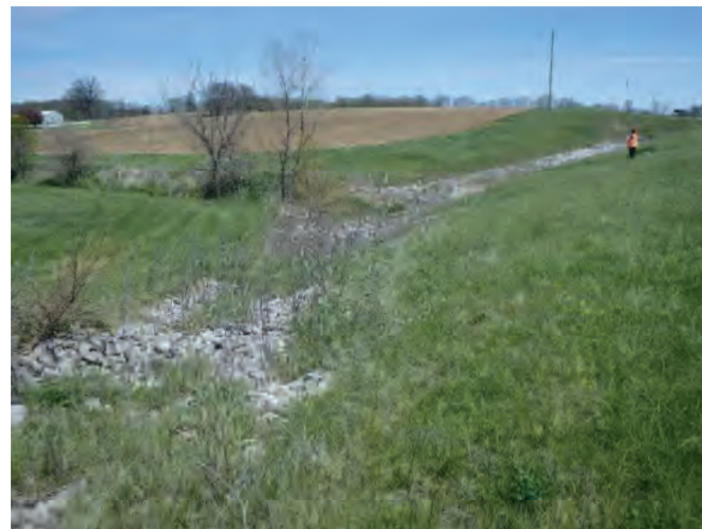
Picture 164: Looking east along a roadside ditch on the north side of SR 26, towards UNT4 to Mud Pine Creek 05/01/2020 (Exhibit 6J)
