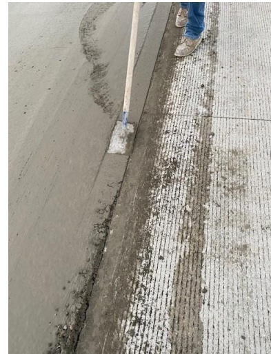
Figure 6-11 Hand Finishing Pavement Edge
