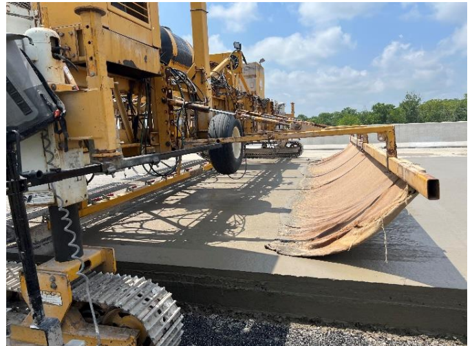
Figure 4-7 Tining Equipment
