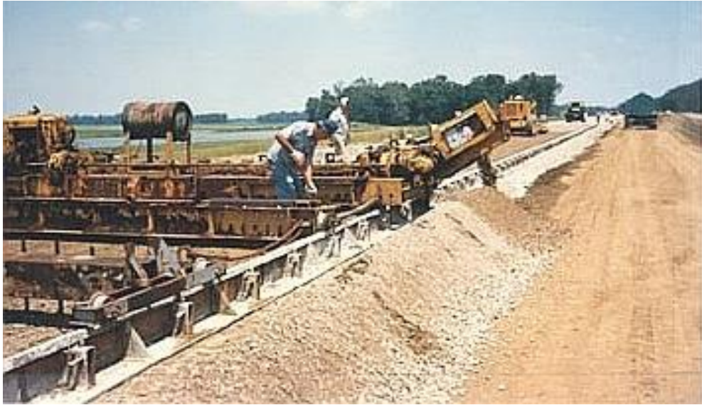
Figure 2-1 Form Paving Spreader
