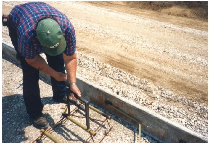
Figure 6-3 Dowel Bar Checker
