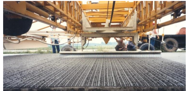
Figure 6-10 Machine Transverse Tining
