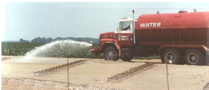
Figure 6-1 Subbase Watering
