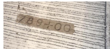
Figure 6-13 Pavement Stationing
