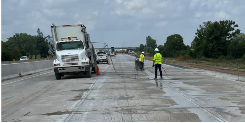
Figure 4-11 Sawing joints into concrete
