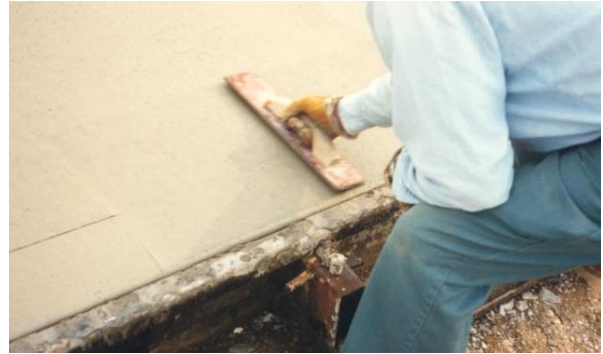
Figure 6-7 Hand Finishing
