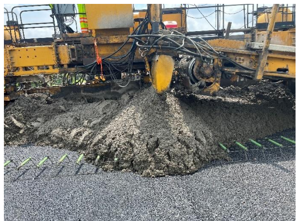
Figure 4-6 Slip-Form Paver
