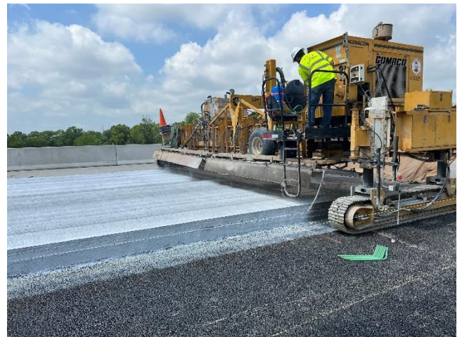
Figure 6-15 Liquid Membrane Application
