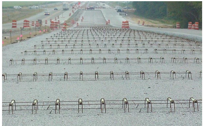
Figure 7-2 Dowel Bar Assemblies
