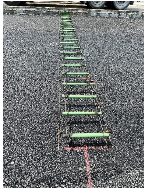
Figure 6-2 Dowel Bar Assembly
