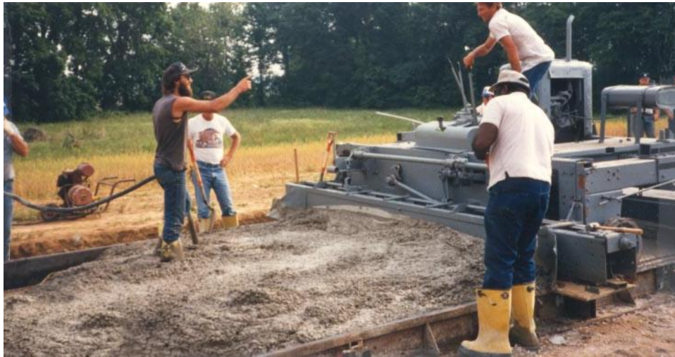
Figure 5-1 Form Paving
