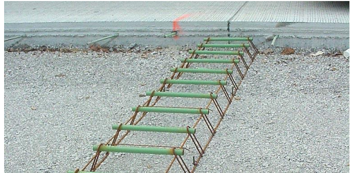
Figure 7-3 Tie Bar Adjustment at Dowel Bar Assembly
