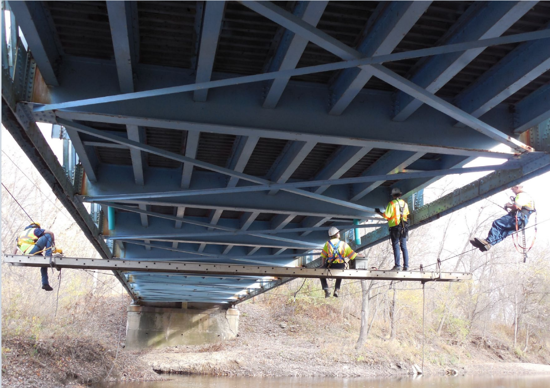
Replace 5 of 8 Substandard Stringers
