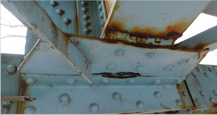
Replace Lower Gusset Plates
