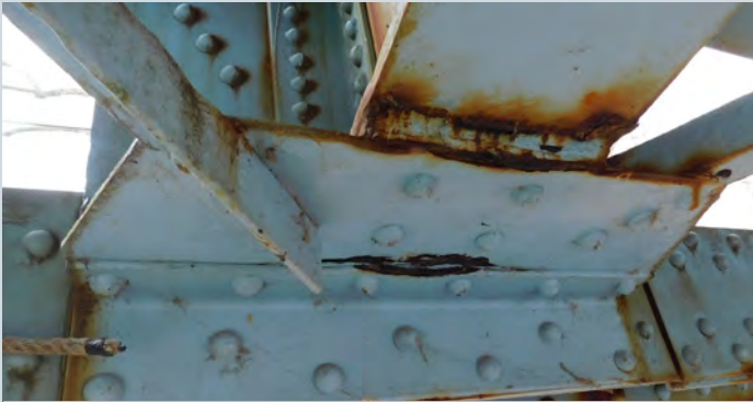
Replace Lower Gusset Plates
