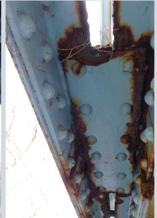
Replace Lower Chord Members
