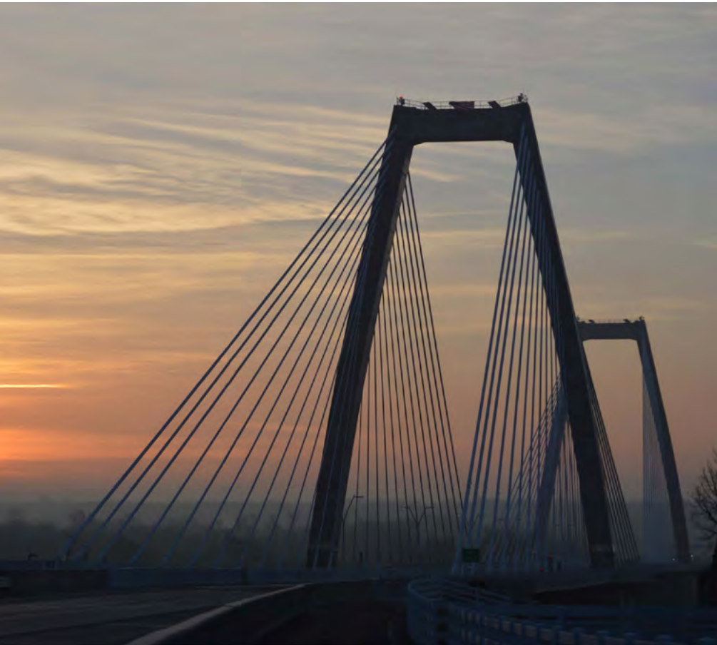
Lewis & Clark Bridge over the Ohio River, on Indiana 265 near Utica
