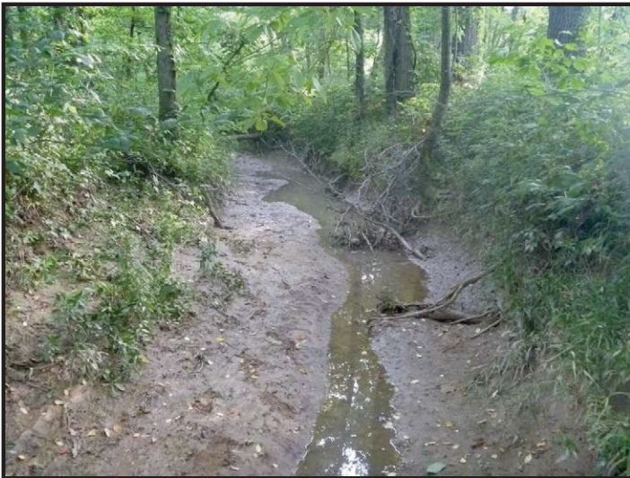
Photo 3 – UNT to Splunge Creek, Upstream from SR 159: Facing upstream to the southwest along UNT to Splunge Creek, upstream of the inlet. The OHWM in this area measured 14 ft. wide by 30 in. deep.
