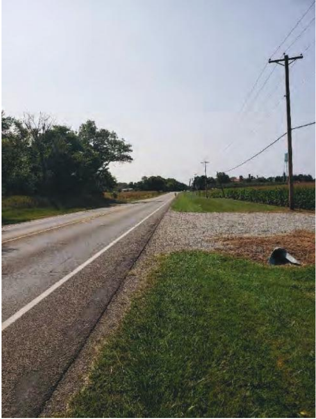
15. Facing south on the north end of the APE on SR 9
