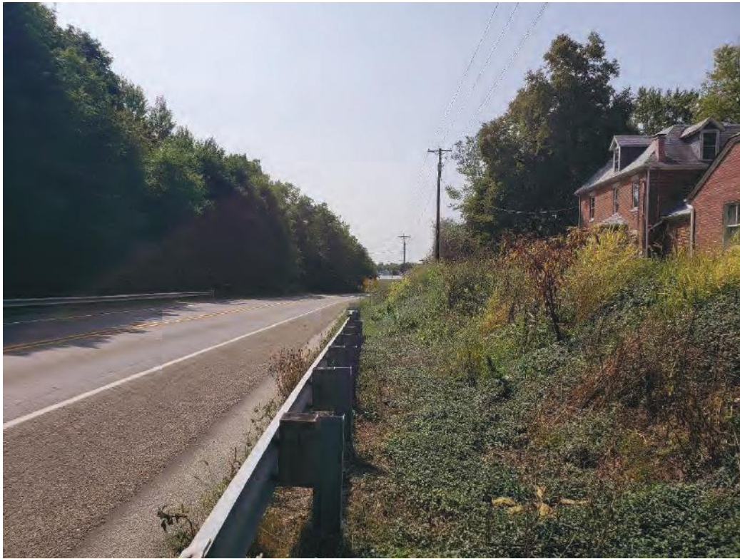
5. Facing south on SR 9 from south-facing side of Bridge No. 009-57-02086C
