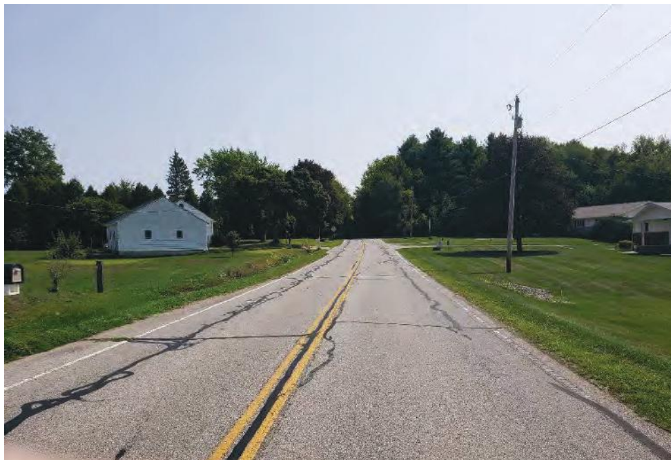
4. Facing east on Northport Rd. at east end of APE
