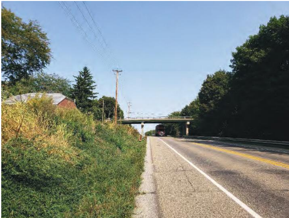
6. Facing north on SR 9 toward Bridge No. 009-57-02086C
