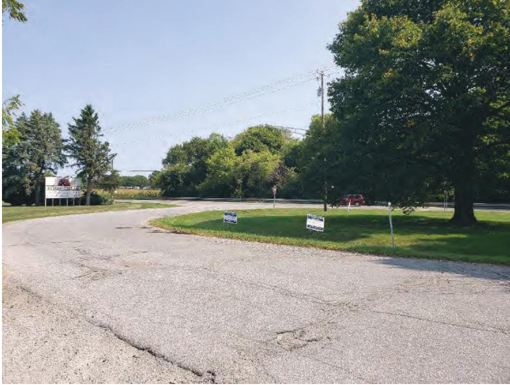
11. Facing northeast on Kelly Rd. toward SR 9
