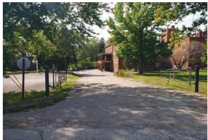
(LEFT) Facing driveway entrance toward wrought iron gates to Kneipp Springs Historic District from SR 9 south of the bridge; work proposed includes the following: driveway approach milling and surfacing with the installation of concrete curb, SR 9 profile grade will be raised approximately two feet; the existing inlet will be replaced in kind and the ditch will be regraded and tied to the existing storm sewer; and existing guardrail will be removed and replaced, extending southward along the edges of SR 9. All work will occur within the existing right-of-way.
