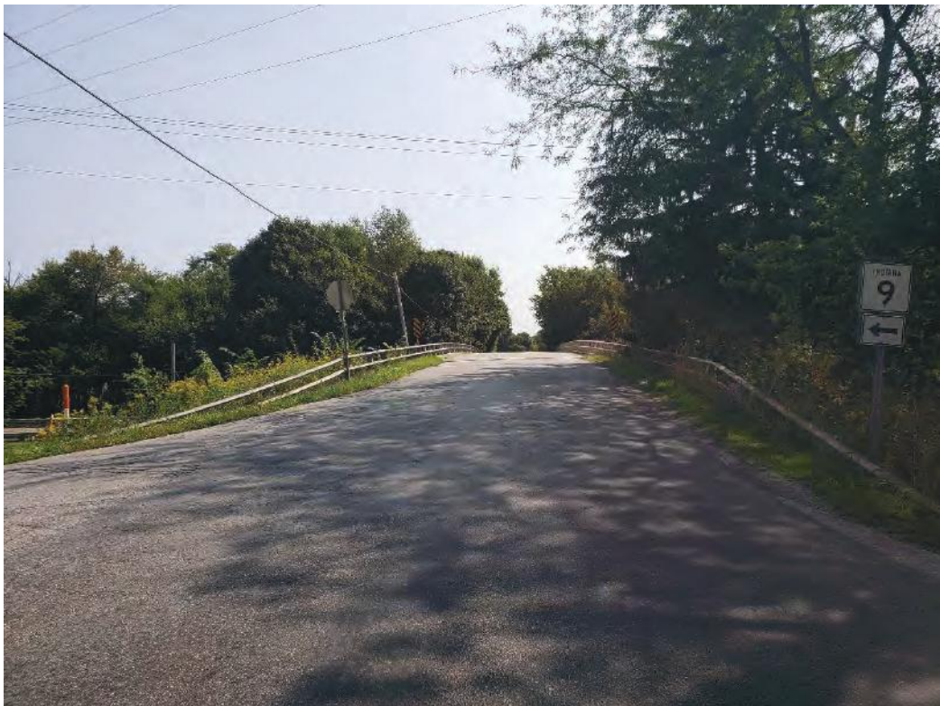
10. Facing east on Northport and Kelly Rd. toward Bridge No. 009-57-02086C
