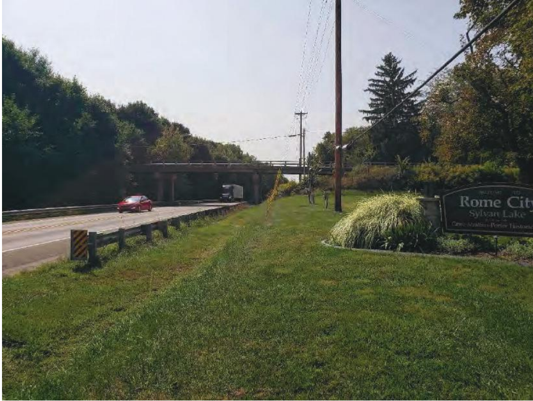
13. Facing south on SR 9 toward north-facing side of Bridge No. 009-57-02086C
