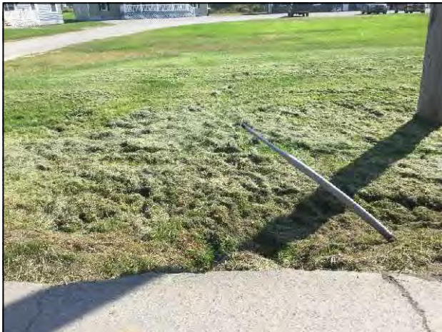
15. View of culvert and SR 5 ROW on the west side of SR 5, looking north within project area.
