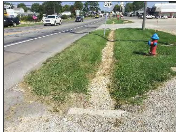
20. View of culvert on the east side of SR 5, looking north within project area.
