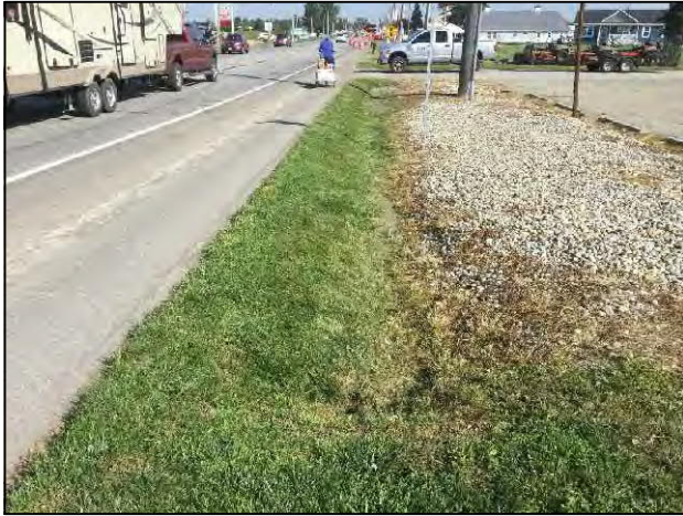
13. View of culvert and SR 5 ROW on the east side of SR 5, looking north within project area.
