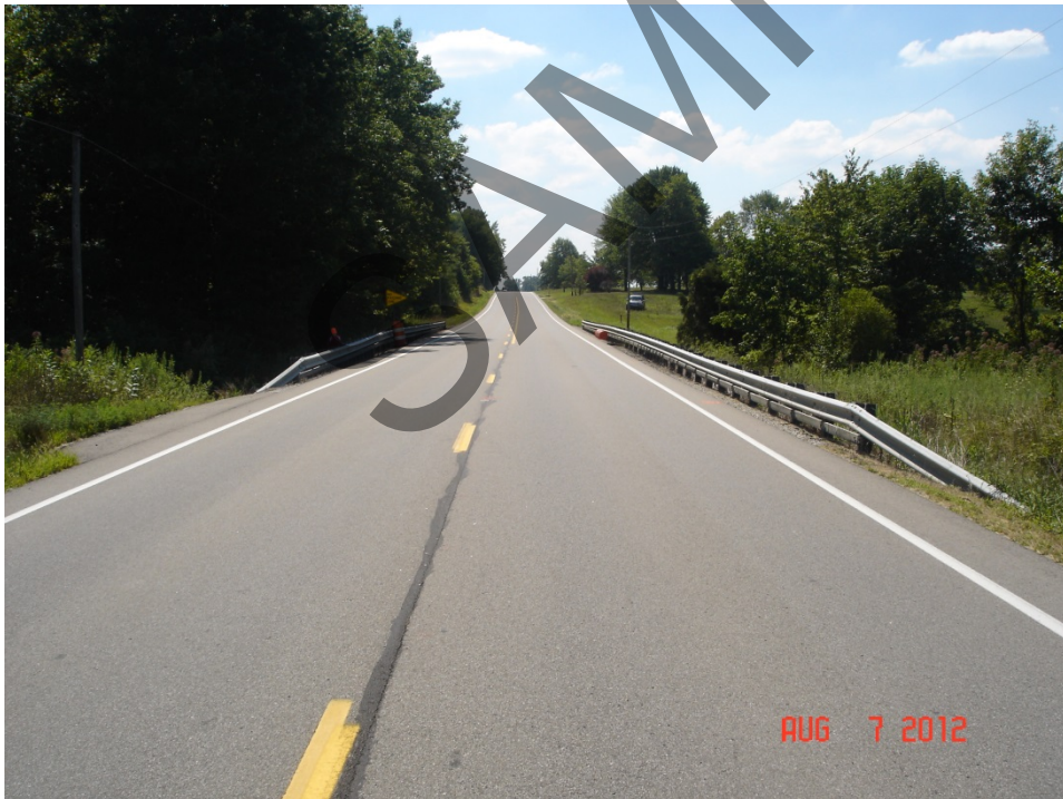
2. Standing north of the structure looking south along SR 7.
