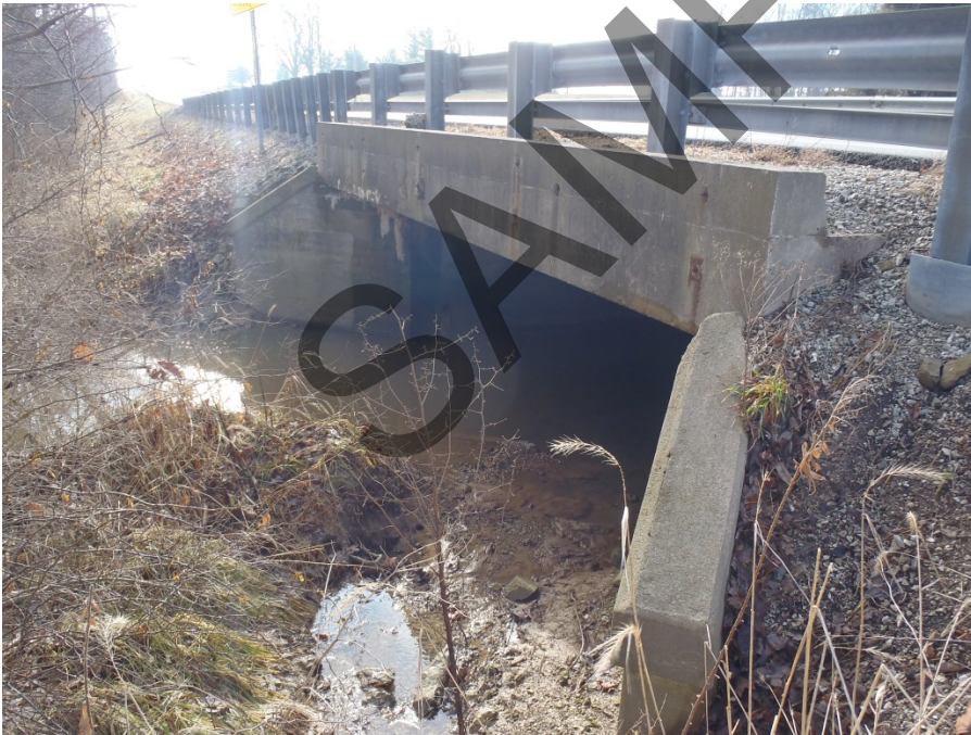
8. Standing east of the structure looking at the downstream northern abutment
