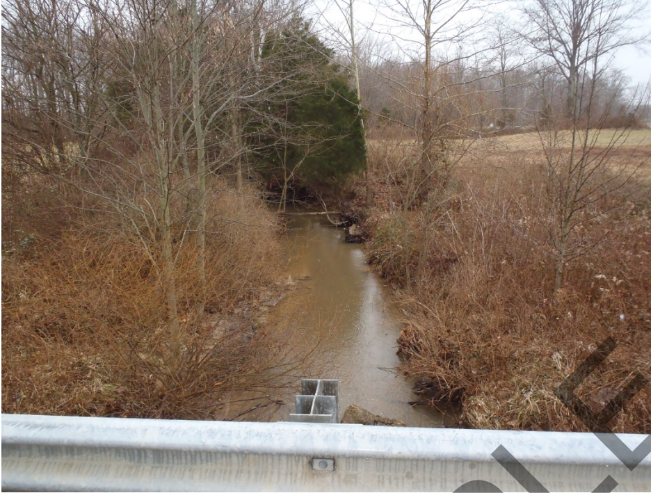
3. Standing at the structure looking west at the creek.
