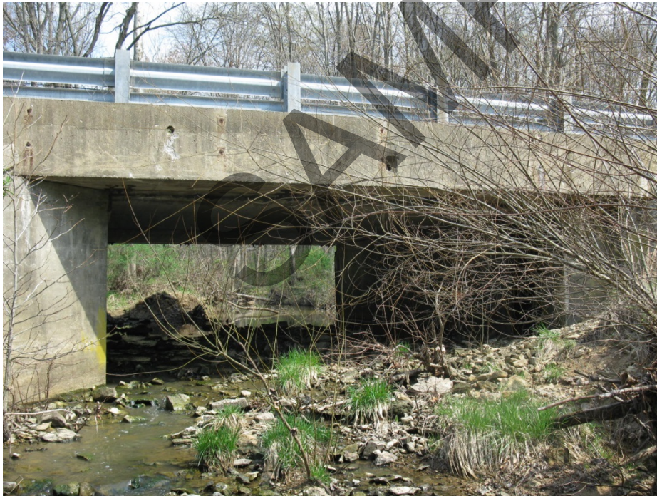
6. Standing upstream of the structure looking east
