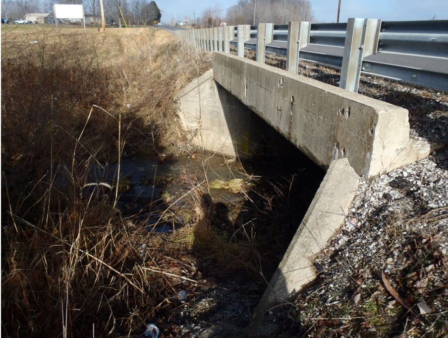
7. Standing west of the structure looking at the upstream southern abutment
