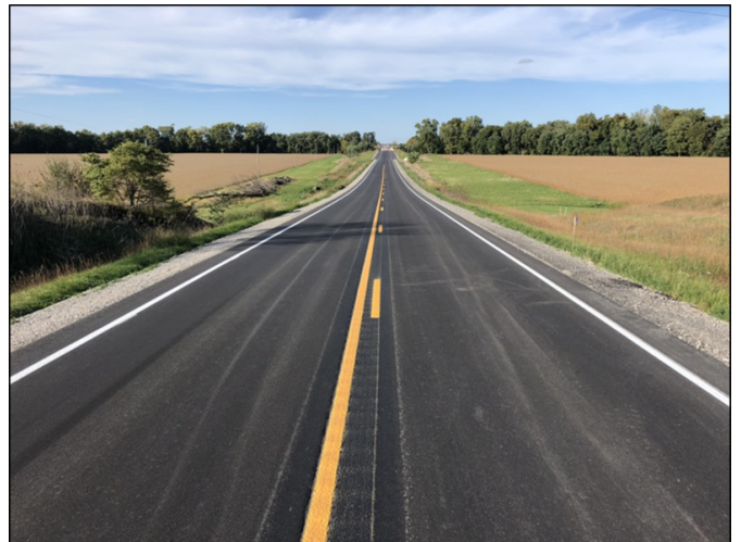
Final Pavement Surface
