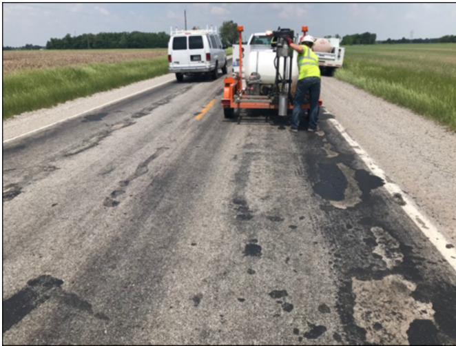
Existing Pavement Surface during Investigative Sampling
