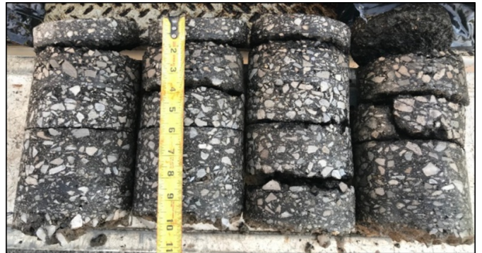
Pavement Samples taken during Investigative Sampling
