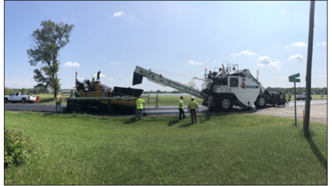
Paving of the 2.0-inch 12.5mm HMA surface
