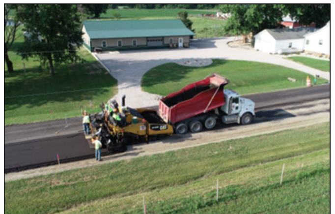
Paving of the 6.0-inch CCPR lift
