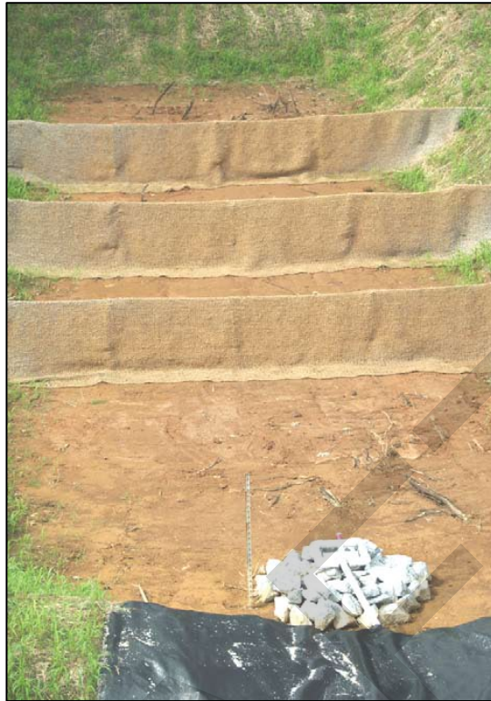
Exhibit 708.06-D. Example of porous baffles made of 700 g/m 2 coir erosion control blanket as viewed from the basin outlet.
