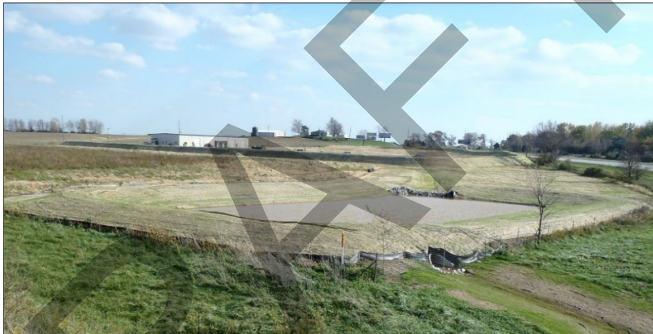
Exhibit 708.02-A. A permanent stormwater basin modified to function as temporary sediment basin during construction.
